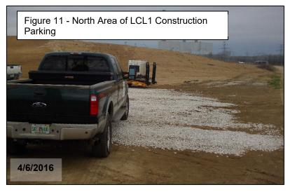
The gravel used for the roadways, under the FCM, and parking lots nearby consists mostly of limestone and dolomite and contains some calcite sourced from nearby quarries. Precipitation and infiltration of surface water through fresh gravel, salting of gravel and road surfaces, and concrete that contains water-soluble salts leach soluble components into the shallow groundwater and can cause an increase in the COIs observed in TMW-2.
