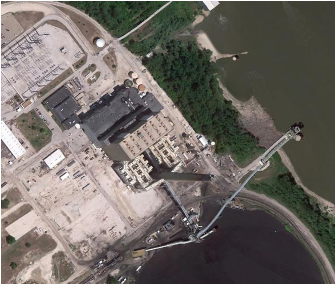
Figure 10: Stacks at Rush Island Plant
