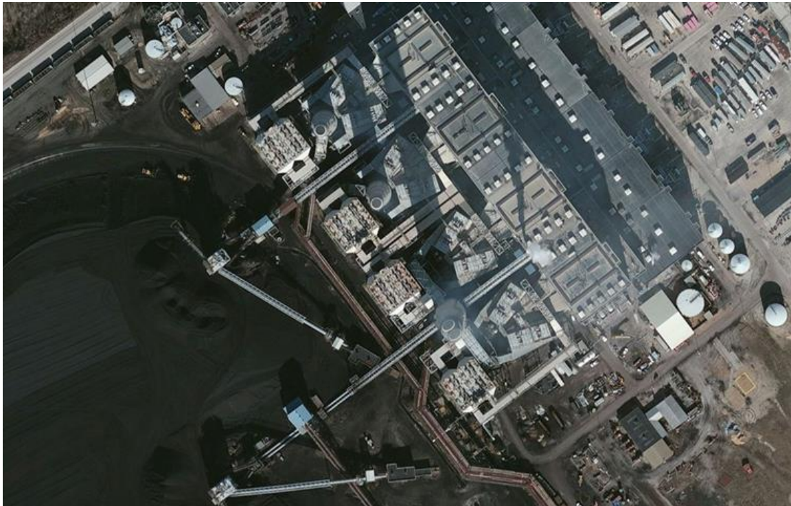
Figure 8: Stacks at Labadie Generating Station
