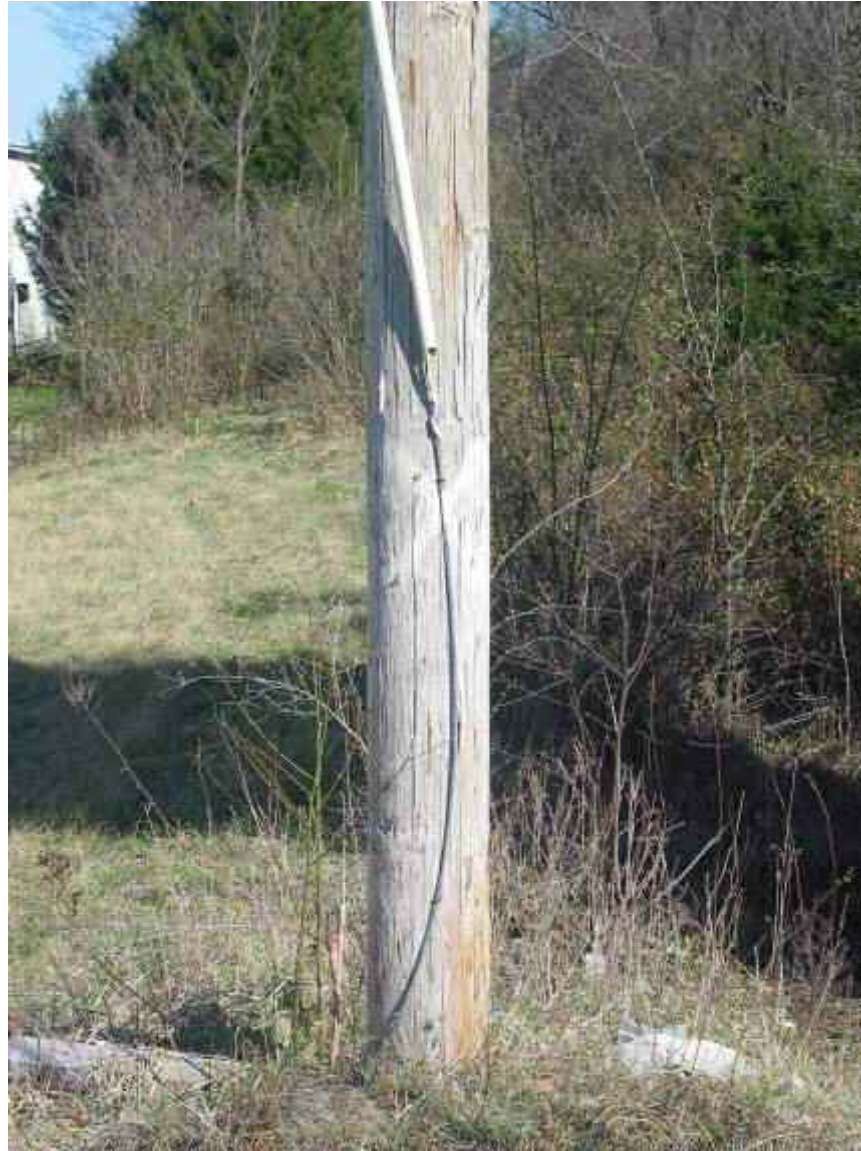
Broken, loose guy wire
