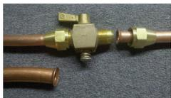
**Flared Gas Fittings** – Over time, corrosion can weaken the flared fittings used to connect copper tubing to house piping and gas appliances. A break can lead to a gas leak, fire or explosion.
