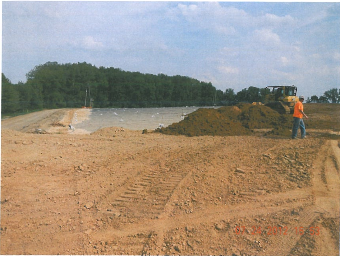
Photograph 9 ▲ - Clay placement facing southeast
