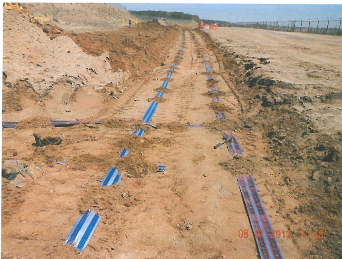
Photograph 15 ▲ - Detectable utility tape in collector trench facing east
