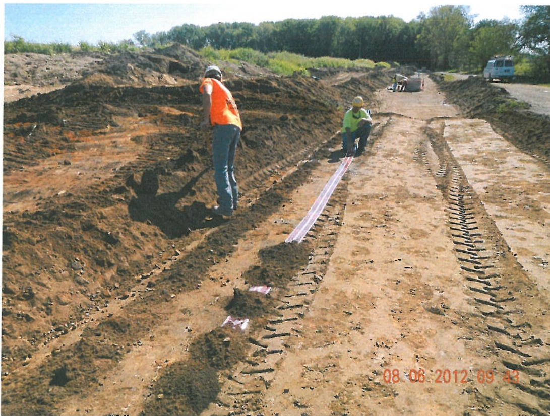
Photograph 2 ▲ - Detectable utility tape in collector trench facing east
