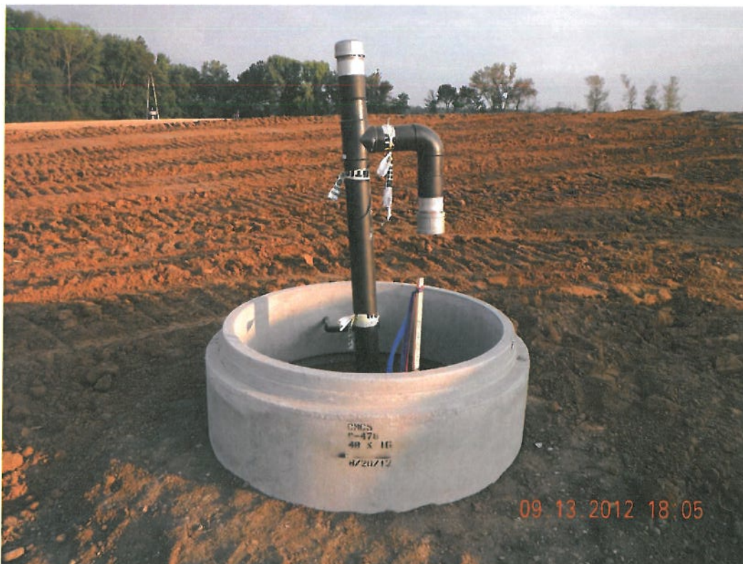
Photograph 4 ▲ - Completed cap vent facing south
