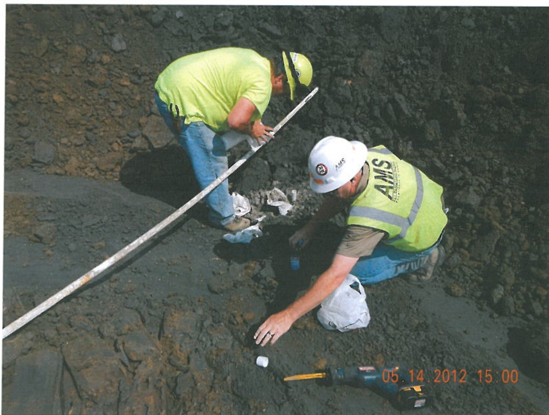
Photograph 6 ▲ - Abandoning monitoring well facing northeast
