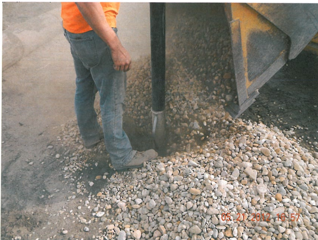
Photograph 4 ▲ - Installing cap vent facing south
