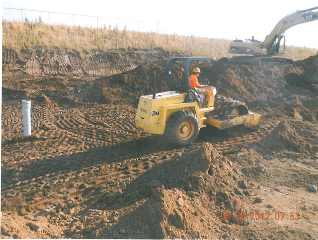
Photograph 9 ▲ - PCP-3 compaction facing north
