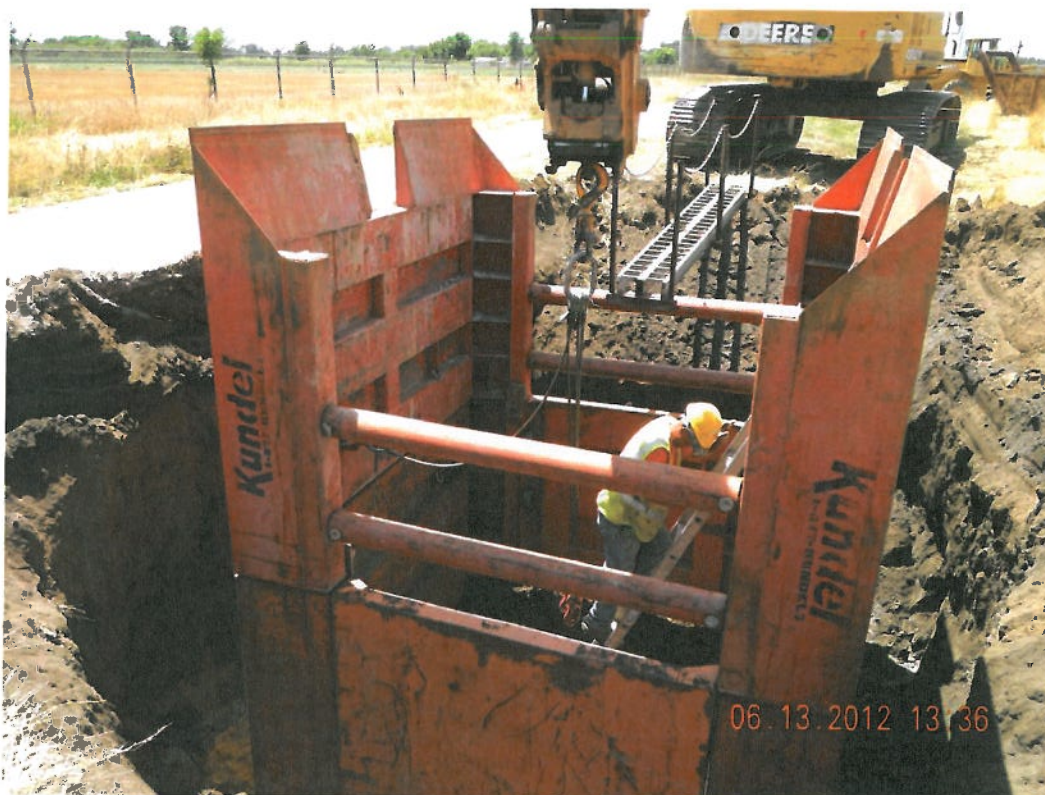
Photograph 6 ▲ - Manhole shoring at DS-1 facing west
