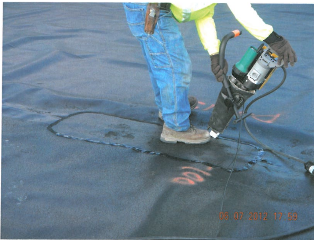
Photograph 8 ▲ - Extrusion welding repairs facing northeast
