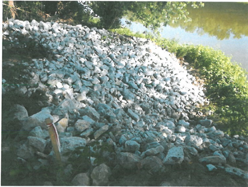
Photograph 1 ▲ - Construction of the outfall swale to the river facing north.
