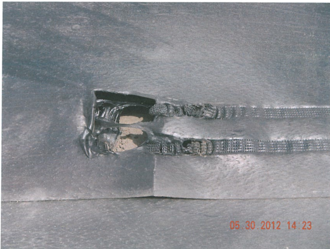
Photograph 4 ▲ - Burn out in seam facing southeast
