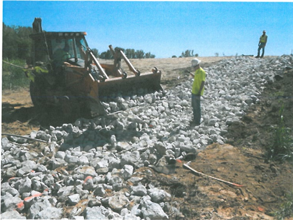
Photograph 7 ▲ - Rock chute construction facing south.
