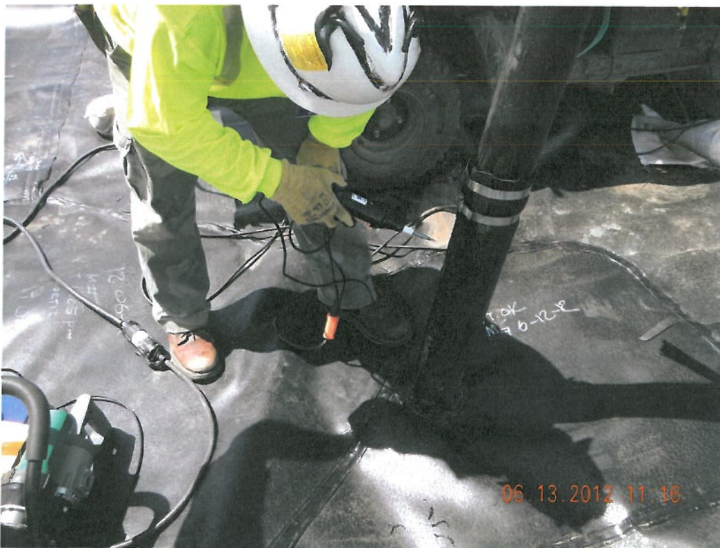
Photograph 4 ▲ - Spark testing cap vent boots facing south
