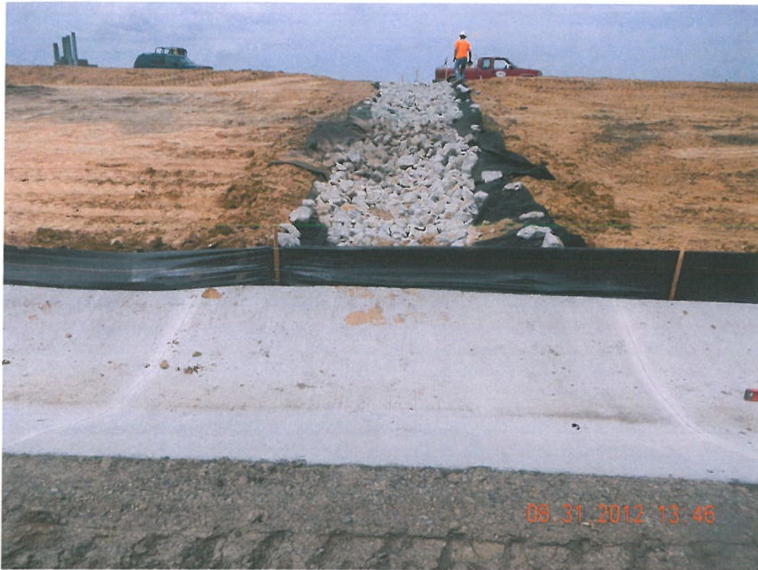
Photograph 9 ▲ - Rock chute construction south of Ash Pond D facing north
