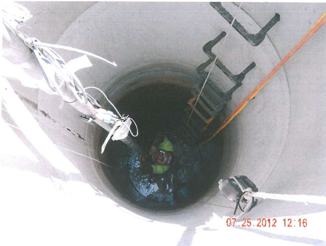
Photograph 10 ▲ - DS-2 sump pump assembly installation facing northeast
