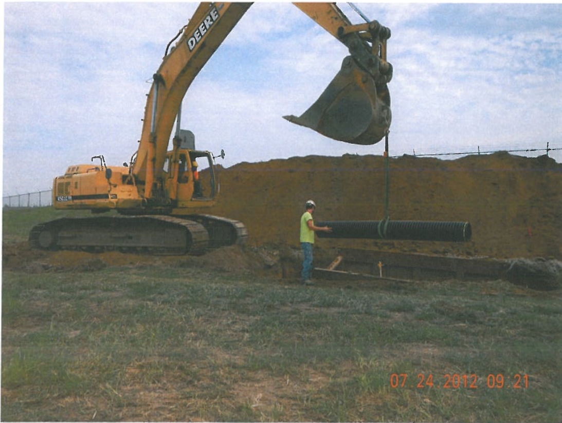
Photograph 5 ▲ - Field tile installation facing northwest
