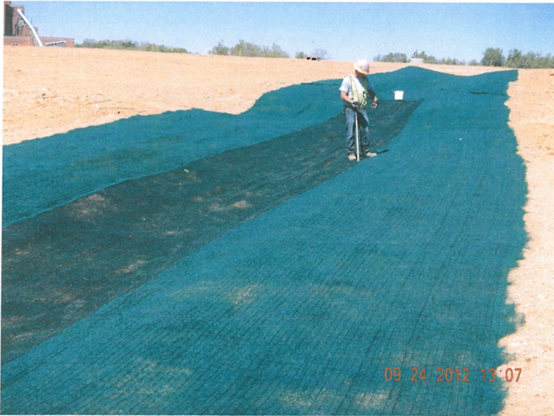
Photograph 5 ▲ - Installing turf reinforcement mat facing north
