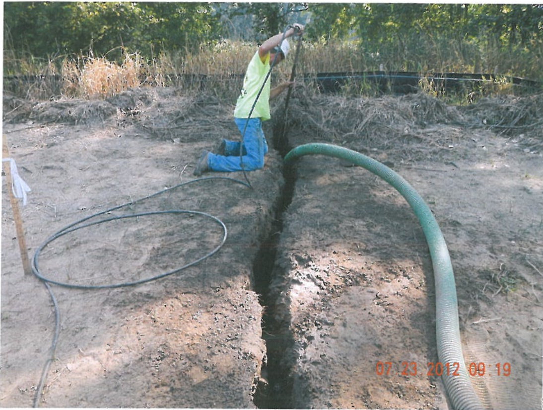
Photograph 3 ▲ - Potholing for deep well utilities facing northeast
