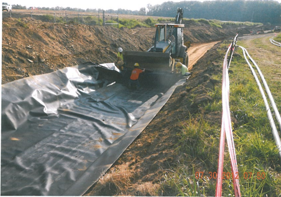
Photograph 3 ▲ - GCL deployment facing northeast
