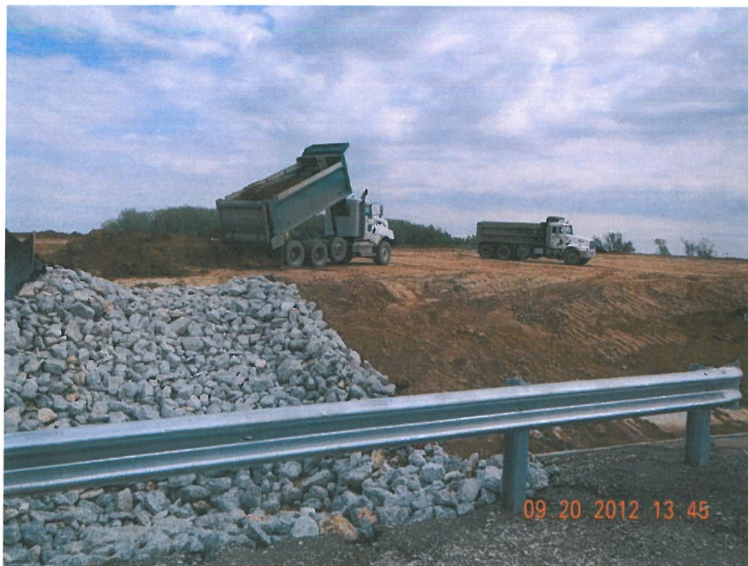
Photograph 8 ▲ - Vegetative layer placement facing east
