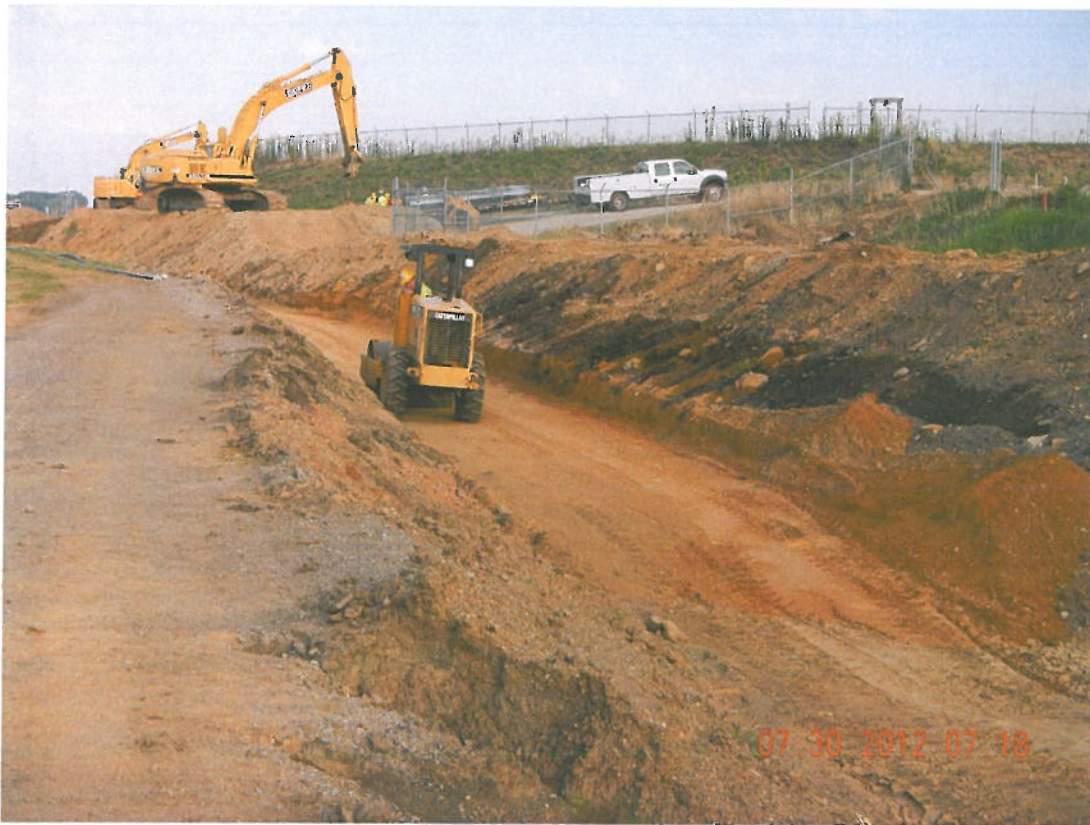
Photograph 1 ▲ - GCL subgrade compaction facing west
