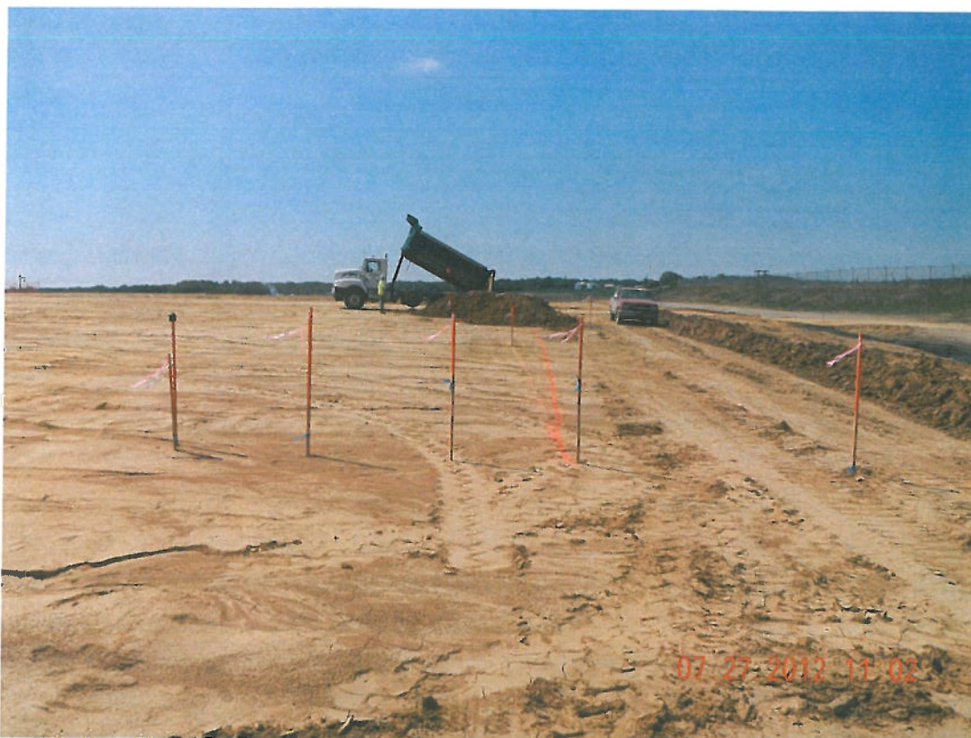
Photograph 12 ▲ - Slope diversion berm construction facing south
