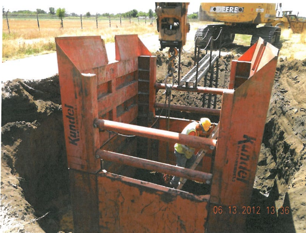
Photograph 6 ▲ - Manhole shoring at DS-1 facing west
