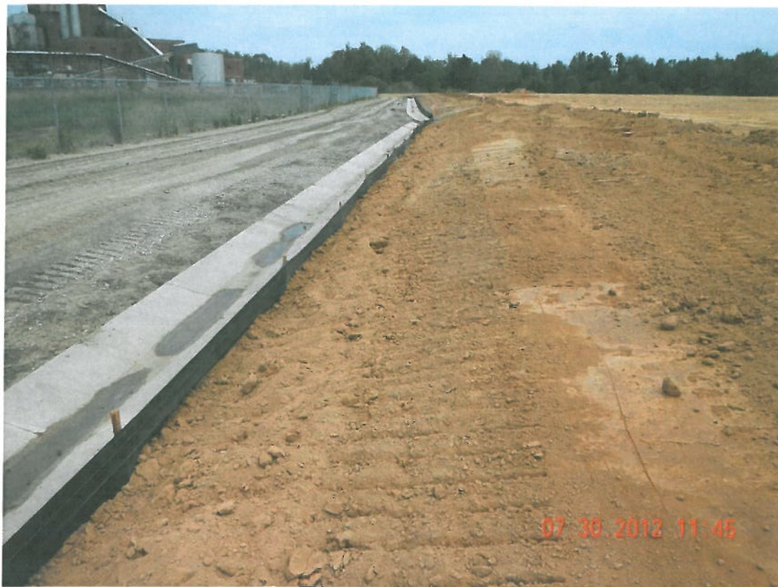
Photograph 7 ▲ - Backfill against paved gutter facing north
