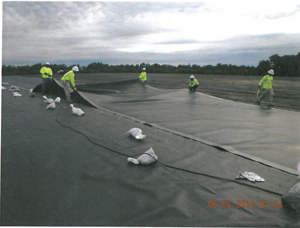
Photograph 1 ▲ - Installing geomembrane facing northeast
