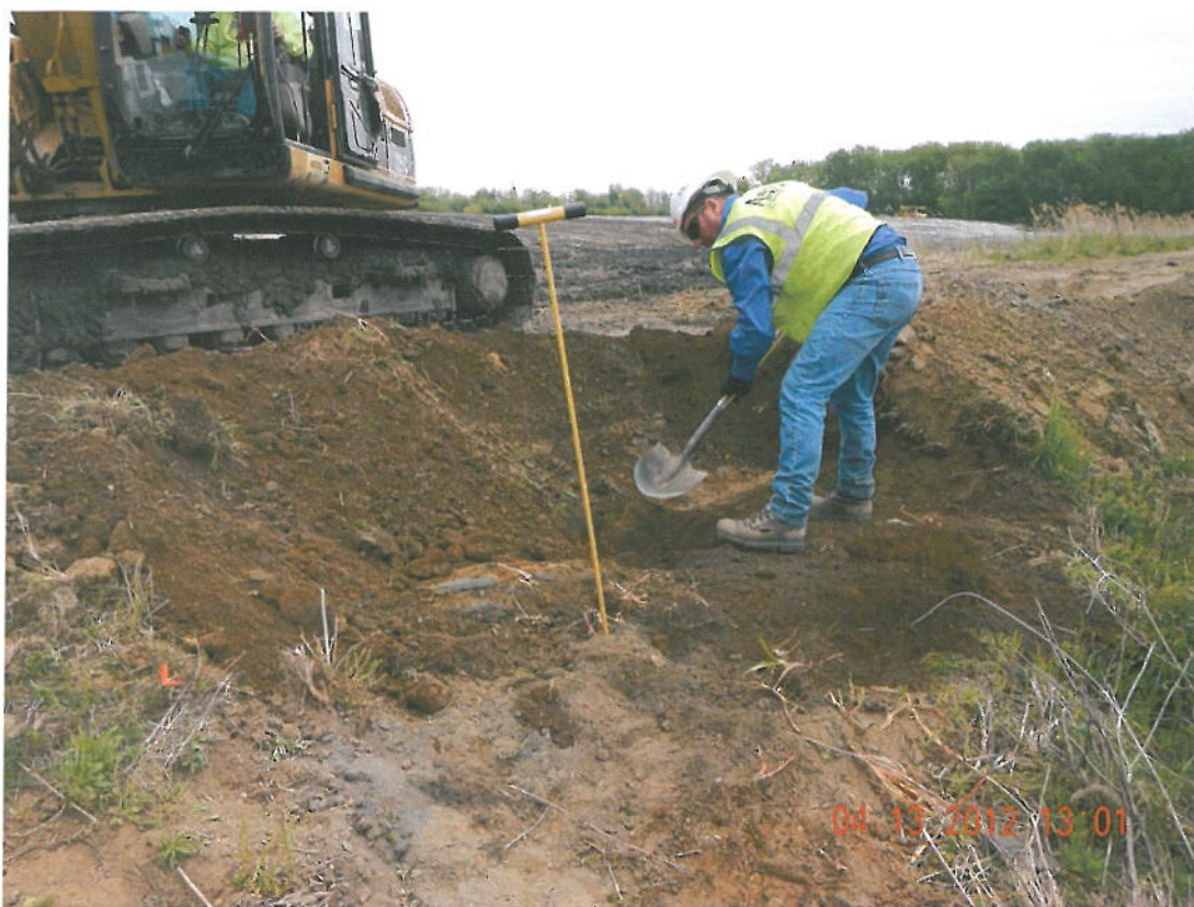
Photograph 9 ▲ - Exposing existing HDPE drainage pipe on embankments facing northwest
