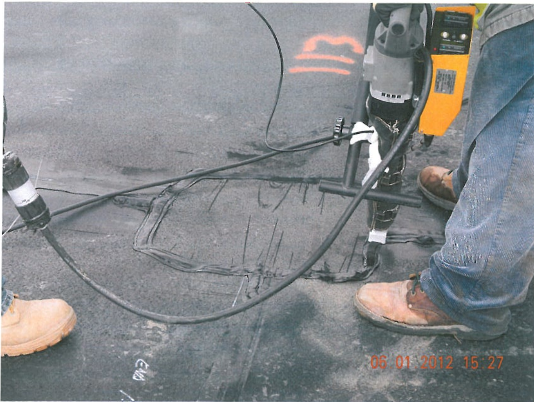
Photograph 13 ▲ - Extrusion welding repair facing east
