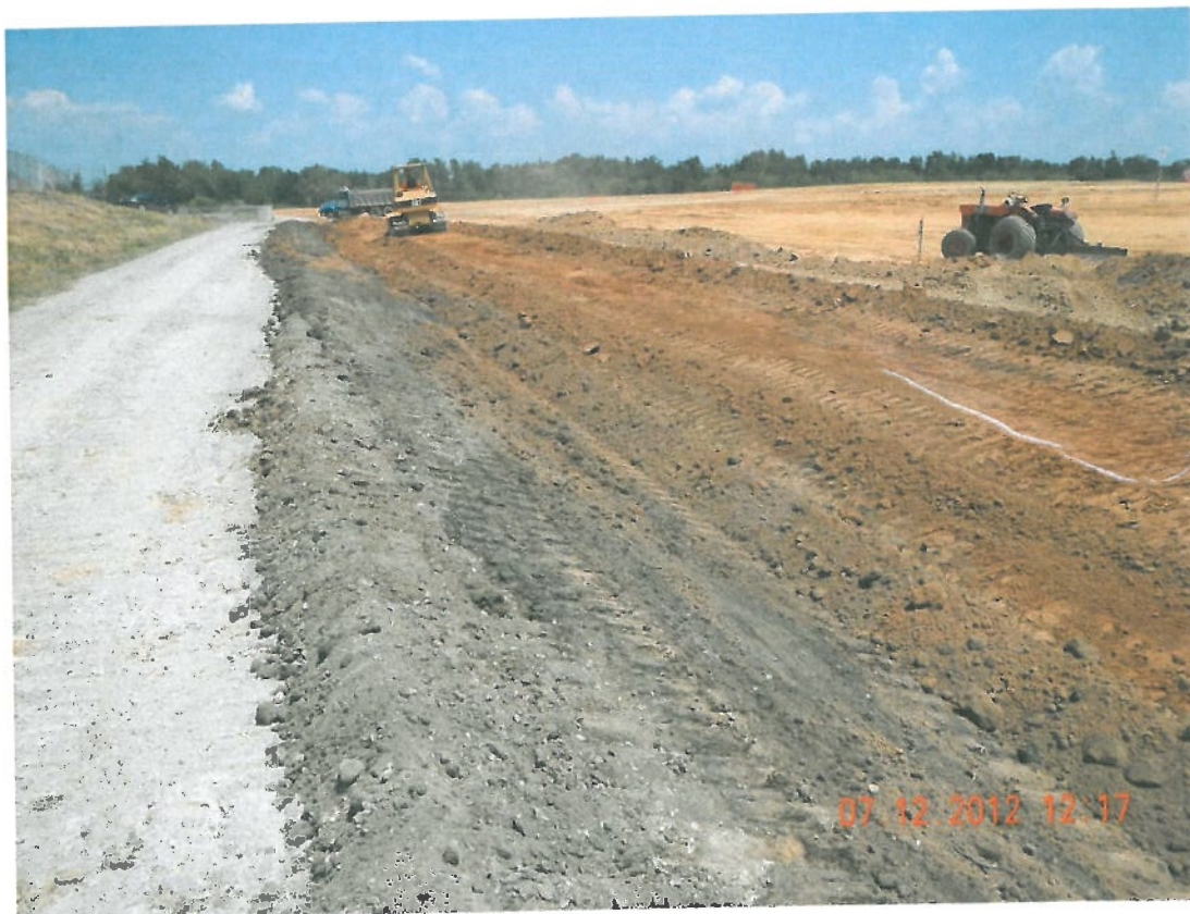
Photograph 6 ▲ - Grading paved gutter facing north
