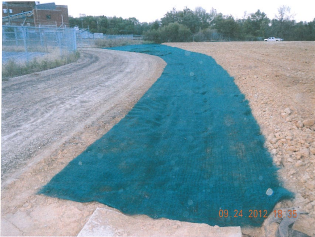
Photograph 7 ▲ - Installing turf reinforcement mat facing north
