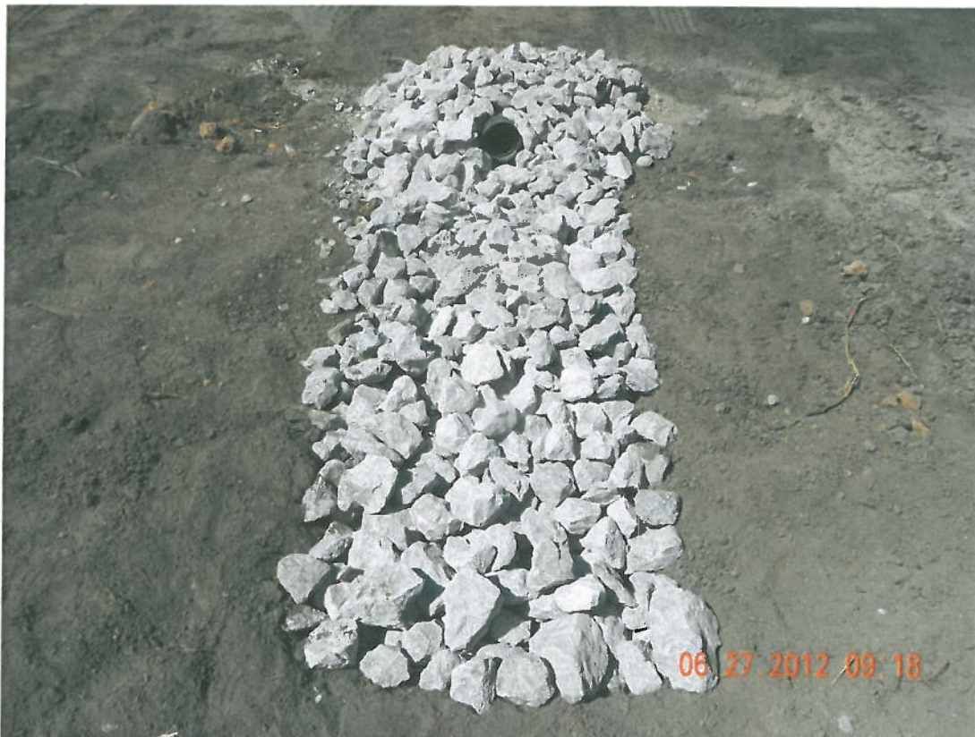
Photograph 8 ▲ - Riprap splash pad for anchor trench drains facing southwest
