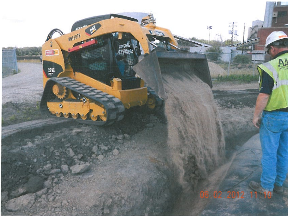
Photograph 15 ▲ - Backfilling anchor trench facing northwest
