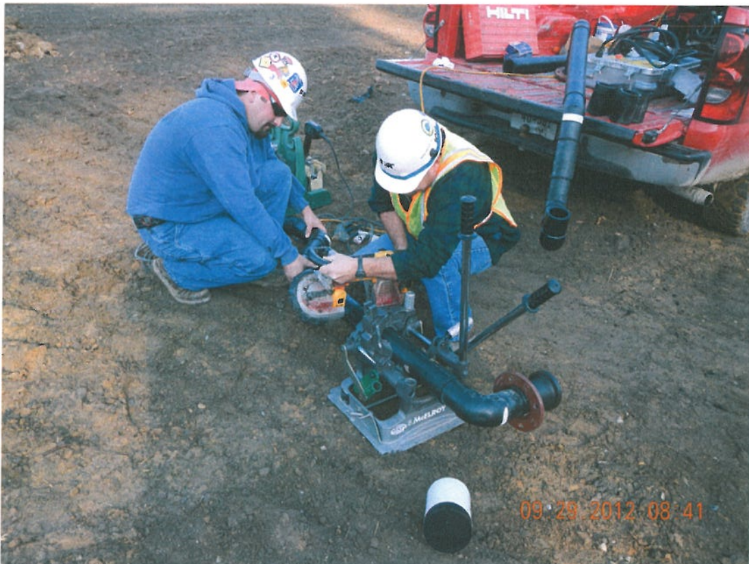
Photograph 8 ▲ - HDPE butt fusion welding facing northwest
