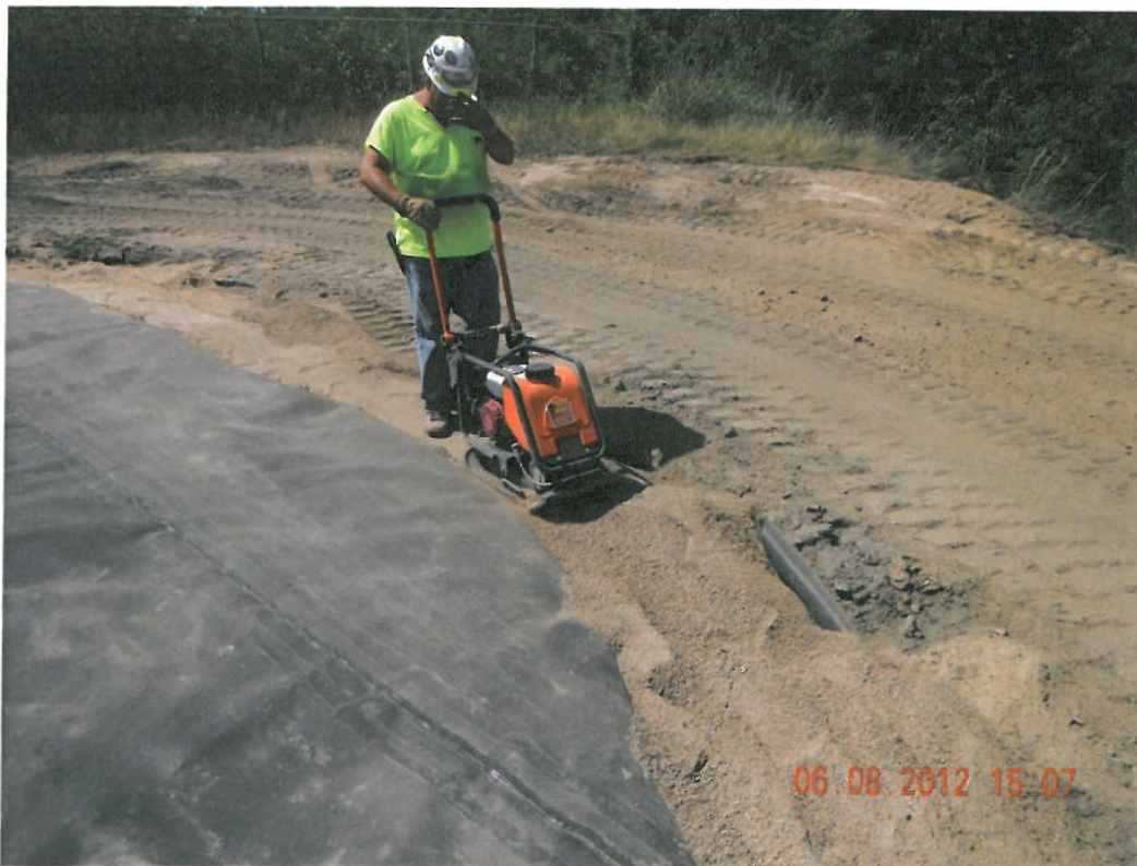
Photograph 10 ▲ - Compaction in anchor trench facing north
