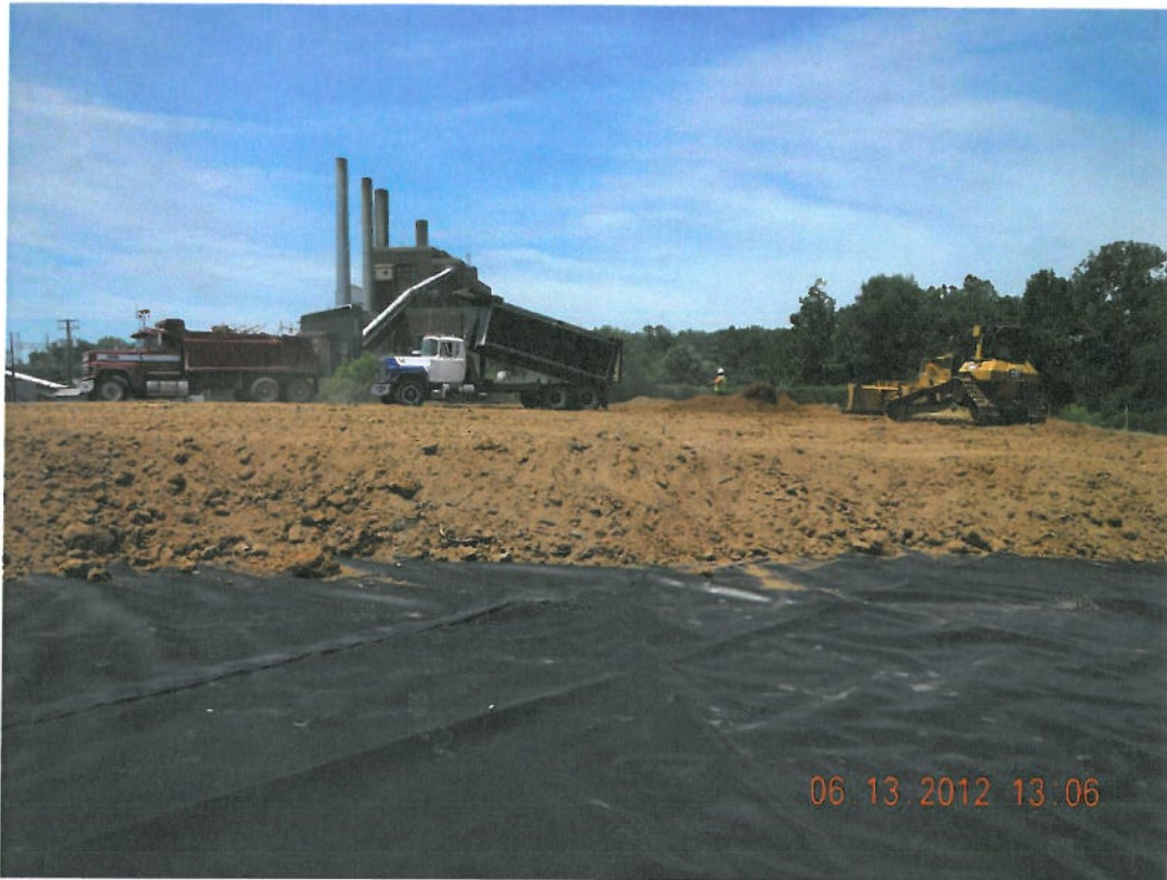
Photograph 5 ▲ - Clay placement in Quadrant A facing north
