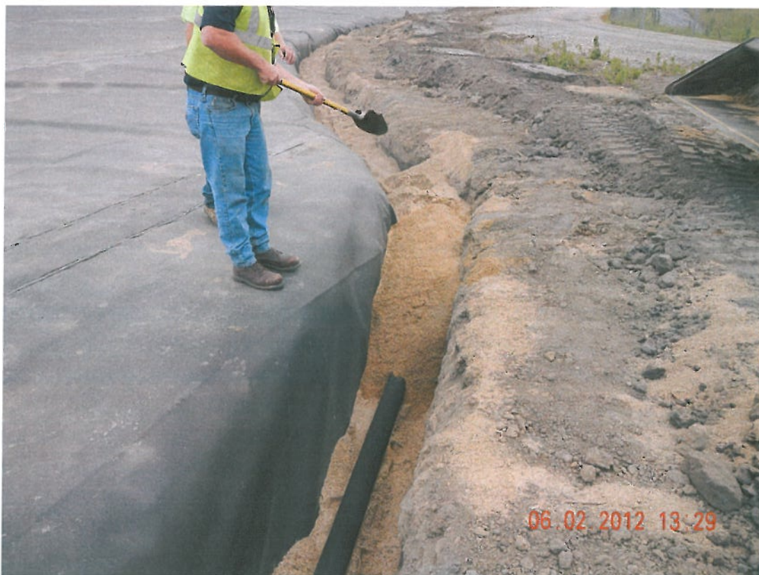
Photograph 16 ▲ - Backfilling anchor trench with drainage pipe facing southeast
