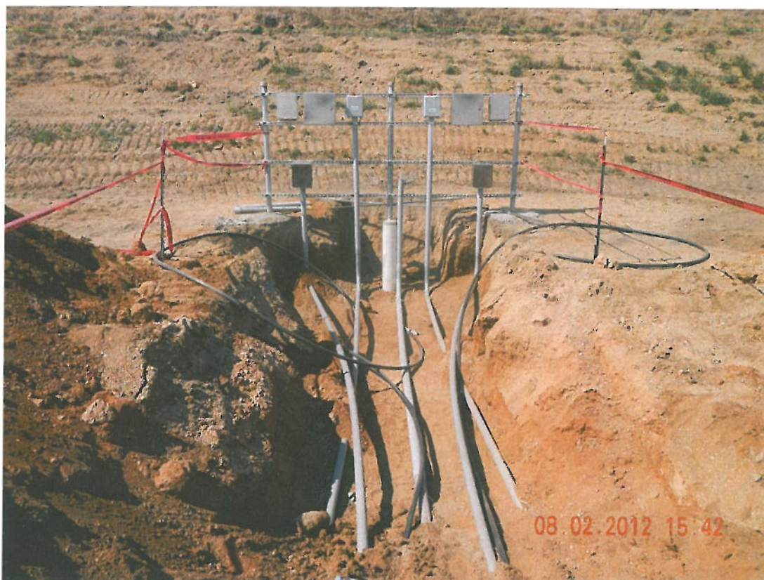
Photograph 16 ▲ - West pump control panel installation facing north
