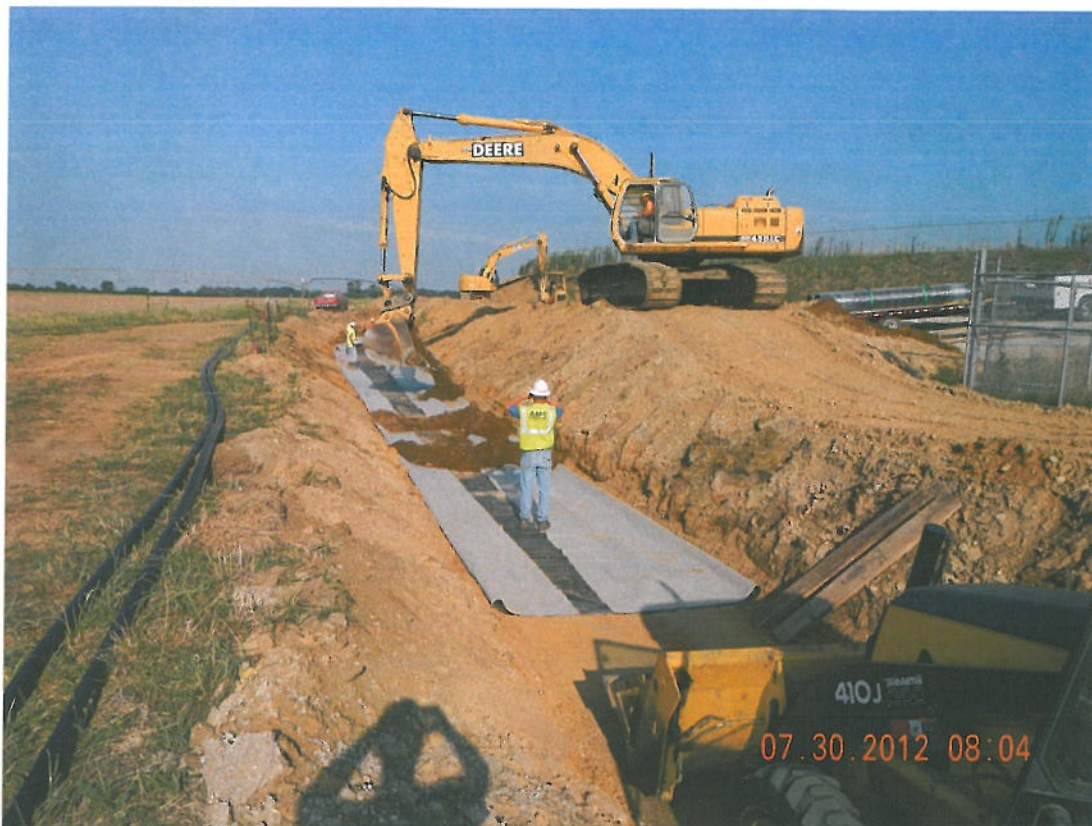
Photograph 4 ▲ - GCL backfill facing west
