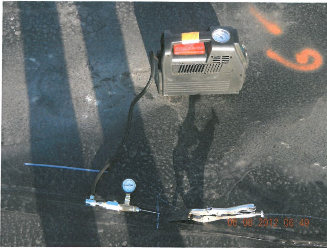
Photograph 9 ▲ - Air test on fusion weld facing west
