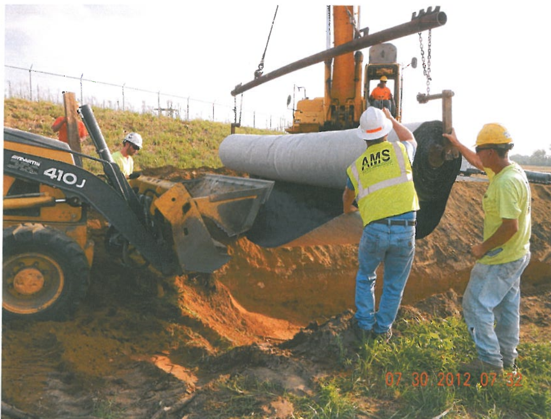
Photograph 2 ▲ - GCL deployment facing northeast
