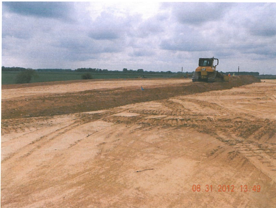
Photograph 10 ▲ - Slope diversion berm construction facing west
