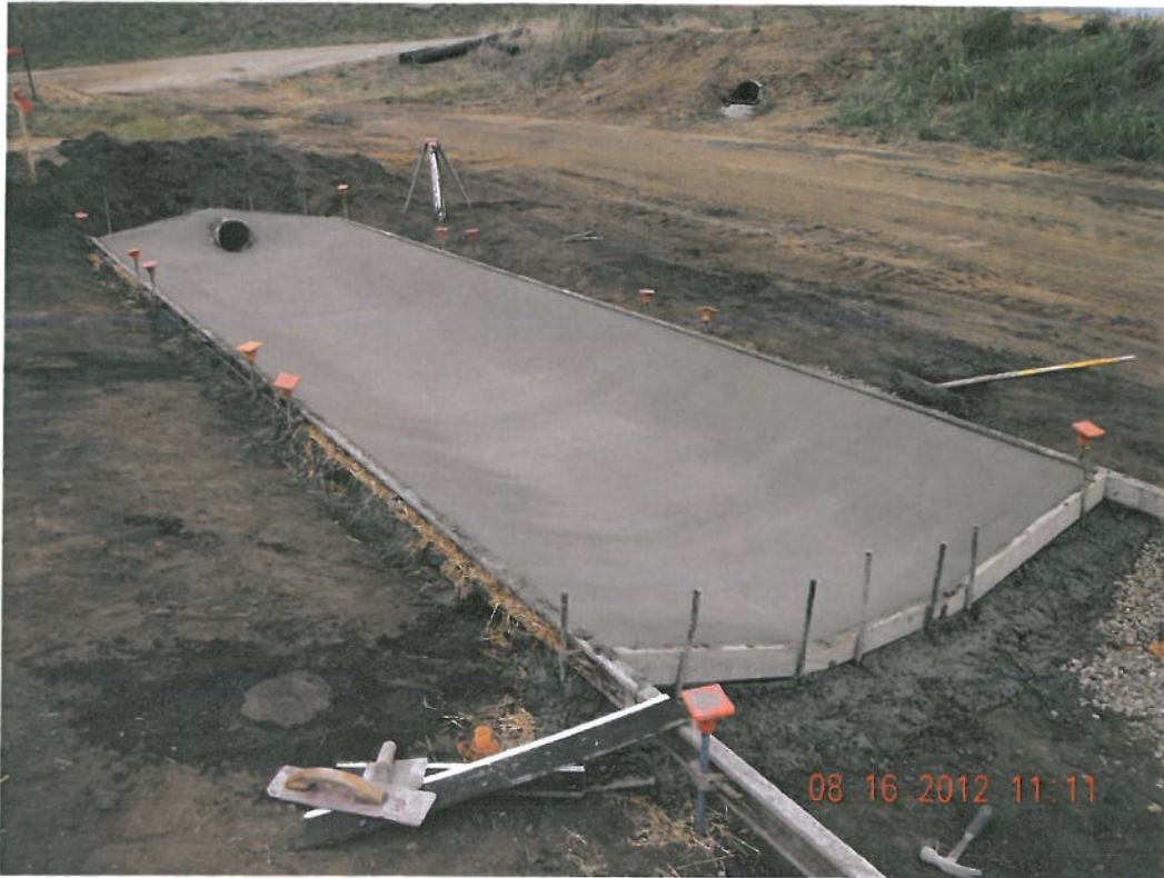
Photograph 11 ▲ - Paved ditch construction facing northwest
