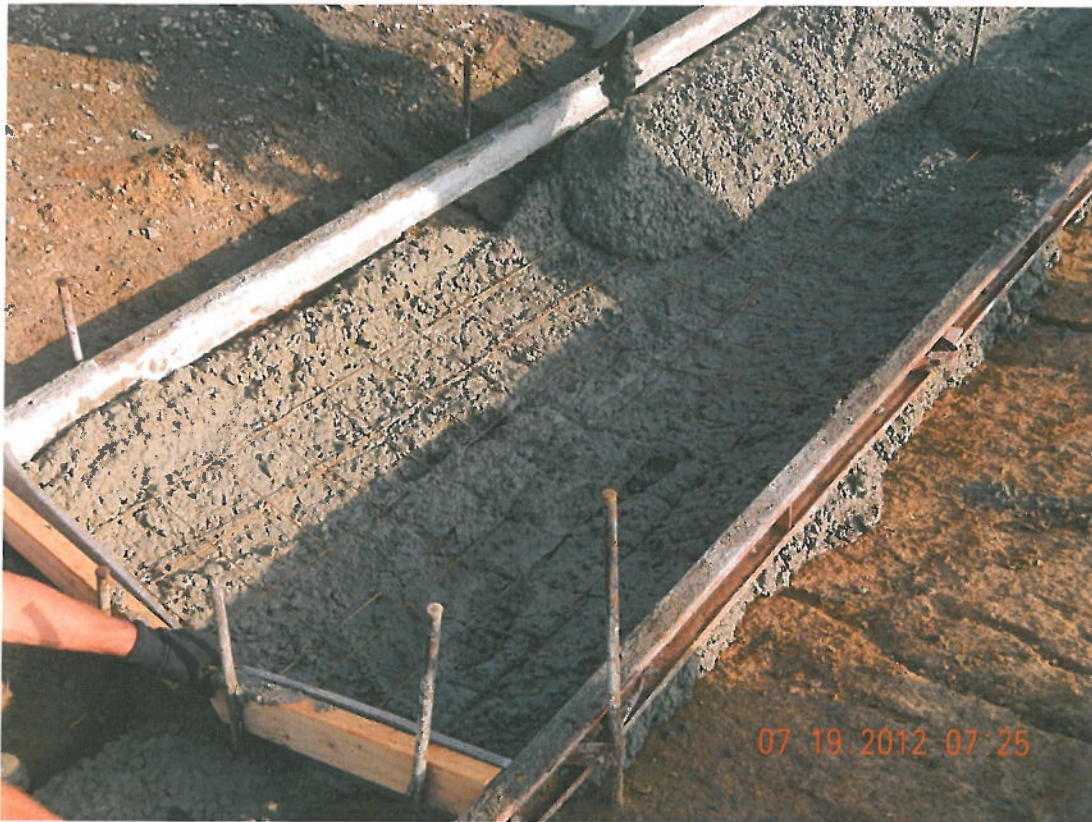
Photograph 9 ▲ - Pouring paved gutter facing northwest
