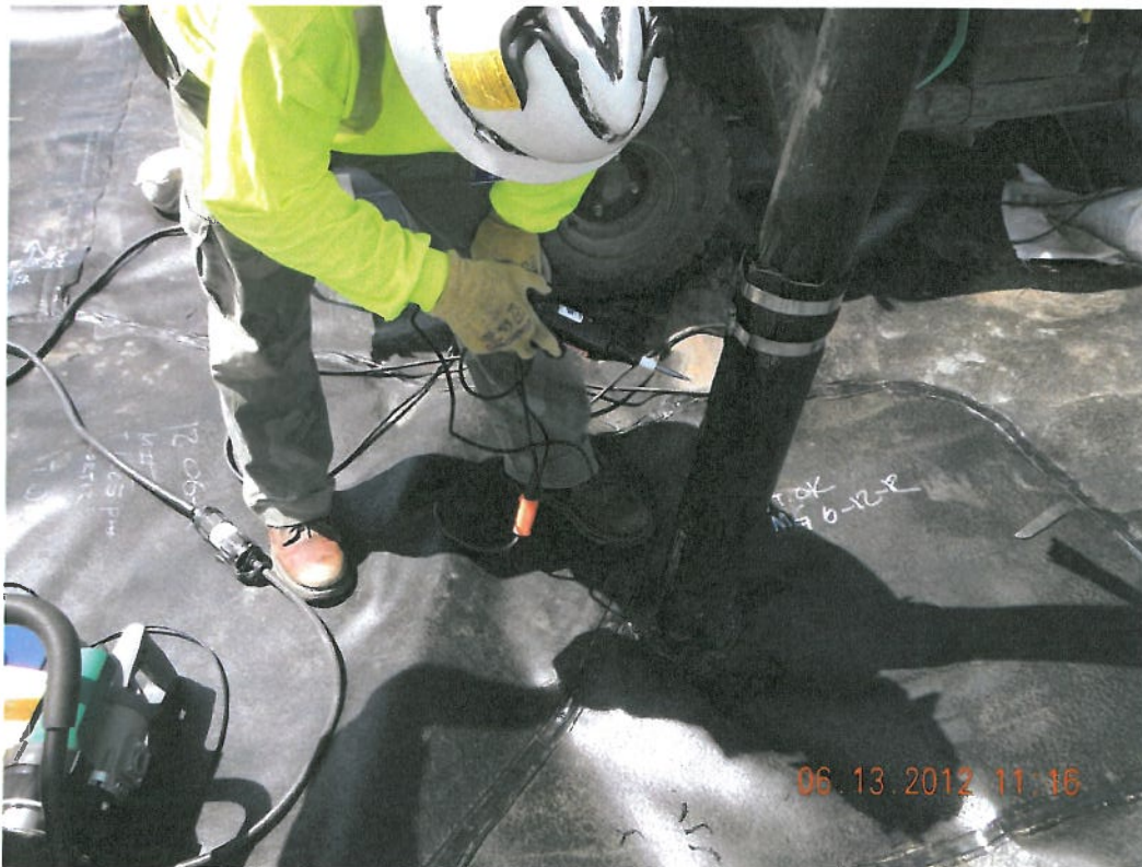
Photograph 4 ▲ - Spark testing cap vent boots facing south
