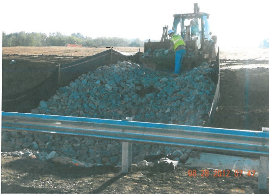
Photograph 3 ▲ - Repairing storm damage at box culvert facing east
