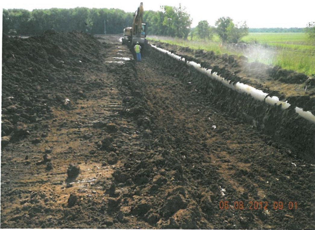
Photograph 3 ▲ - Digging new grade for 18" HDPE pipe facing east
