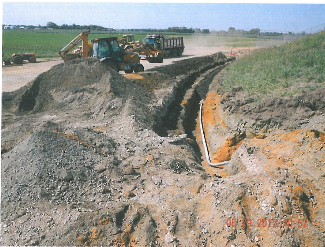
Photograph 7 ▲ - Installing PVC conduit for electric facing southwest
