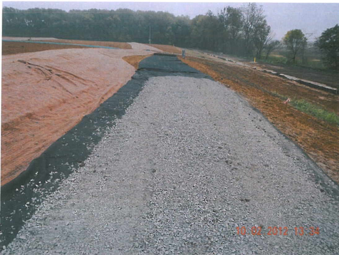
Photograph 8 ▲ - Gravel surfacing for new access road facing east
