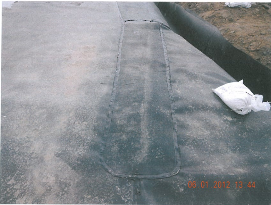
Photograph 9 ▲ - Typical geomembrane repair facing south
