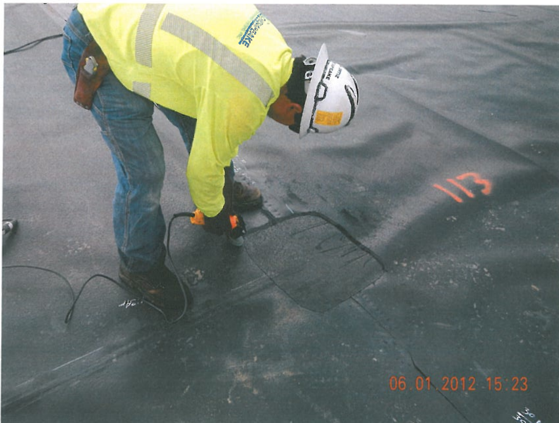
Photograph 12 ▲ - Grinding edge of patch for good deal facing northeast
