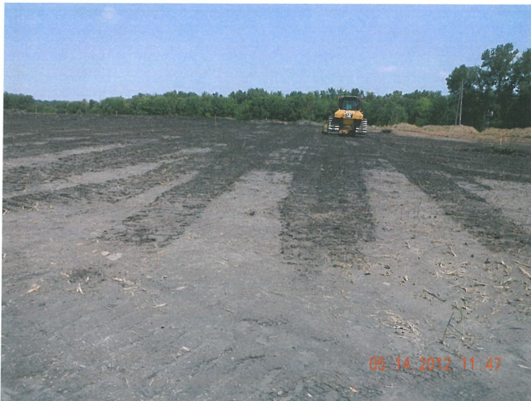
Photograph 4 ▲ - Final grading Quadrant D facing north
