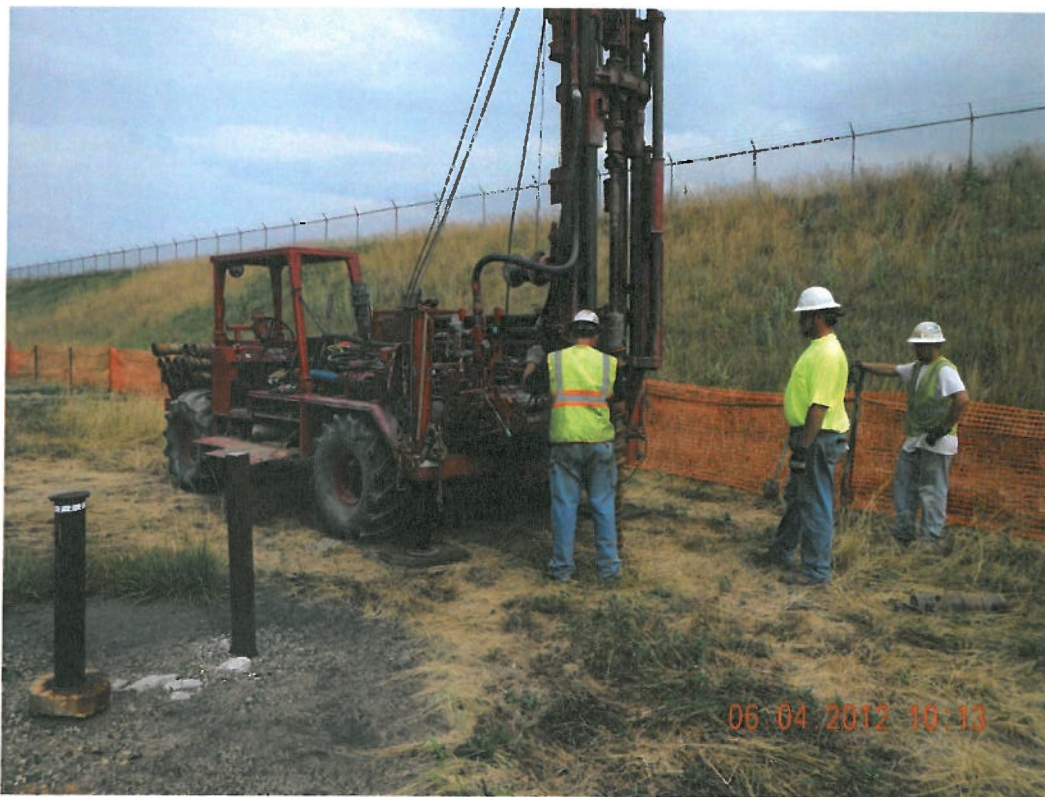
Photograph 2 ▲ - Installing monitoring well MW-2R facing northwest
