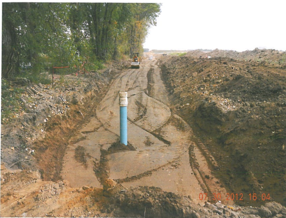
Photograph 9 ▲ - GCL backfill compaction facing west
