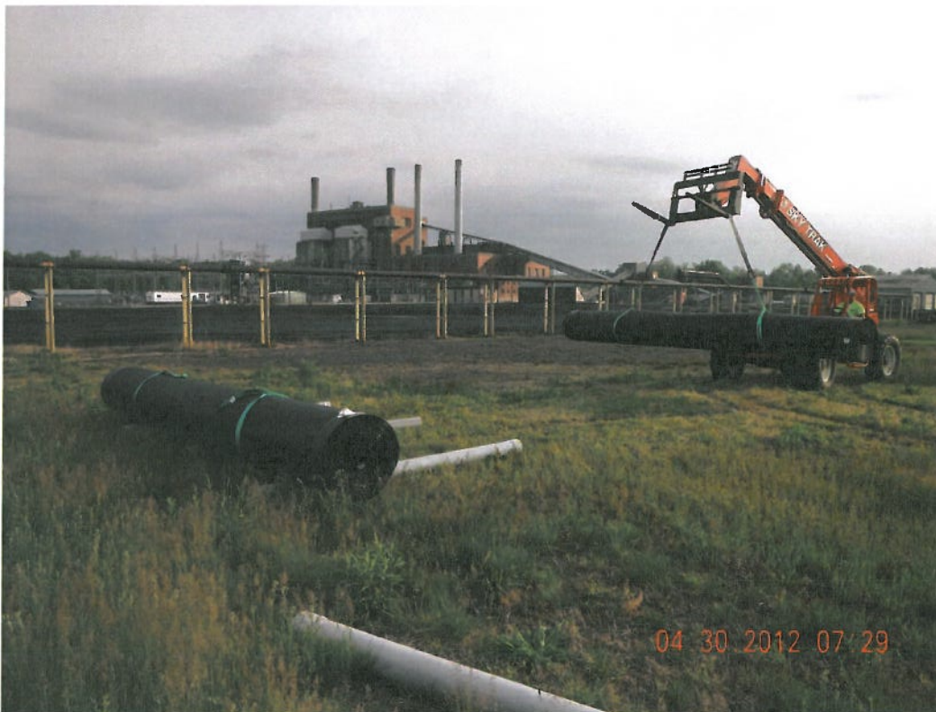
Photograph 2 ▲ - Unloading 40 mil HDPE geomembrane facing south
