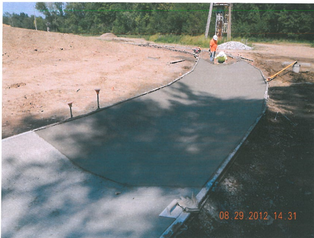
Photograph 8 ▲ - Paved ditch construction facing northeast
