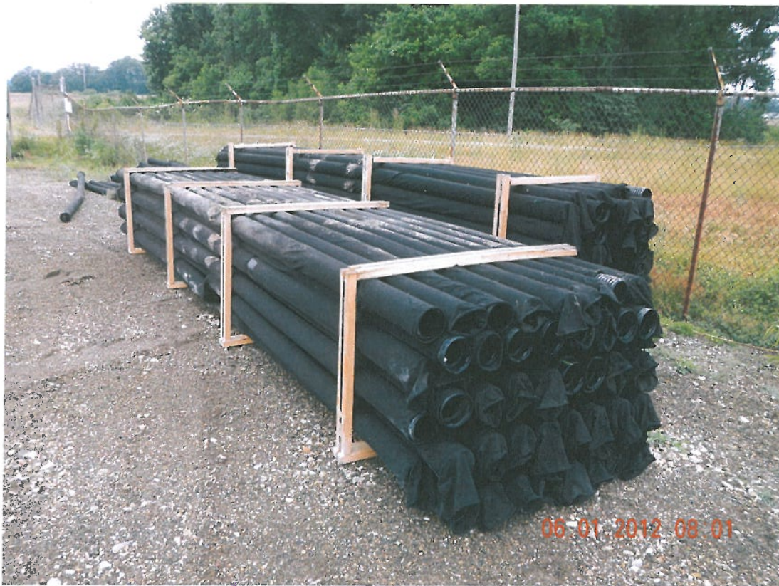
Photograph 7 ▲ - Perforated 4" drainage pipe for anchor trench facing northwest
