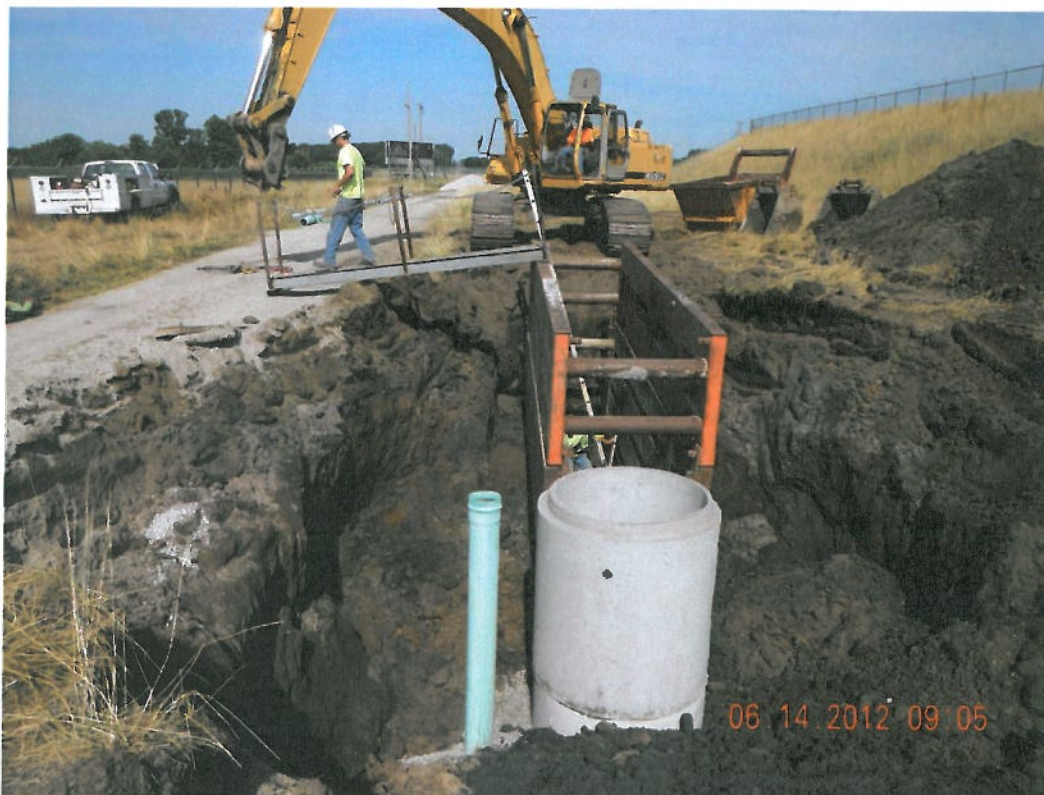
Photograph 8 ▲ - Installing PCP-1 facing west
