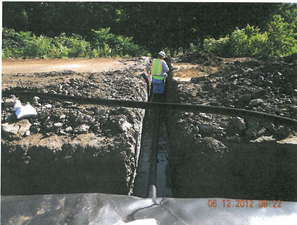
Photograph 2 - Drainage pipe placement in anchor trench facing northeast
