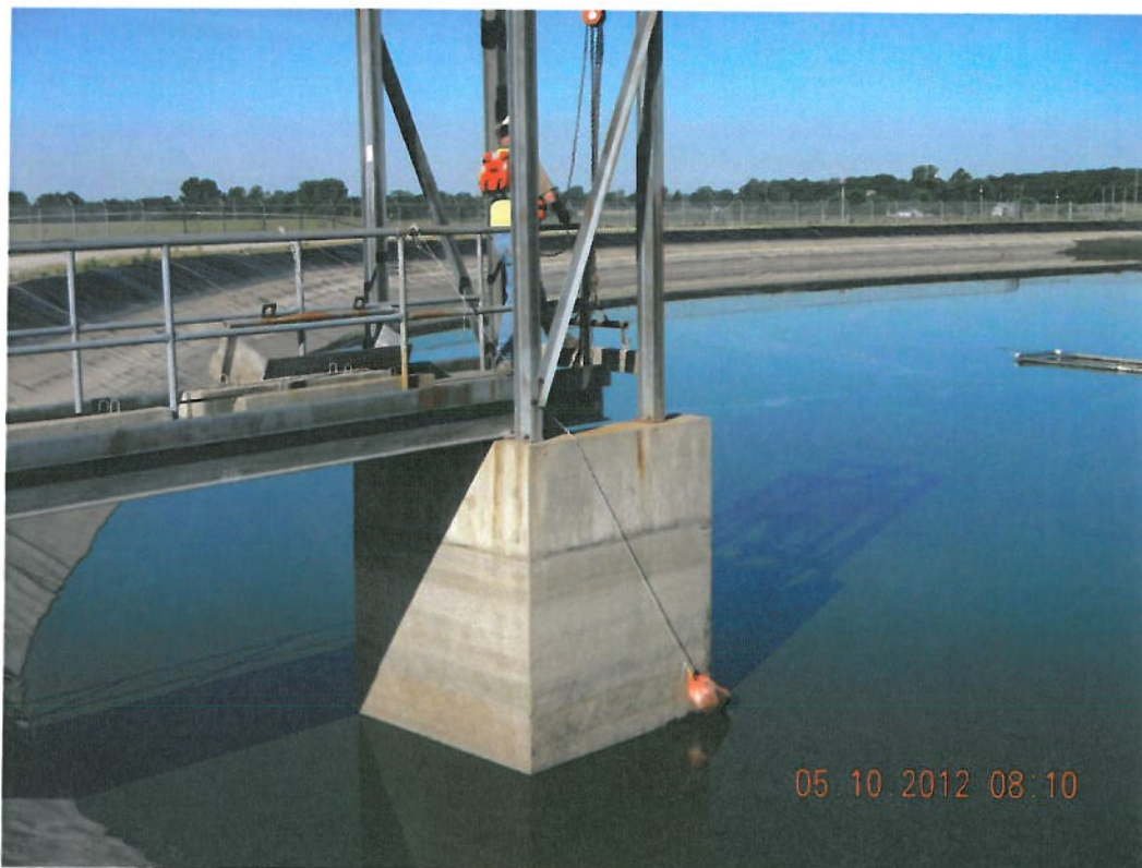
Photograph 6 ▲ - Placing stop logs in Ash Pond B outfall facing southwest
