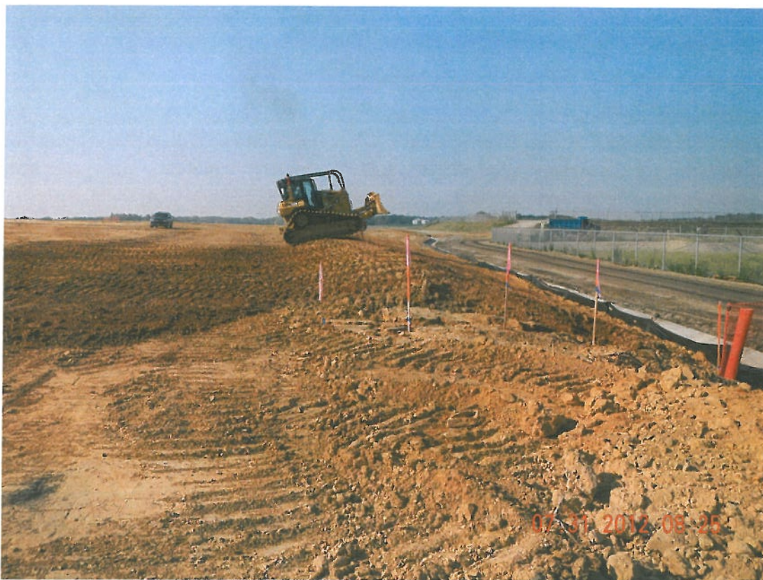
Photograph 10 ▲ - Slope diversion berm construction facing south
