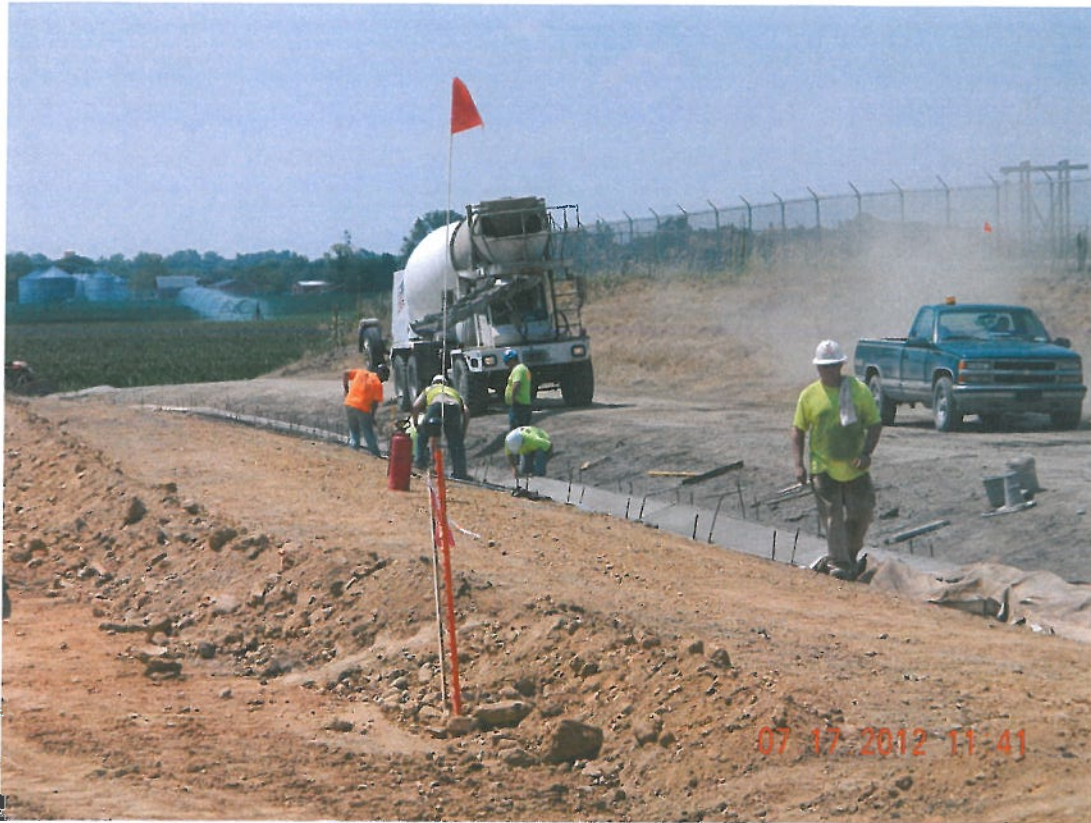
Photograph 7 ▲ - Pouring paved gutter facing southwest
