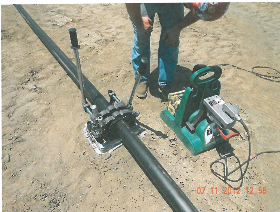
Photograph 9 ▲ - Butt fusion welding 3-inch HDPE pipe facing west
