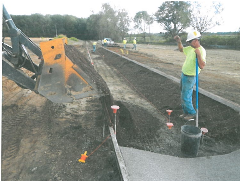
Photograph 4 ▲ - Placing IDOT CA-6 bedding for the paved ditch facing east.
