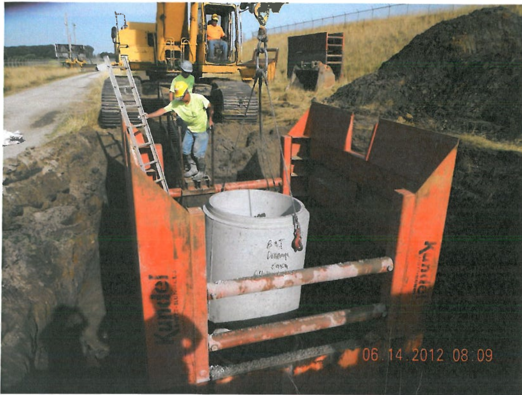
Photograph 7 ▲ - Installing DS-1 manhole facing west
