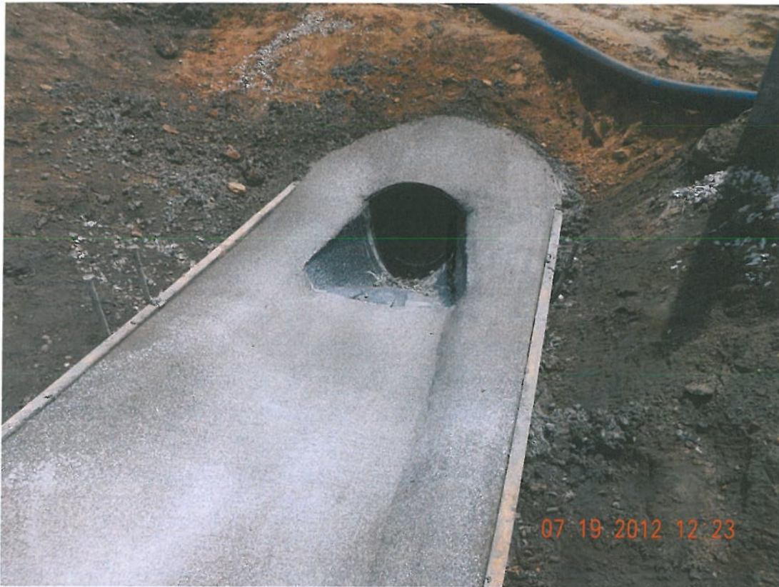
Photograph 11 ▲ - Curing paved gutter facing southeast
