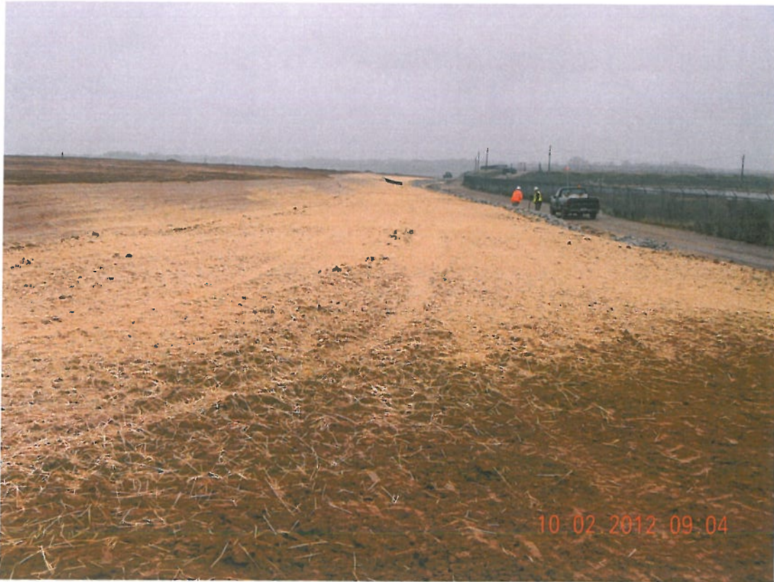
Photograph 7 ▲ - Straw mulch placement facing south
