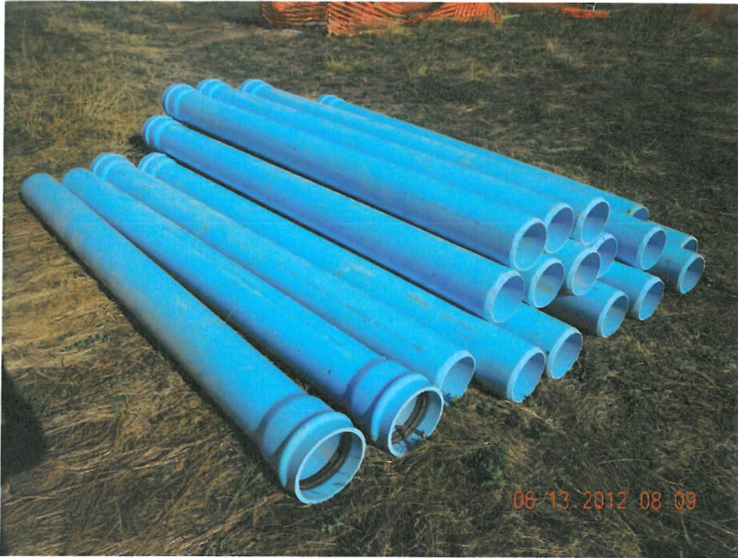
Photograph 3 ▲ - 8-inch perforated DR18 PVC C900 pipe for PCP facing northwest
