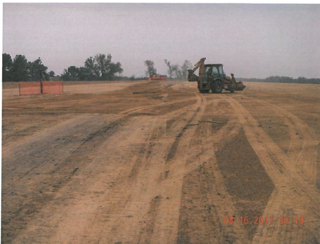
Photograph 8 ▲ - Grading Ash Pond D cap facing southeast
