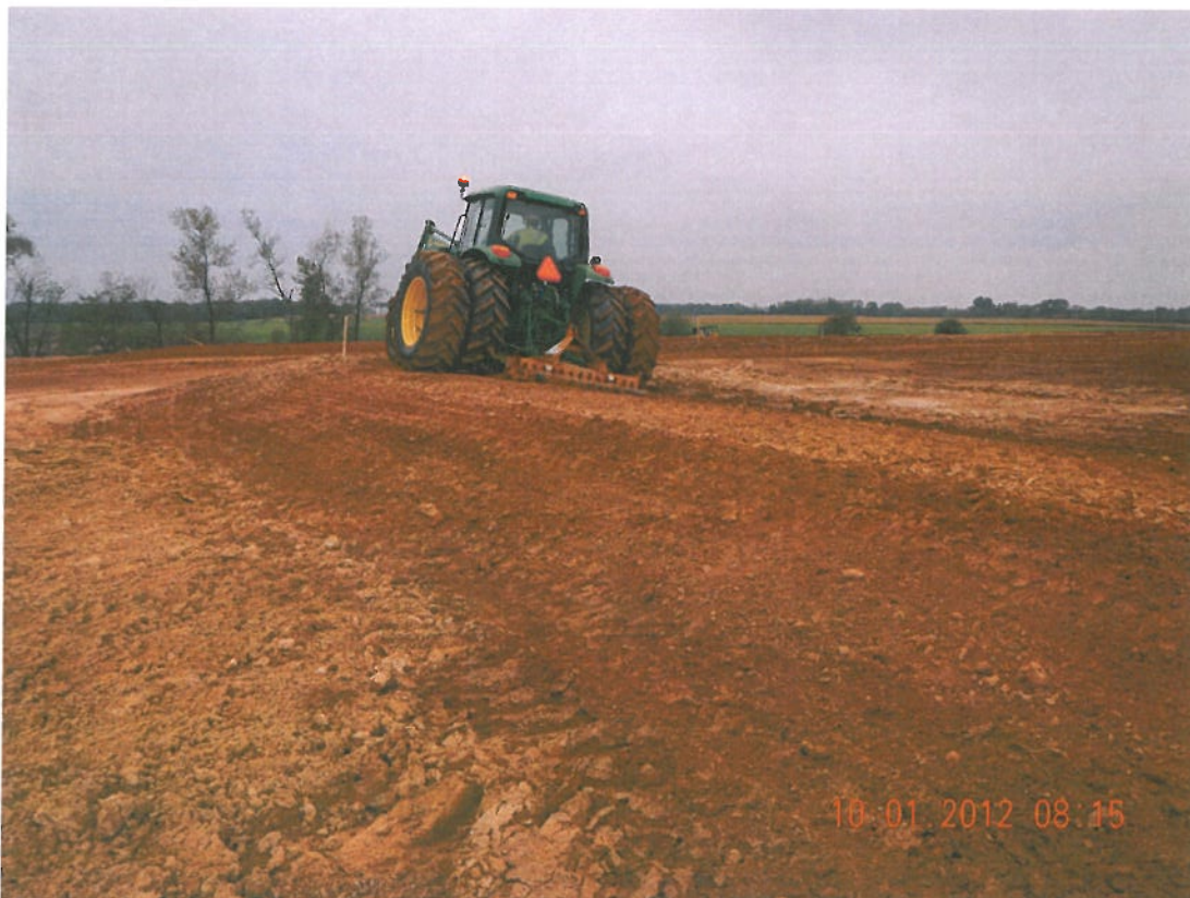
Photograph 2 ▲ - Aerating slope diversion berms facing southwest
