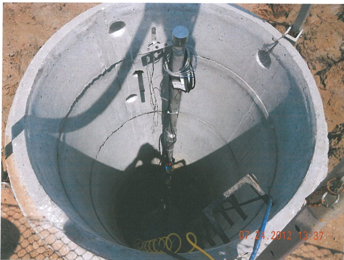
Photograph 8 ▲ - DS-1 sump pump assembly installation facing east
