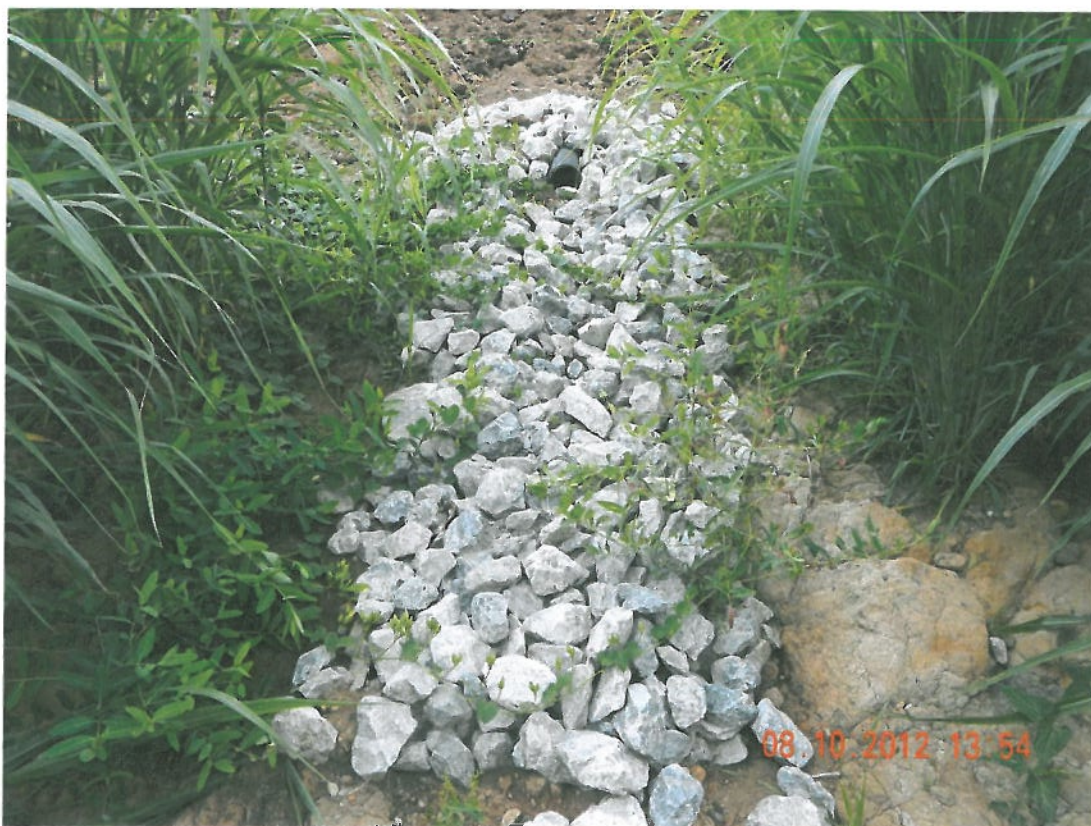
Photograph 8 ▲ - Anchor trench outlet toe drain repairs facing west
