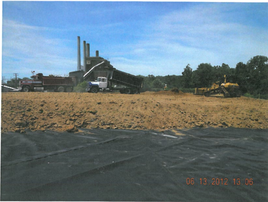
Photograph 5 ▲ - Clay placement in Quadrant A facing north
