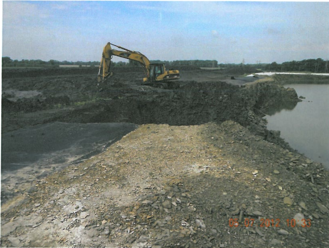
Photograph 1 ▲ - Digging trench in Ash Pond A facing west
