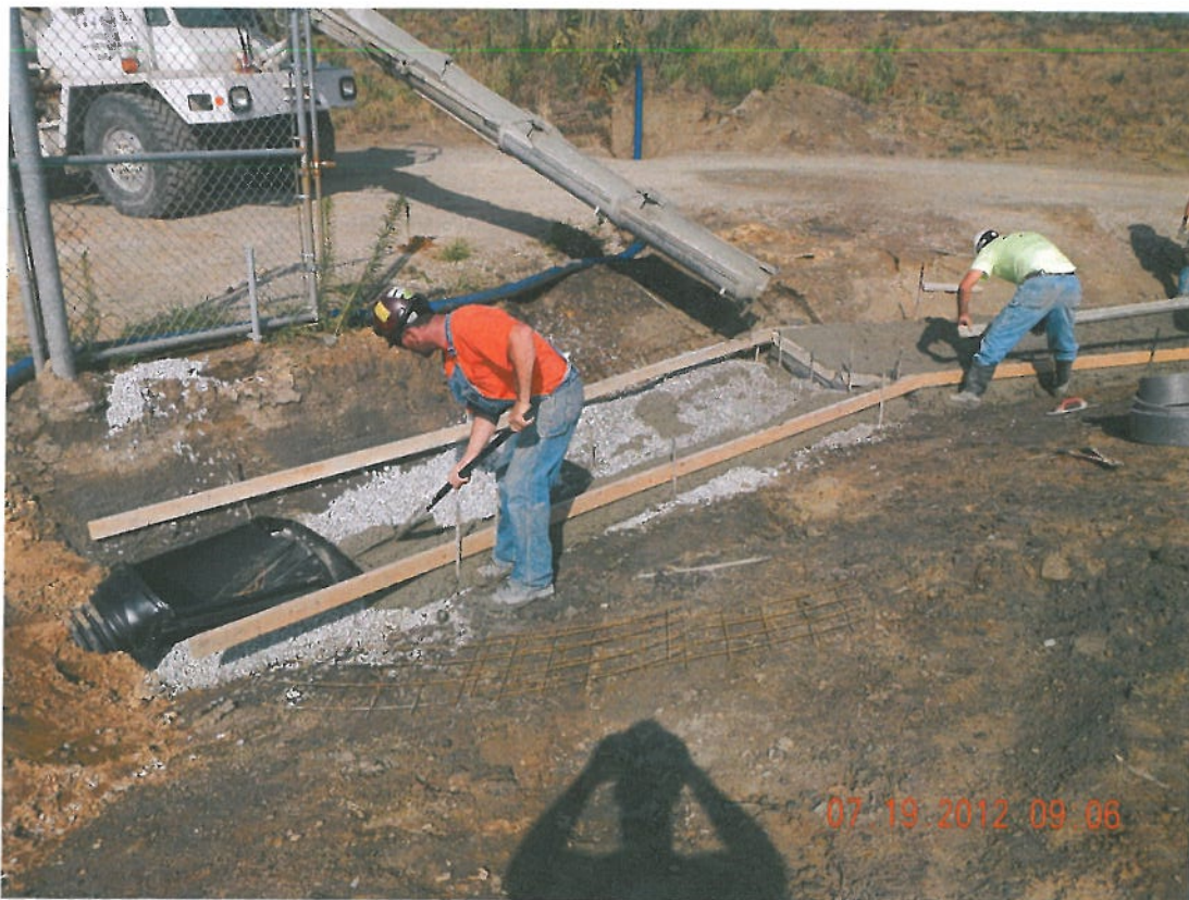
Photograph 10 ▲ - Pouring paved gutter facing southwest
