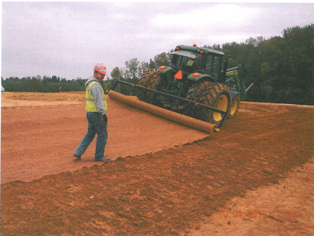
Photograph 6 ▲ - Installing erosion control blankets on berms facing northeast
