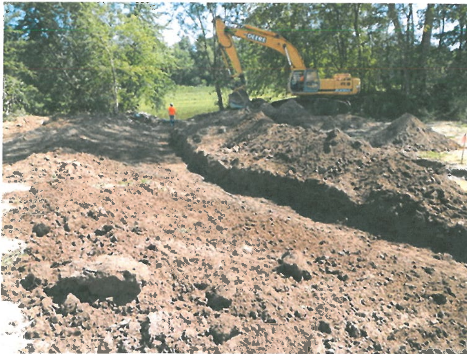
Photograph 2 ▲ - Grading for the paved ditch facing northeast.
