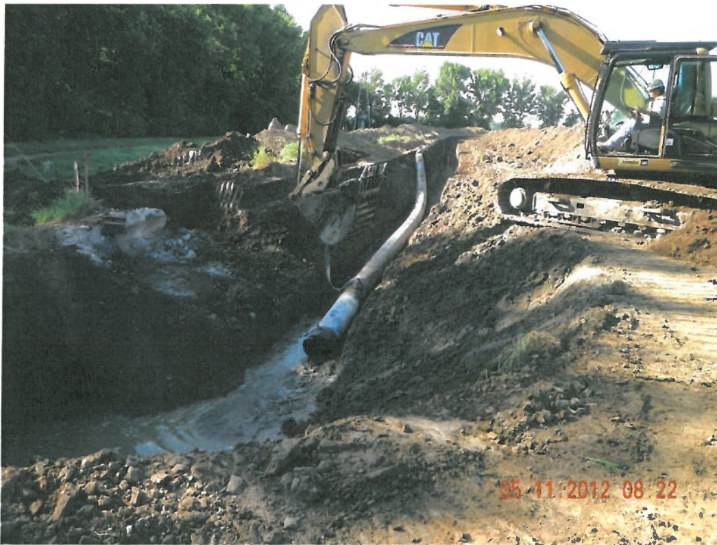
Photograph 10 ▲ - 18" HDPE pipe relocation facing southeast
