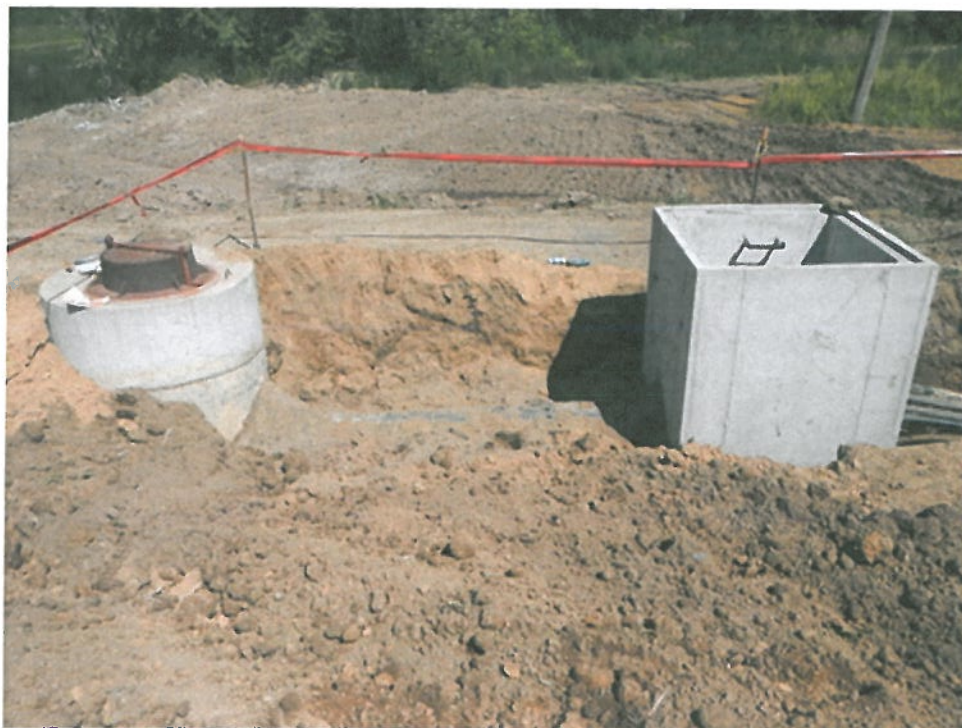
Photograph 5 ▲ - Collector box precast installation facing east.
