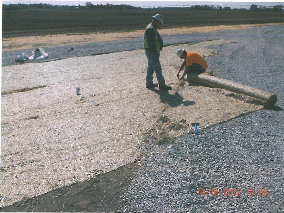
Photograph 1 ▲ - Installing straw blankets facing south
