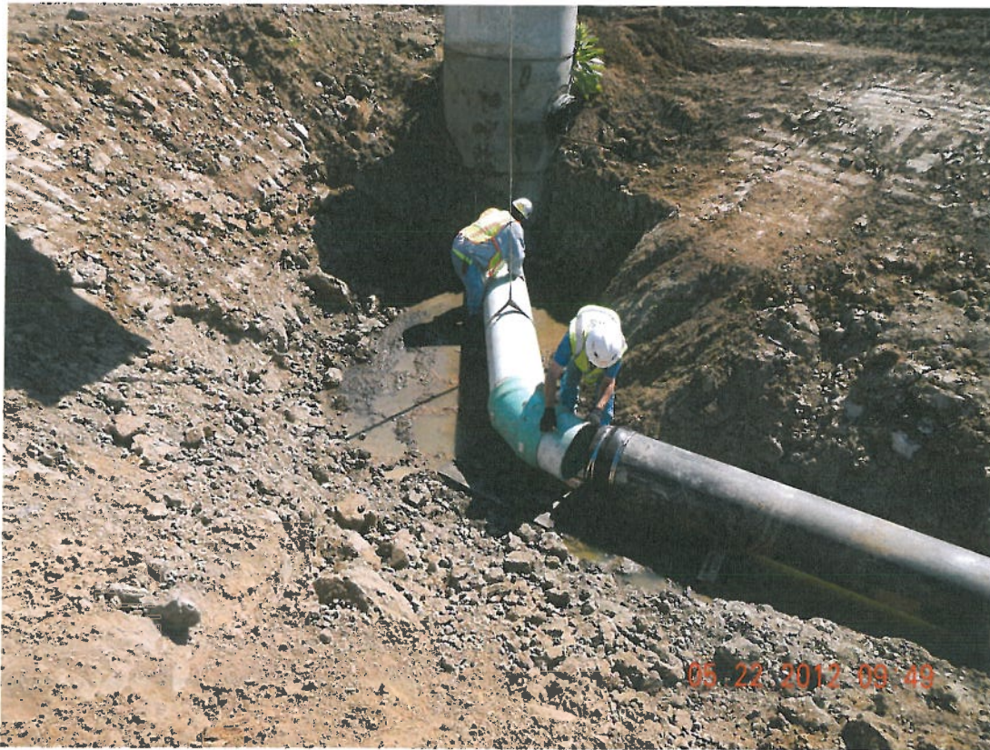
Photograph 5 ▲ - Connecting HDPE pipe to PVC pipe facing northeast
