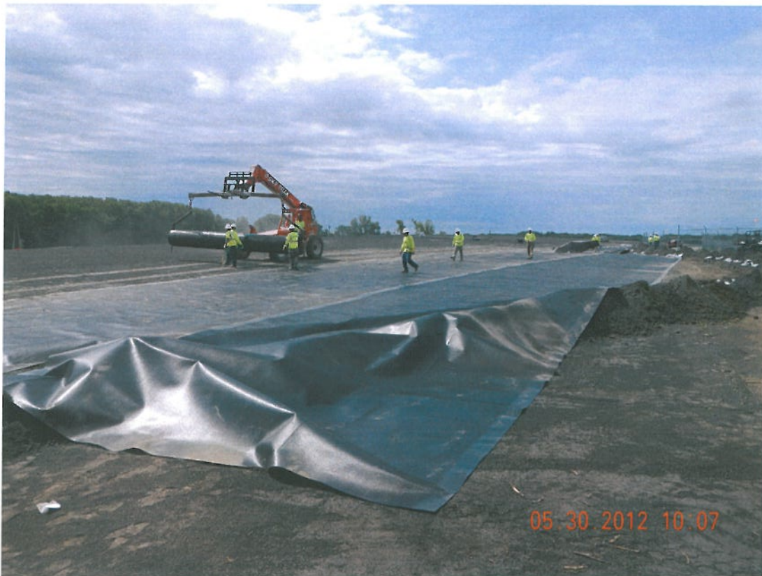
Photograph 2 ▲ - Geomembrane installation facing southeast
