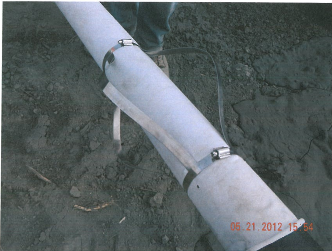
Photograph 3 ▲ - Cap vent filter sock and centralizer facing northeast
