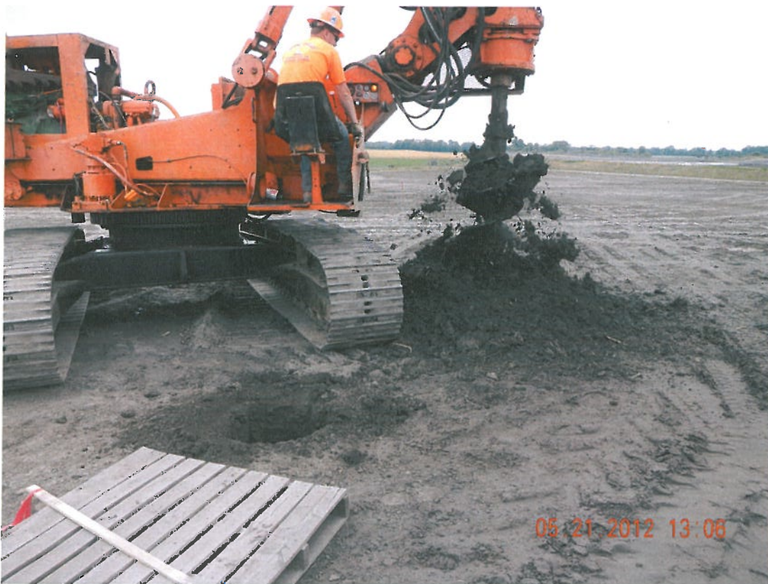
Photograph 2 ▲ - Drilling cap vents facing west
