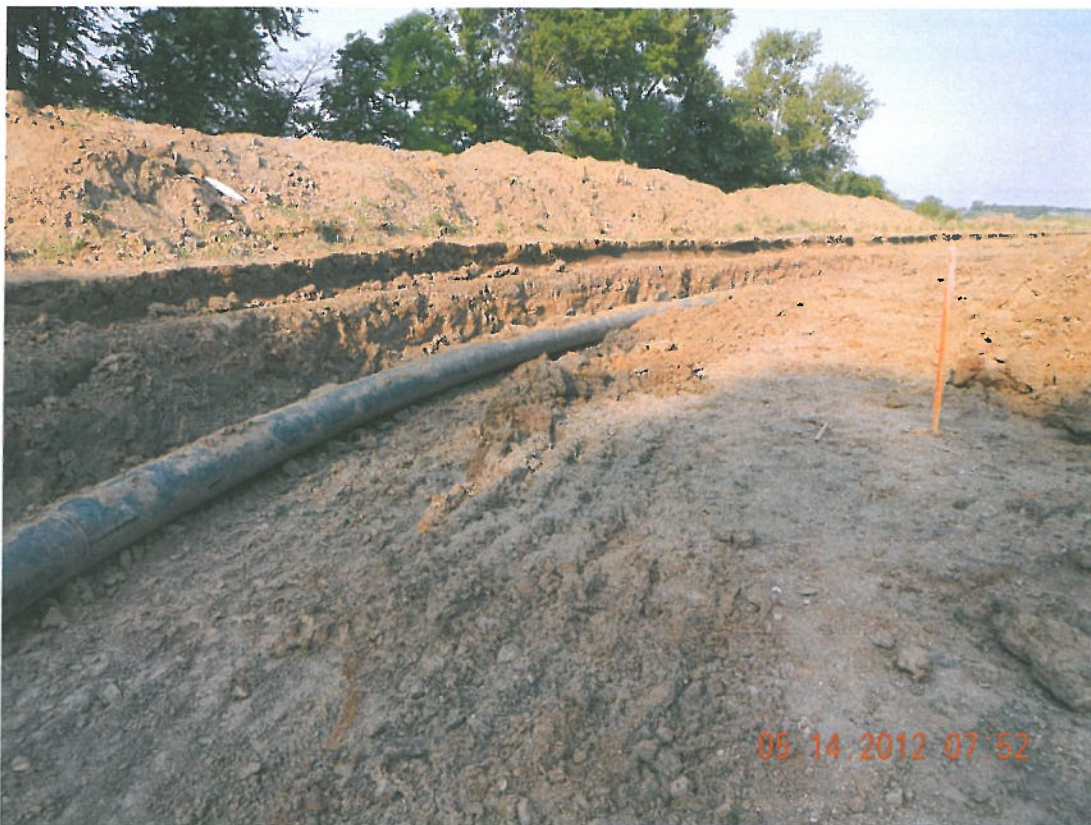
Photograph 2 ▲ - Relocated 18" HDPE pipe facing west
