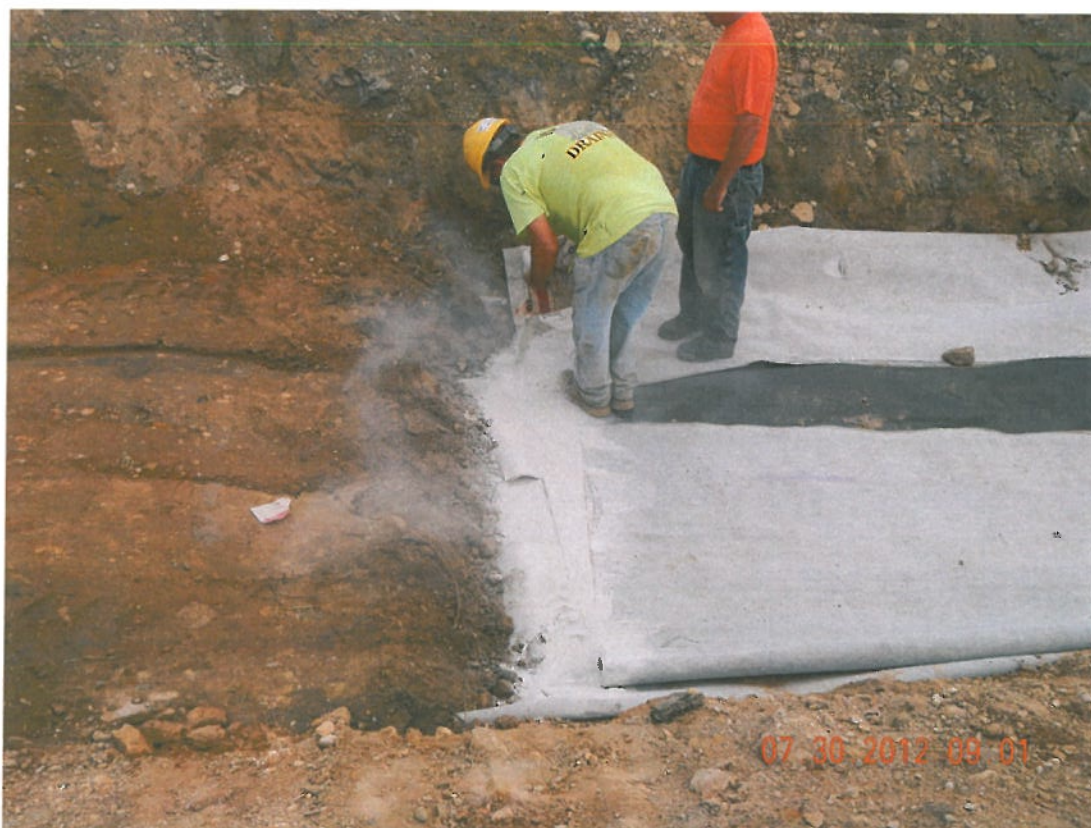
Photograph 6 ▲ - GCL seaming facing north
