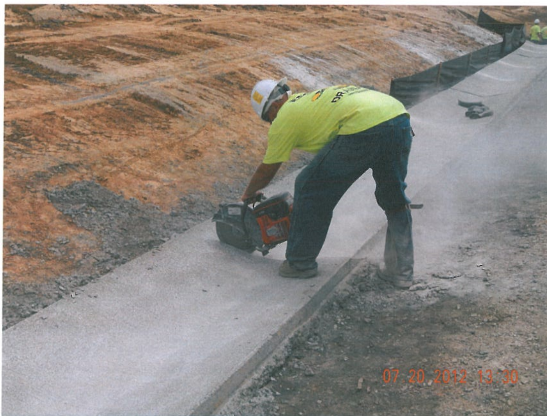
Photograph 14 ▲ - Saw cutting paved gutter facing east
