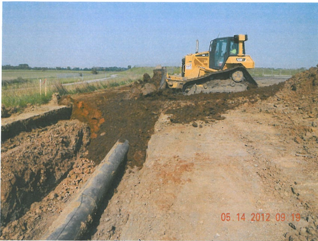
Photograph 3 ▲ - Backfilling relocated 18" HDPE pipe facing west
