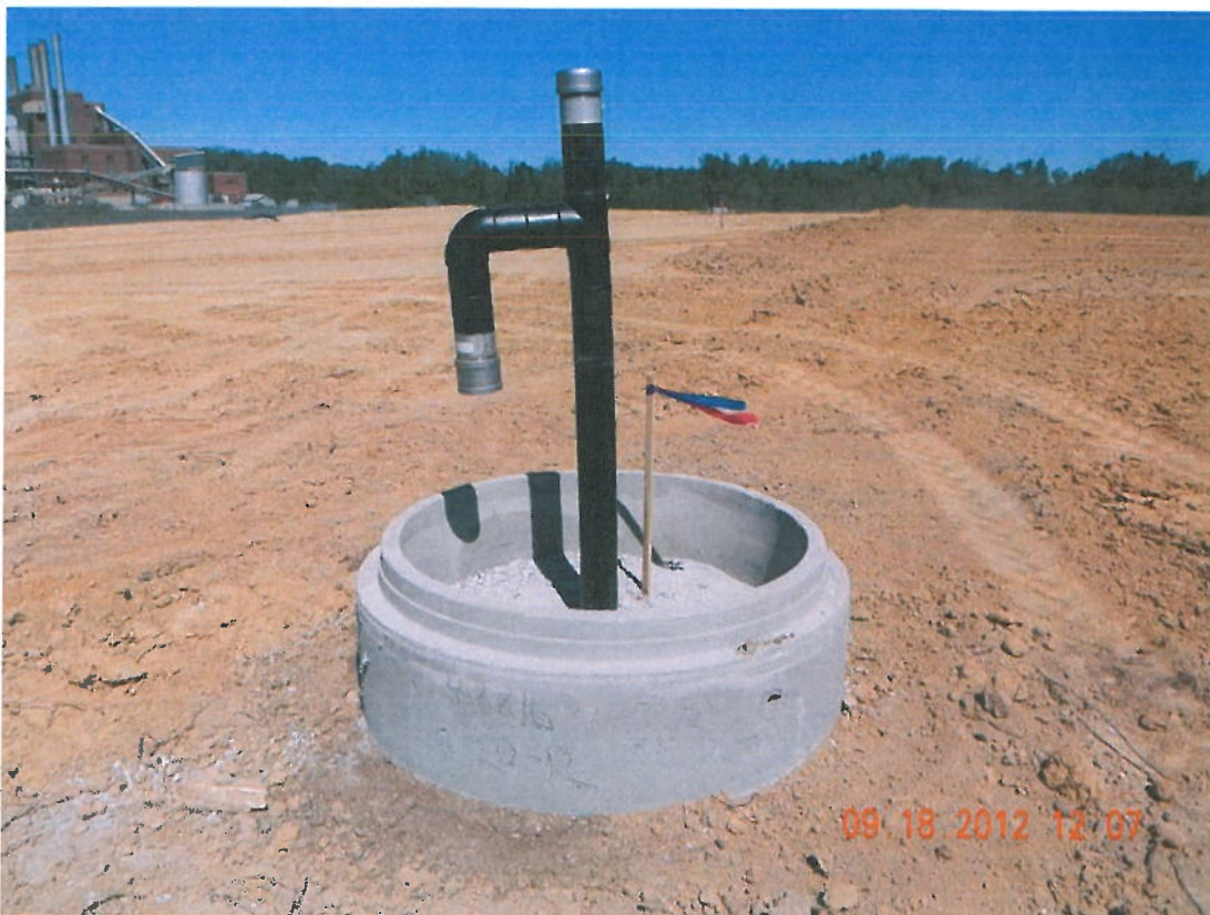
Photograph 4 ▲ - Rock bedding in cap vent protective barriers facing north
