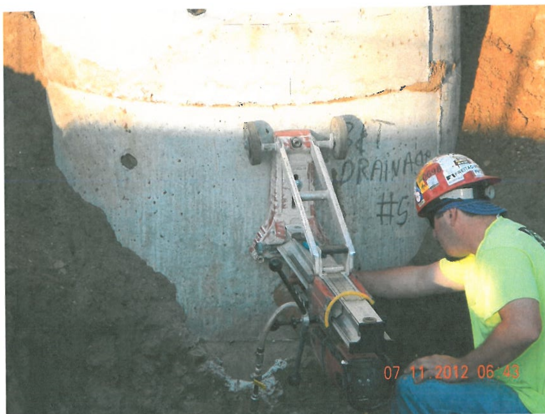
Photograph 7 ▲ - Coring holes for sump discharge in DS-2 facing west
