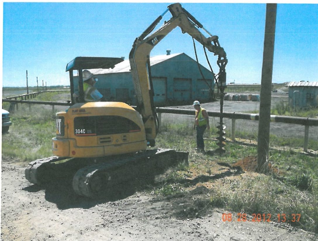
Photograph 4 ▲ - Power pole installation facing south
