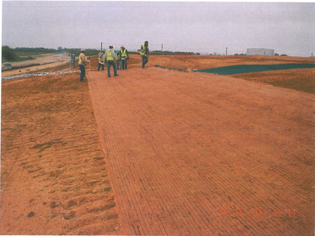
Photograph 5 ▲ - Installing erosion control blankets on berms facing east
