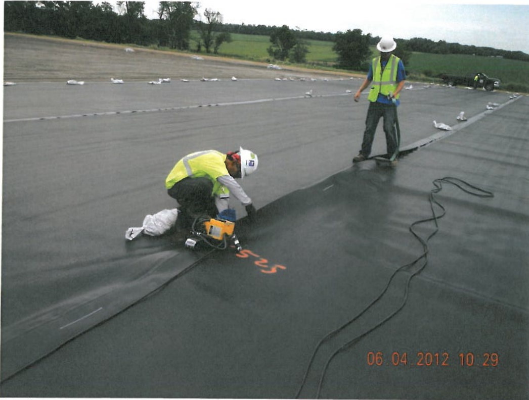
Photograph 3 ▲ - Fusion seaming geomembrane facing southeast
