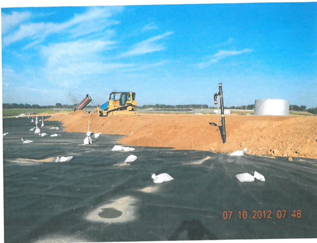
Photograph 5 ▲ - Clay placement facing west
