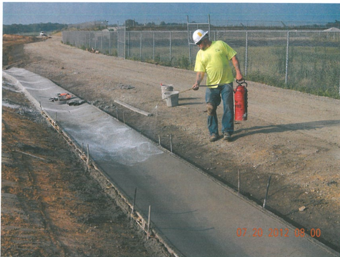
Photograph 12 ▲ - Curing paved gutter facing southwest
