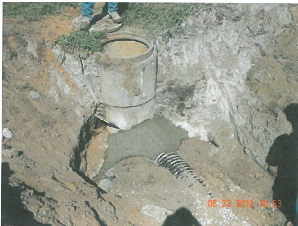
Photograph 8 ▲ - Field tile installation facing northwest.
