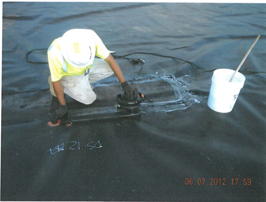
Photograph 7 ▲ - Vacuum testing extrusion welds facing southeast
