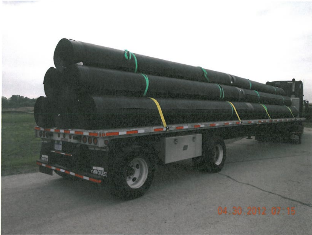
Photograph 1 ▲ - 40 mil HDPE geomembrane delivery facing south
