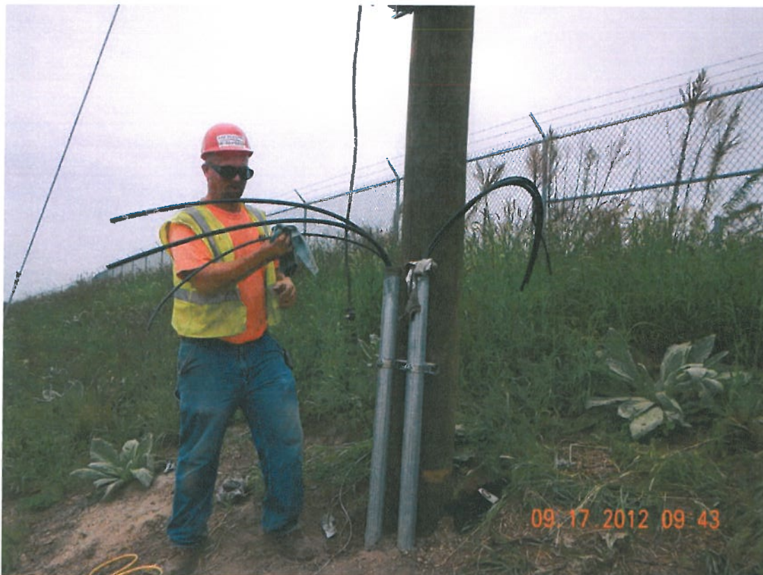
Photograph 2 ▲ - Pulling electric to west pump control panel facing west
