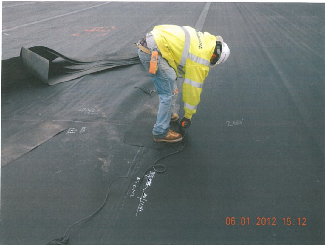
Photograph 11 ▲ - Tacking patch to geomembrane with a lyster facing south
