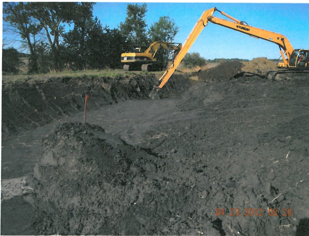
Photograph 2 ▲ - Undercutting wet ash in south embankment facing west
