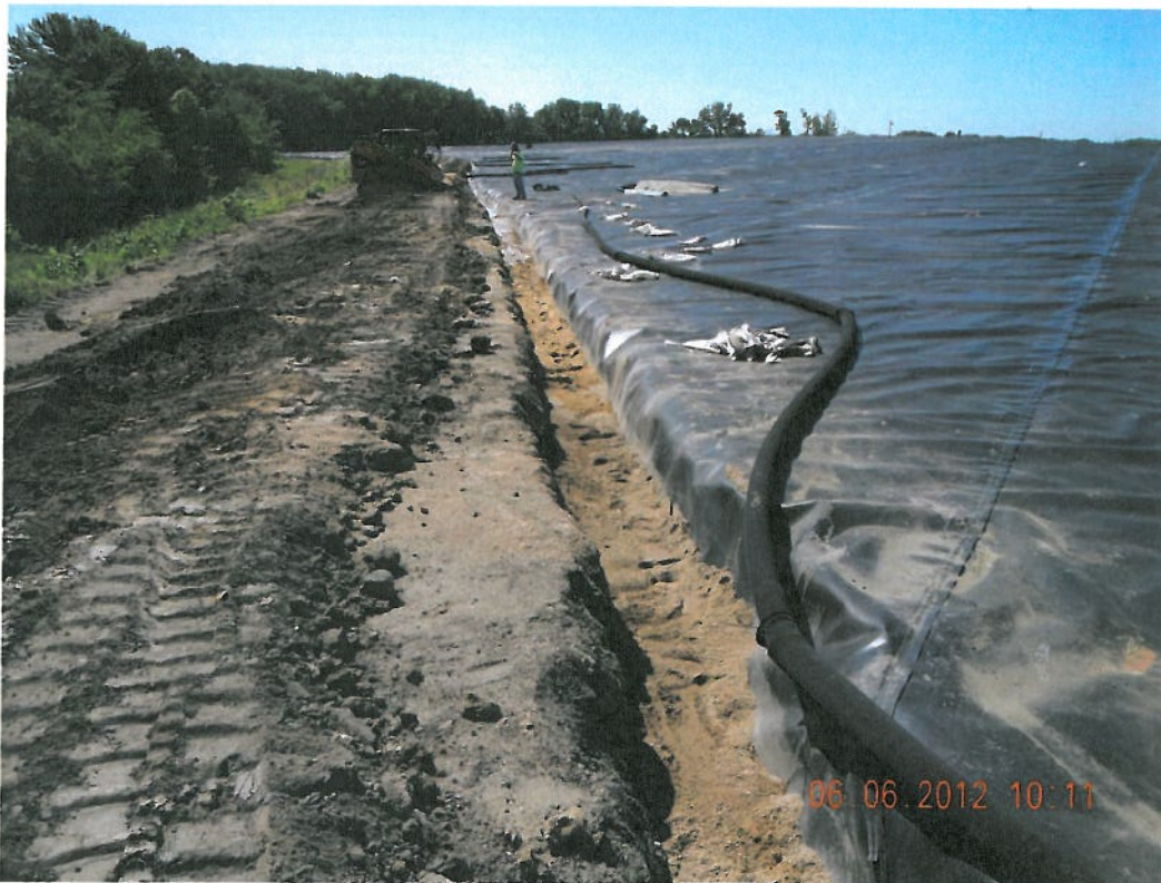
Photograph 6 ▲ - Placing pipe bedding in anchor trench facing southeast
