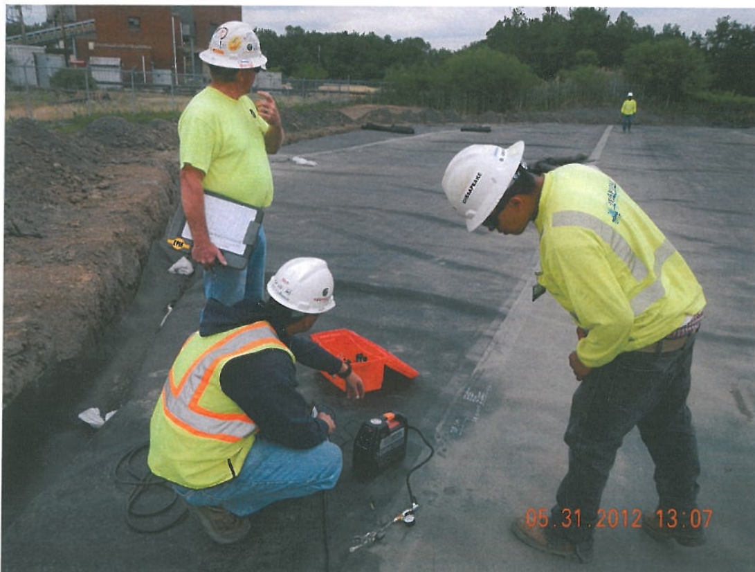
Photograph 6 ▲ - Air testing seam facing north
