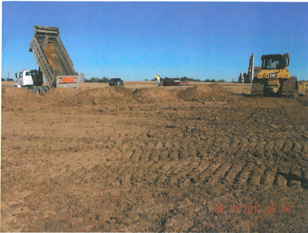
Photograph 3 ▲ - Vegetative layer placement facing northwest
