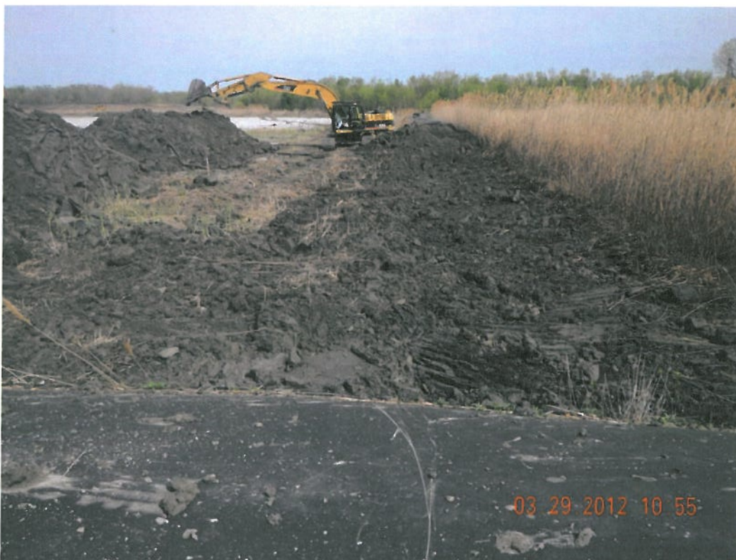
Photograph 8 ▲ - Breaking Geotubes on east end facing northeast
