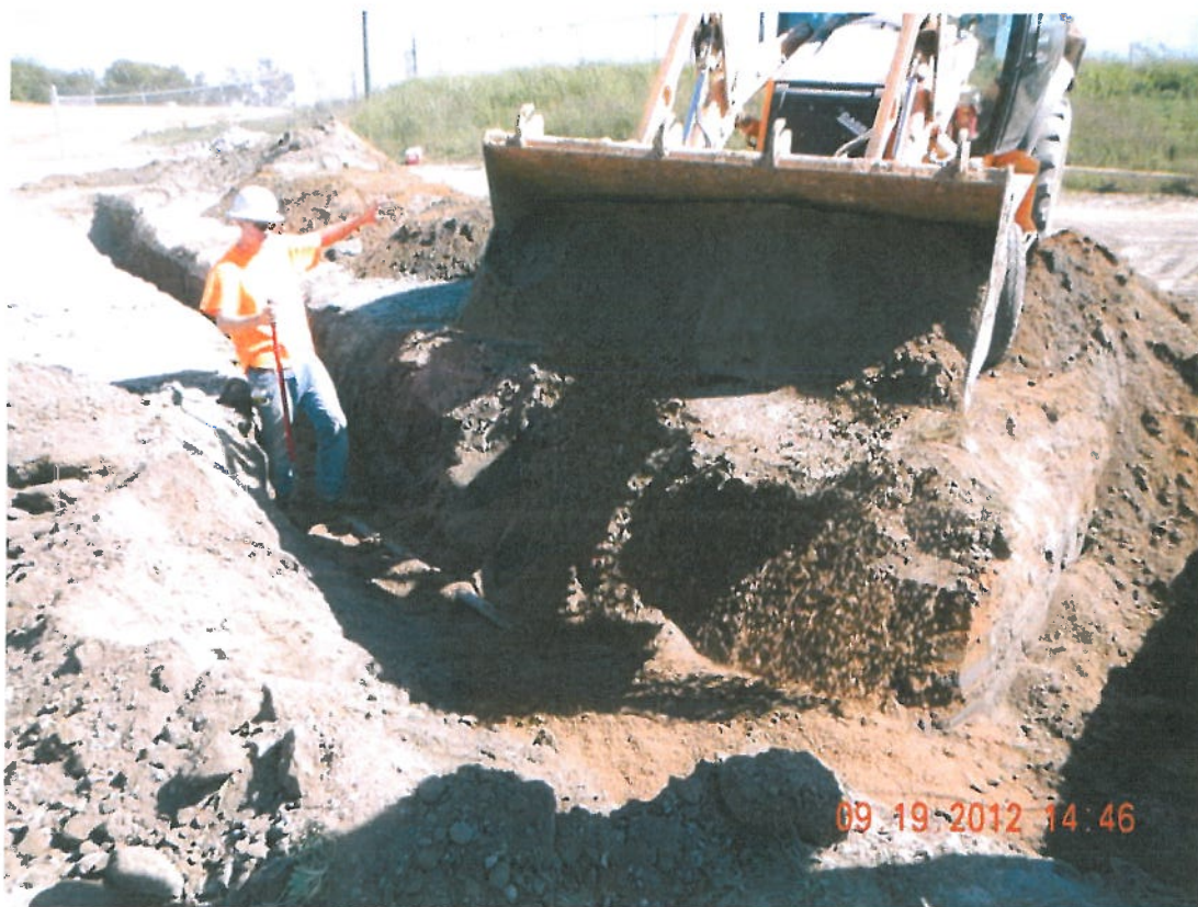
Photograph 7 ▲ - PVC conduit for Ash Pond C electrical feed facing south
