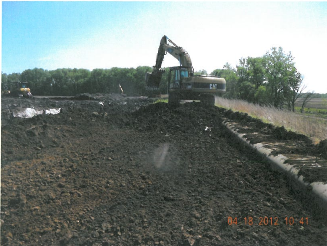
Photograph 7 ▲ - Removing ADS pipe and exposing 18" HDPE drainage pipe facing east
