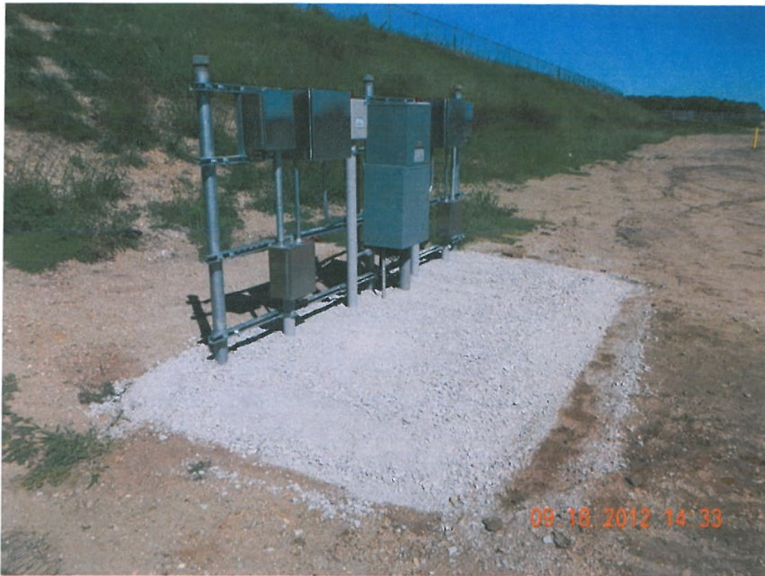
Photograph 5 ▲ - Gravel pad for west pump control panel facing northeast
