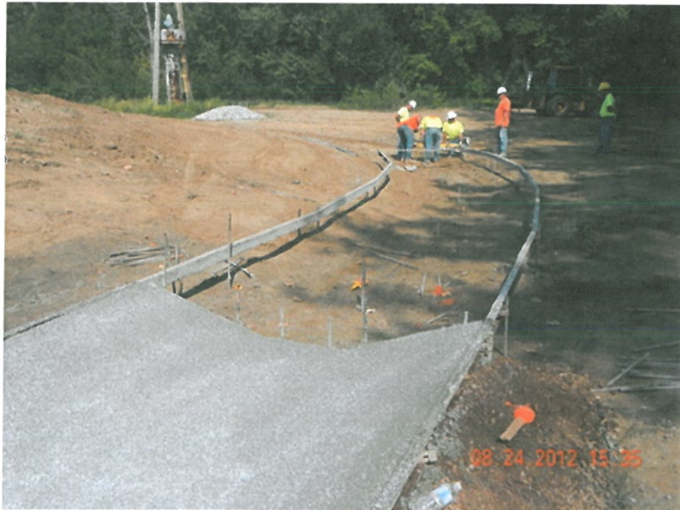
Photograph 11 ▲ - Forming the paved ditch facing east.
