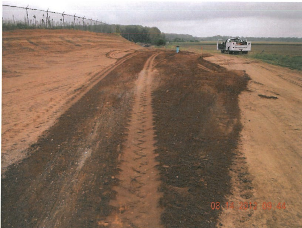
Photograph 4 ▲ - Collector trench backfill facing northeast
