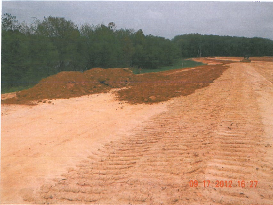
Photograph 3 ▲ - Vegetative layer placement facing east
