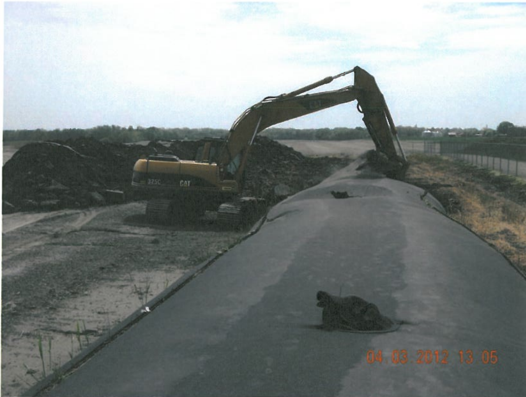
Photograph 5 ▲ - Breaking geotubes on west end of Ash Pond D facing south
