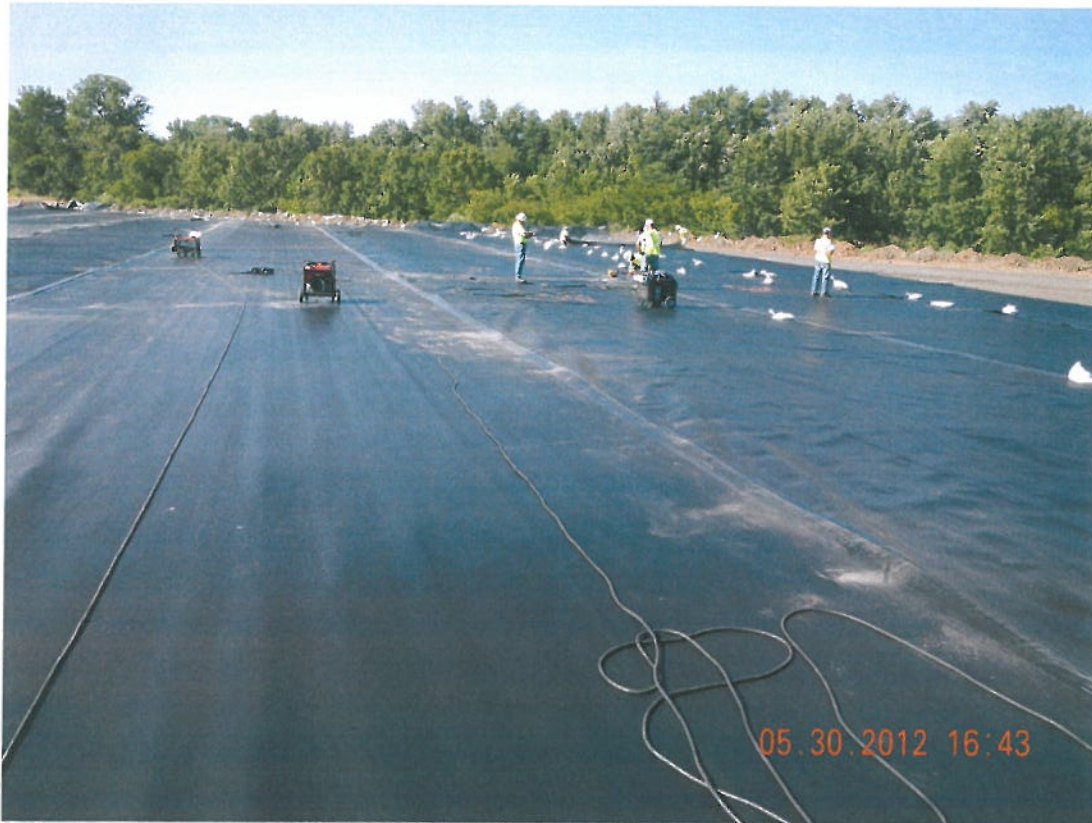
Photograph 5 ▲ - Geomembrane installation facing north
