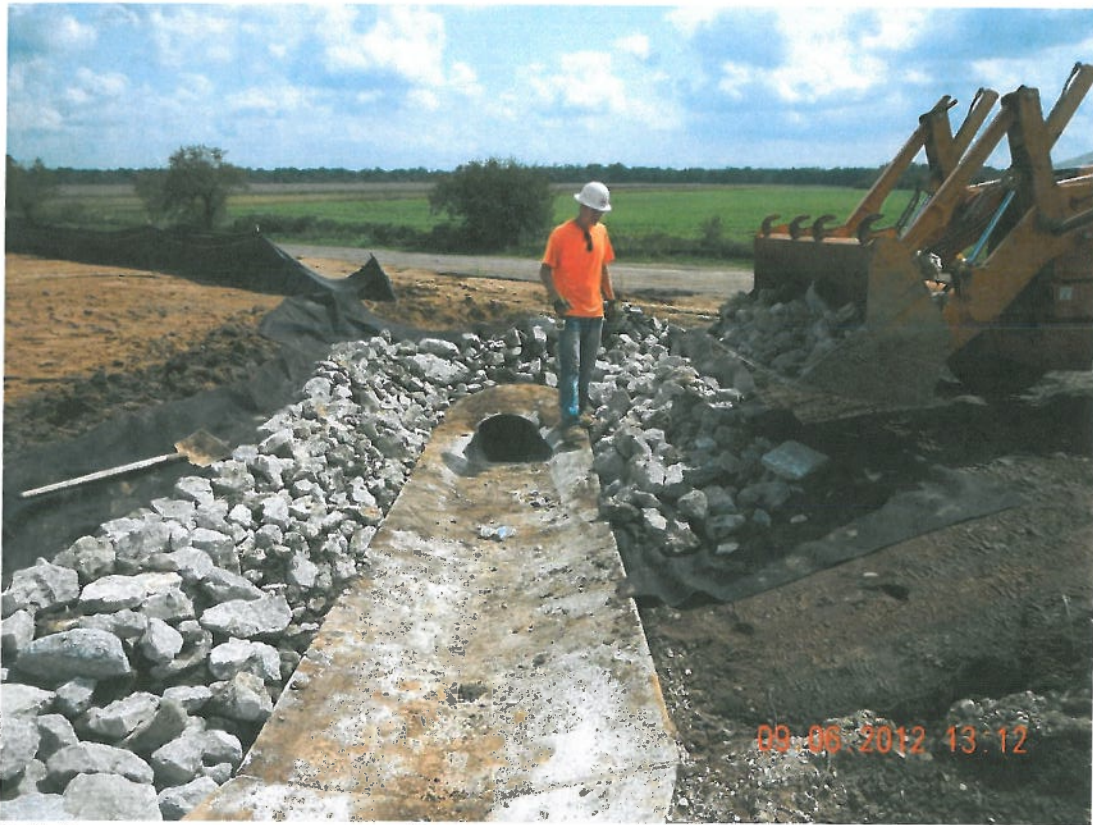
Photograph 7 ▲ - Placing rip rap for paved gutter facing northwest
