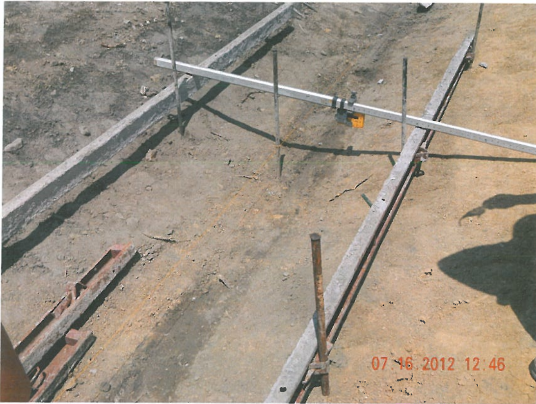
Photograph 3 ▲ - Forming paved gutter facing north
