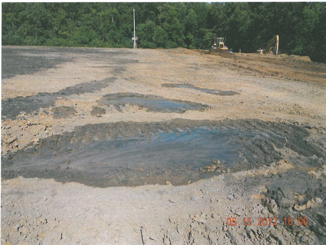
Photograph 8 ▲ - Water seeps in Quadrant D facing east
