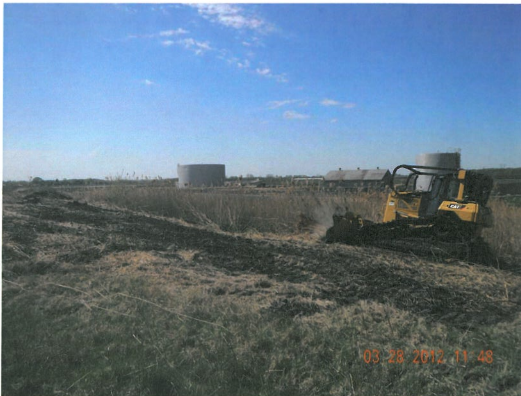
Photograph 4 ▲ - Stripping vegetation in Quadrant A facing west
