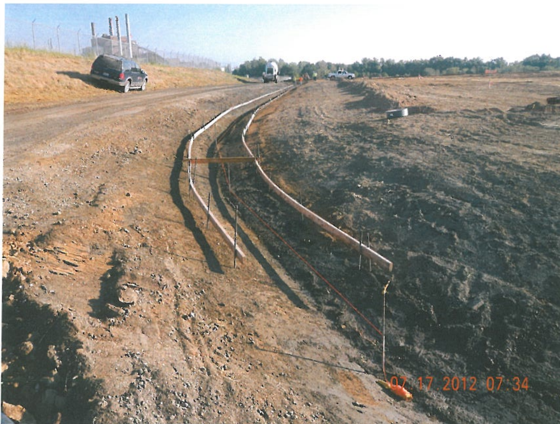
Photograph 6 ▲ - Forming paved gutter facing north
