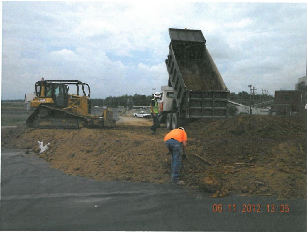
Photograph 1 ▲ - Root removal during clay placement facing west
