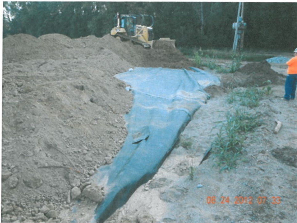
Photograph 9 ▲ - Completing clay placement facing northeast.
