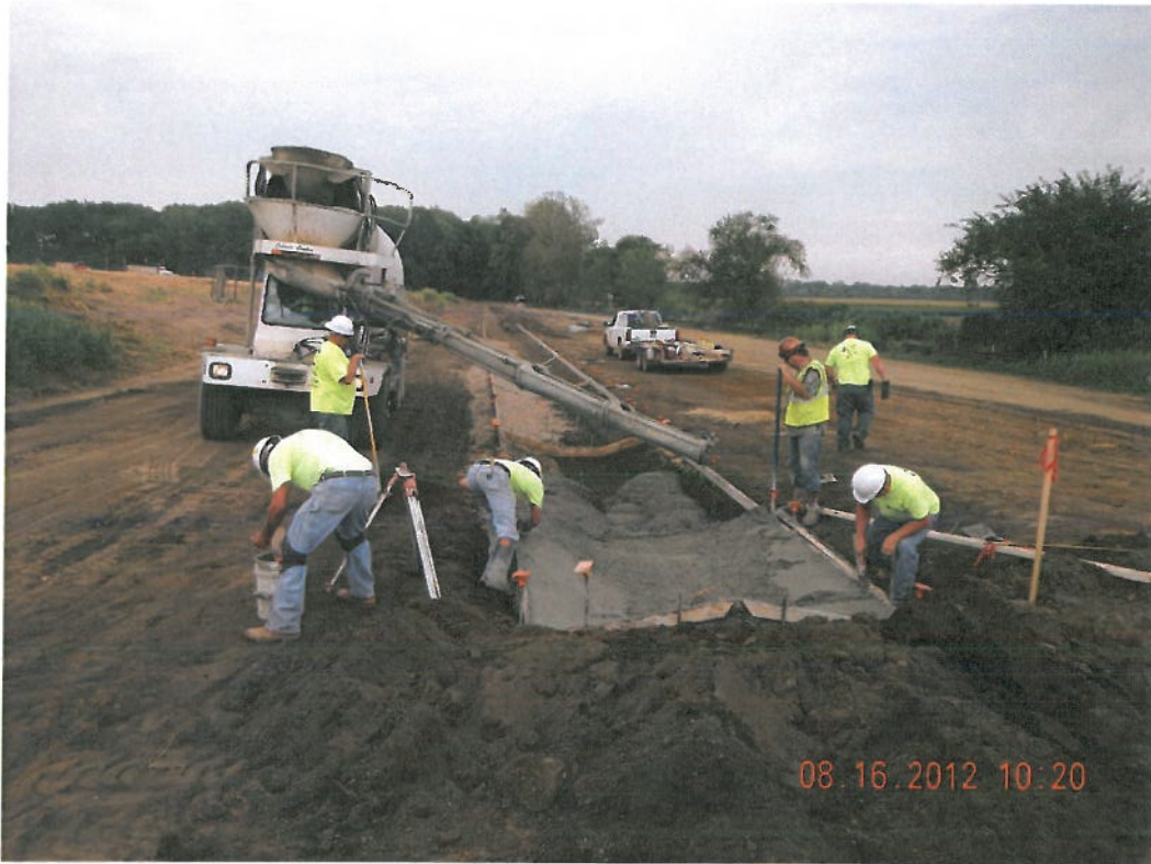
Photograph 9 ▲ - Paved ditch construction facing east
