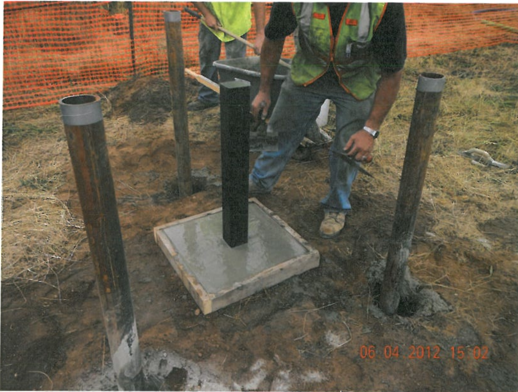
Photograph 5 ▲ - Installing monitoring well MW-2R facing northeast
