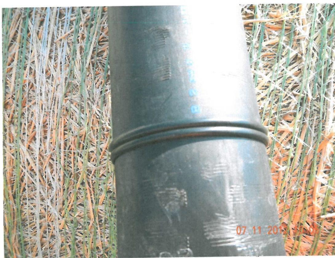
Photograph 8 ▲ - Typical HDPE pipe butt fusion weld facing south
