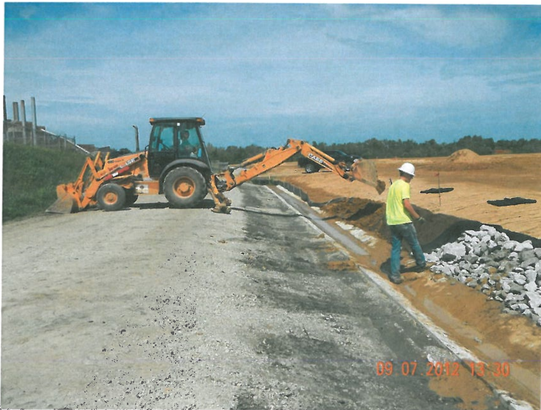
Photograph 8 ▲ - Placing rip rap for paved gutter facing north
