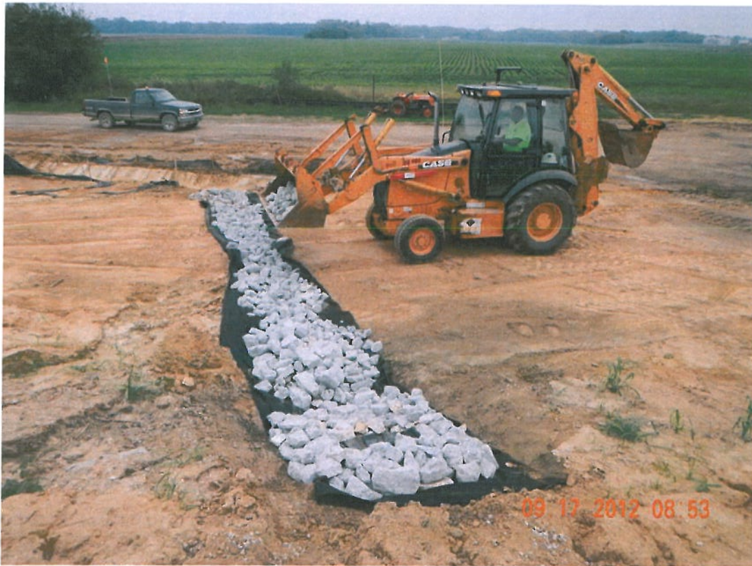
Photograph 1 ▲ - Rock chute for paved gutter culvert facing south
