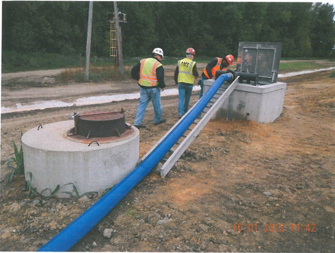
Photograph 3 ▲ - Groundwater collection system pump commissioning facing southeast
