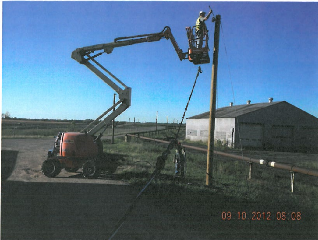
Photograph 1 ▲ - Installing overhead electric lines facing south
