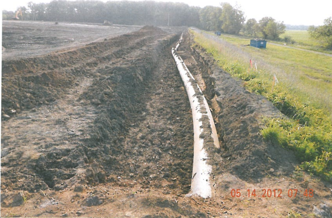
Photograph 1 ▲ - Relocated 18" HDPE pipe facing east
