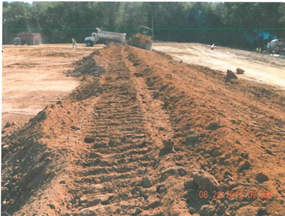
Photograph 10 ▲ - Slope diversion berm construction facing east.
