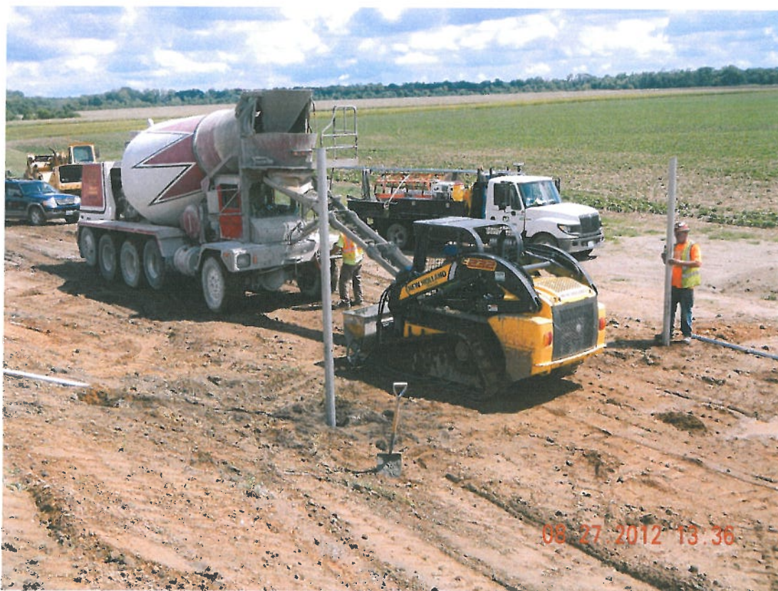
Photograph 2 ▲ - Installing new fence posts facing southeast
