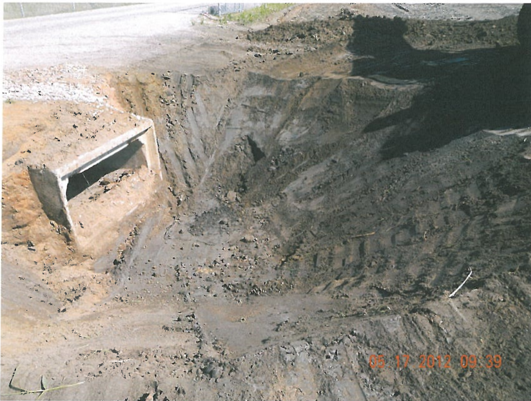
Photograph 11 ▲ - Preparing box culvert pad facing north
