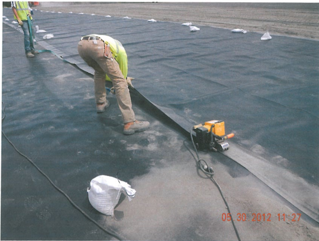
Photograph 3 ▲ - Double wedge seaming facing northeast
