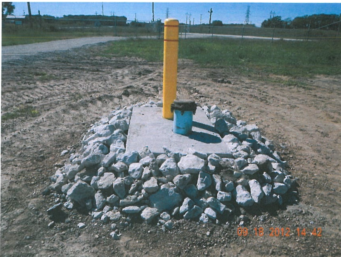
Photograph 6 ▲ - Rip rap around cleanout concrete slabs facing northwest
