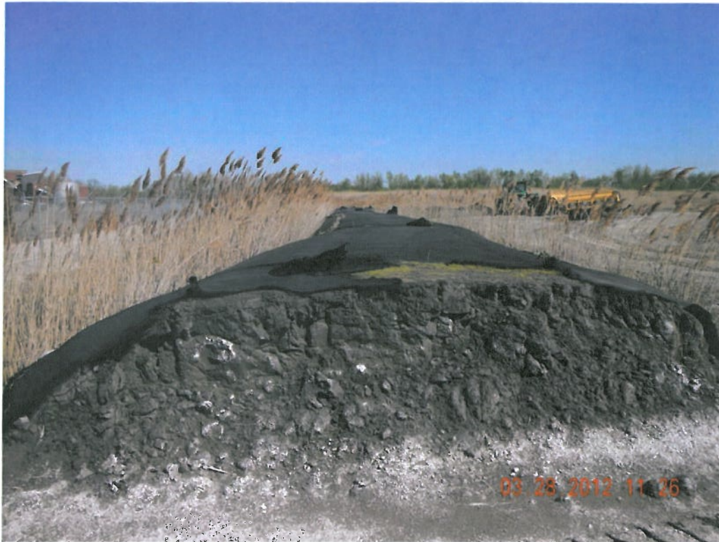
Photograph 3 ▲ - Geotube on west end cut for pond access facing north
