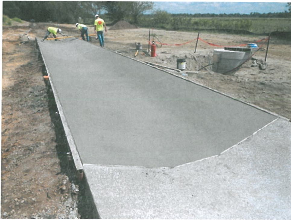
Photograph 3 ▲ - Typical finishing for the paved ditch facing east.
