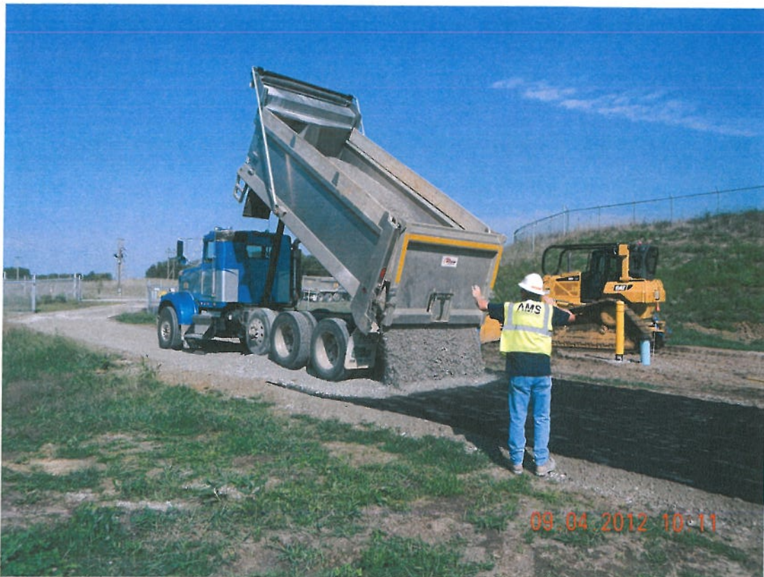
Photograph 4 ▲ - Gravel road surfacing facing northwest
