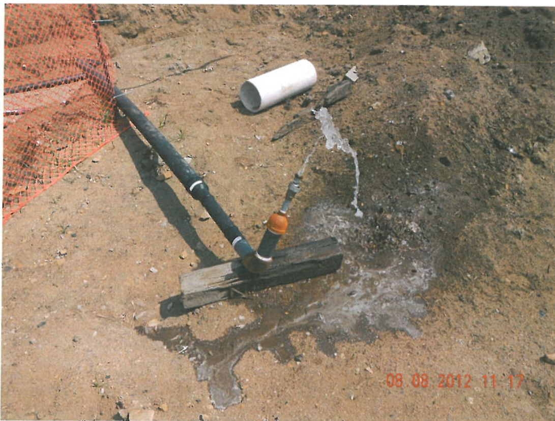
Photograph 6 ▲ - Bleed valve at DS-2 for hydrostatic testing facing northeast
