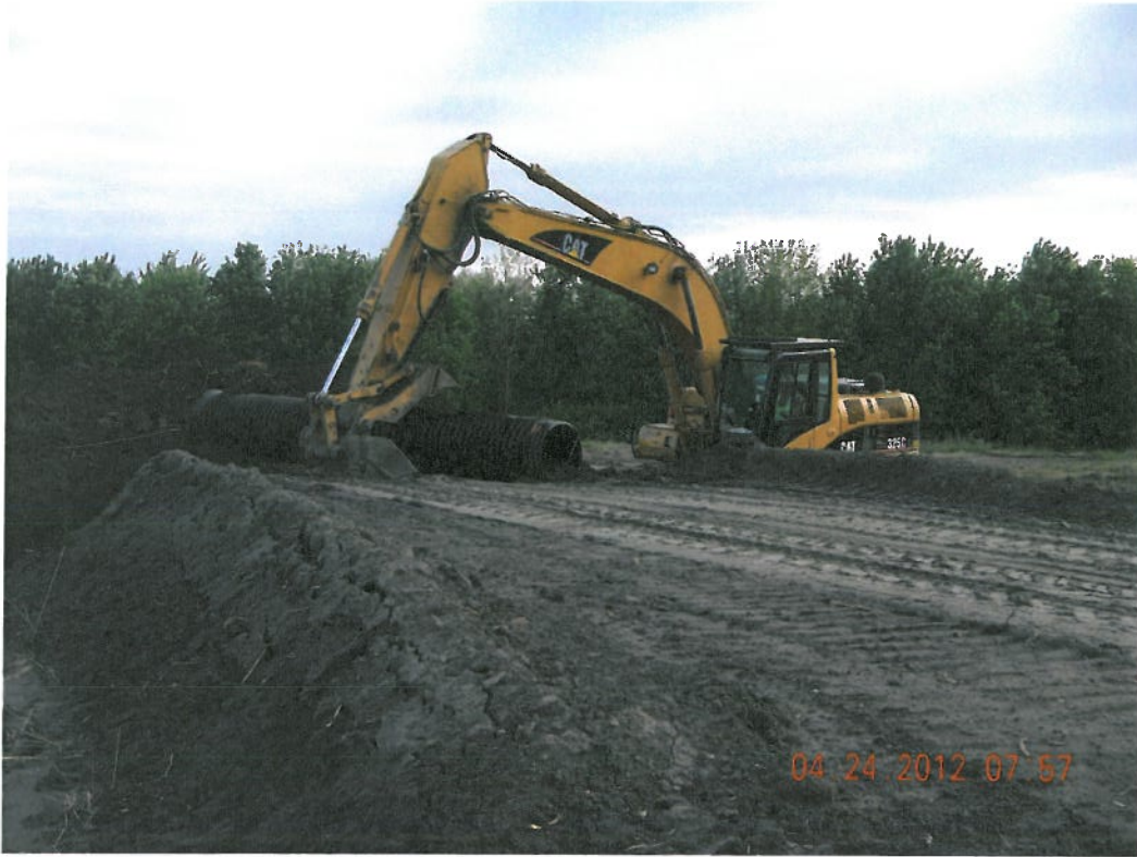
Photograph 3 ▲ - Removing temporary ADS drainage pipe in Quadrant B facing northeast
