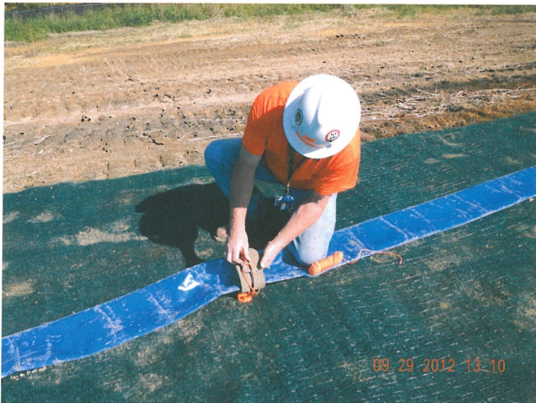
Photograph 10 ▲ - Anchoring flexible hose for temporary discharge into bottom ash pond facing east
