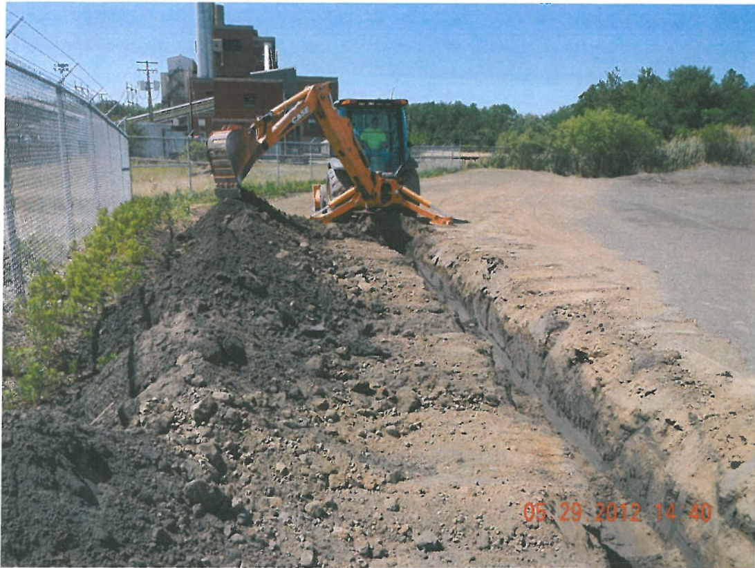
Photograph 1 ▲ - Geomembrane anchor trench facing west
