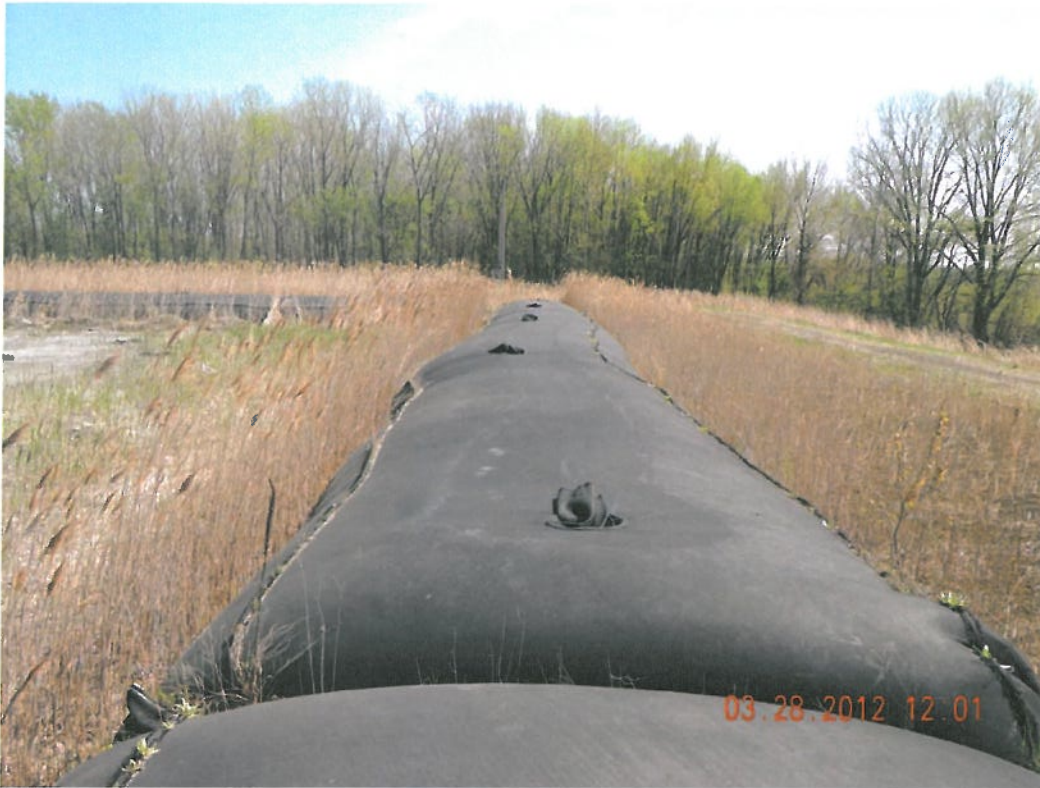
Photograph 5 ▲ - Geotubes on south end facing east
