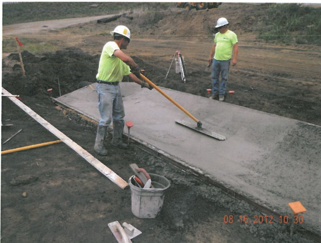
Photograph 10 ▲ - Paved ditch construction facing northwest
