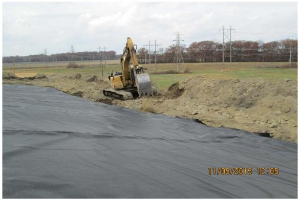
Photograph 12 A - Backfill material placement in the anchor trench.
