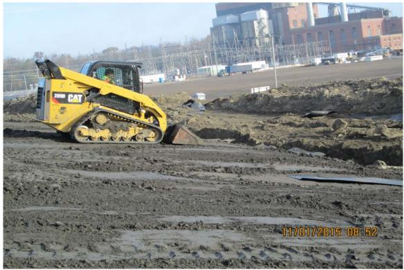
Photograph 1 A - Preparation of surface before HDPE geomembrane installation on the east slope of Ash Pond A, facing north.
