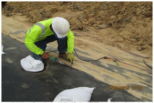
Photograph 14 ^ - Preparing the Ash Pond D slope HDPE geomembrane for the tie-in to the existing Ash Pond D HDPE geomembrane, looking northeast.
