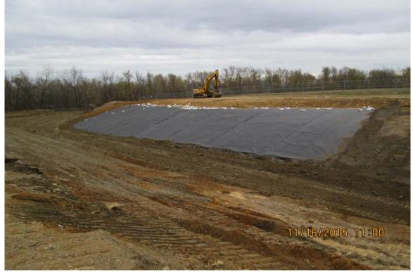
Photograph 3 A - View of Ash Pond D protective cover material replaced over Ash Pond D HDPE geomembrane, looking northeast.
