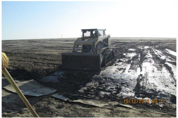
Photograph 2 A - View of cleaning the edges of Ash Pond A, looking east.
