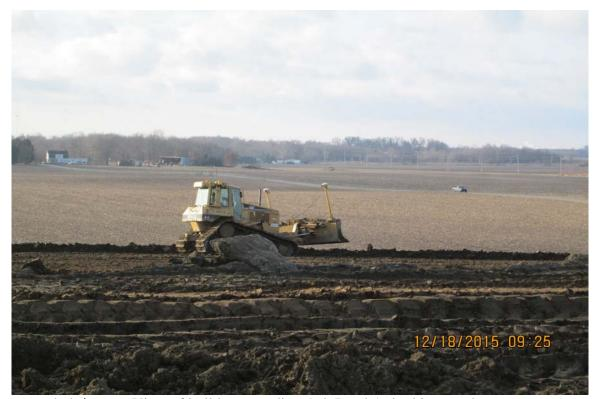
Photograph 4 A - View of bulldozer grading Ash Pond A, looking south.
