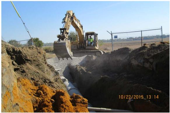
Photograph 13 A - View of placing gravel pipe bedding over the concrete pipe at the Ash Pond B outfall.
