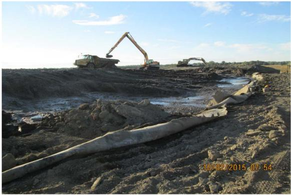
Photograph 19 A - View of excavators removing ash and placing dry soil at the western corner of Ash Pond A.
