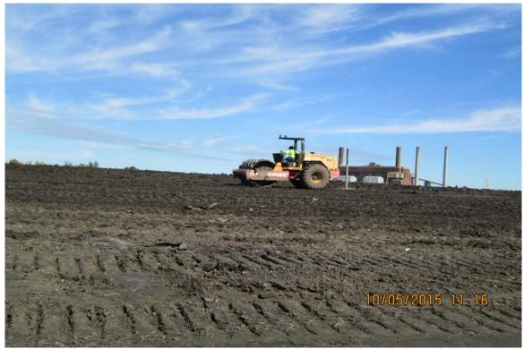
Photograph 3 A - View of sheepsfoot roller compacting wet ash to promote drying.
