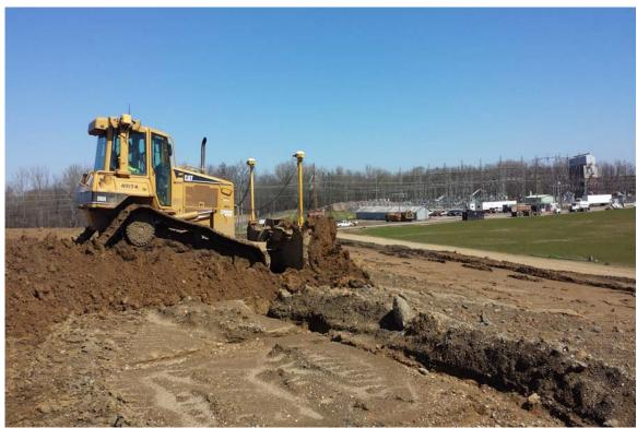
Photograph 7 A - View of placement of soil in rills to cover exposed liner on Ash Pond A, looking north.
