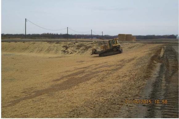
Photograph 1 ^ - View of tracking the slopes of Ash Pond C in preparation for anticipated rain, looking south.
