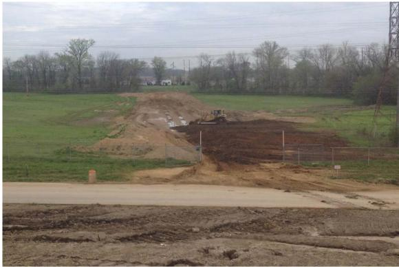
Photograph 9 A - View from the top of Ash Pond A of regrading activities associated with the borrow field haul road, looking northwest.
