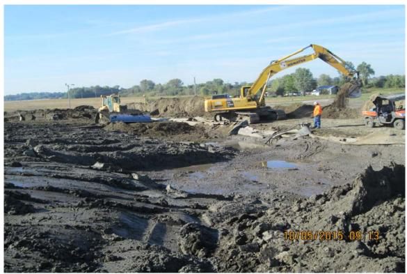
Photograph 1 A - View of placing dry soil over wet ash at the western corner of Ash Pond A.
