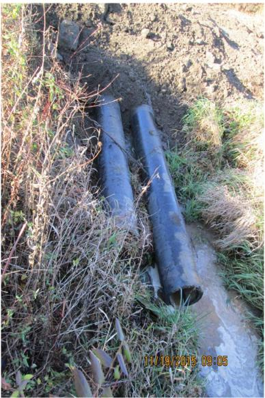
Photograph 6 A - View of culverts installed under the ditch crossing on the borrow field road, looking west.
