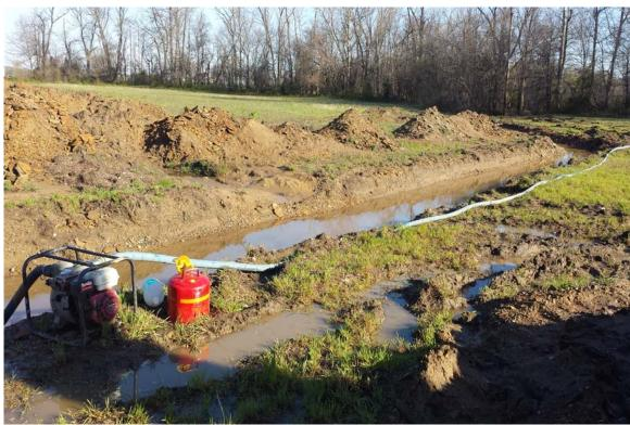
Photograph 1 A - View of dewatering the haul road to the borrow field on April 12, 2016, looking northeast.
