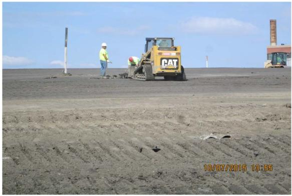
Photograph 7 A - View of deleterious material removal from the surface of Ash Pond A, looking north.
