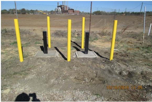
Photograph 18 A - View of completed Monitoring Wells MW-22D and MW-22S.
