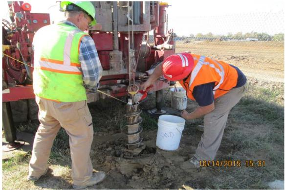
Photograph 8 ^ - View of placing sand as filter pack in the Monitoring Well MW-22D annular space.
