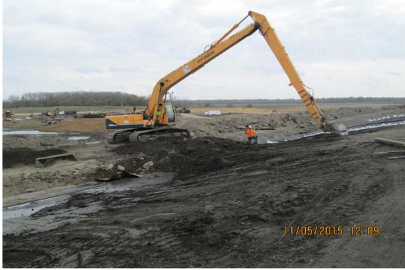
Photograph 13 A - Excavating the access ramp to Ash Pond A.
