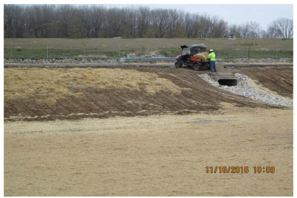
Photograph 2 A - View of placing straw over areas where it had been blown away by winds, looking southeast.
