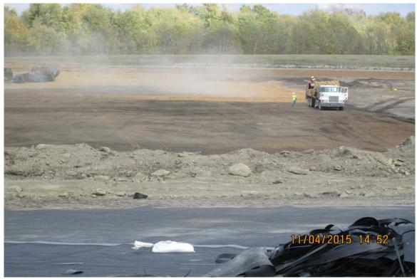
Photograph 10 A - Spreading straw over the seeded Coal Yard, looking northeast.
