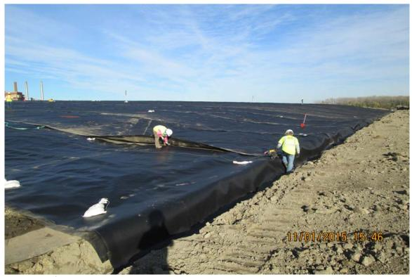
Photograph 7 A - Fusion welding HDPE geomembrane on Ash Pond A, looking northeast.
