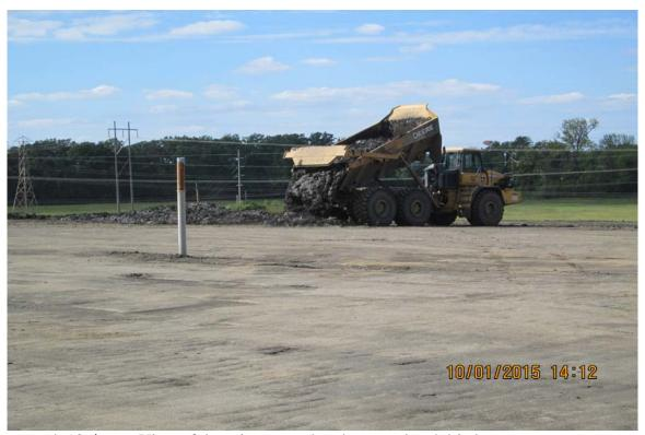
Photograph 18 ▲ - View of dumping wet ash to be spread and dried.
