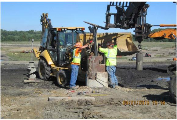
Photograph 4 A - View of gravel placement in the annular space of the vents on Ash Pond A.
