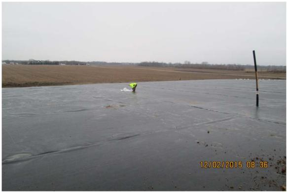
Photograph 12 ^ - View of Ash Pond A sandbag removal prior to protective cover placement, looking southeast.
