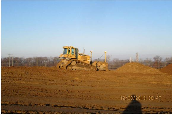
Photograph 17 A - View of Ash Pond A protective cover placement, looking west.
