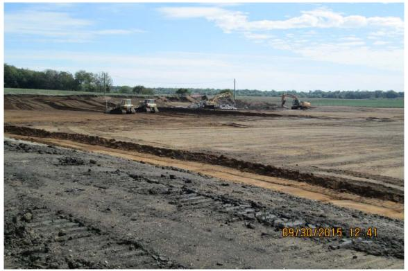
Photograph 14 A - View of grading and structure demolition activity in Ash Pond B.
