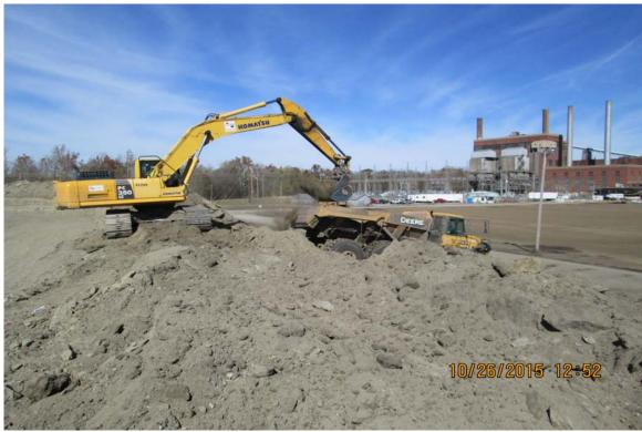
Photograph 3 - Loading out large cementitious material from the Ash Pond east levee, looking north.
