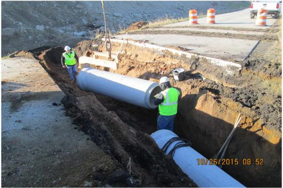
Photograph 1 A - Placing RCP culvert under the main access road near the northeast corner of Ash Pond A, looking south.
