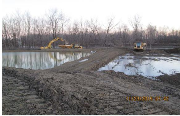
Photograph 1 A - View of Bottom Ash Pond levee excavation for use as protective cover, looking north.
