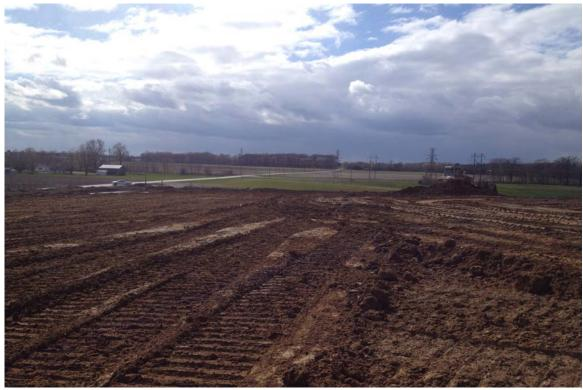
Photograph 13 A - View of the cover soil on Ash Pond A, looking east.
