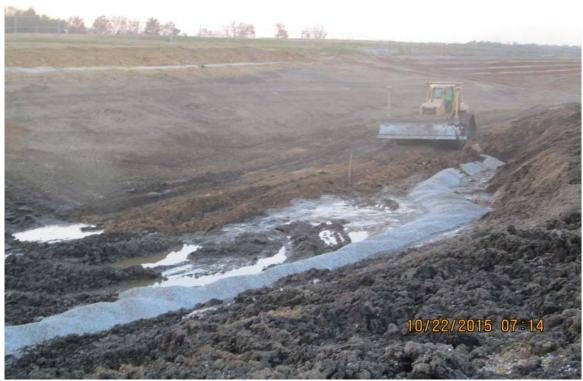
Photograph 11 ^ - View of placing dry soil over wet soil at the Bottom Ash Pond anchor trench.
