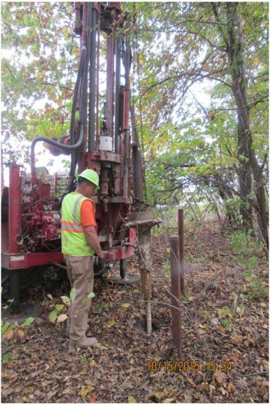
Photograph 15 A - View of Monitoring Well MW-1 abandonment.
