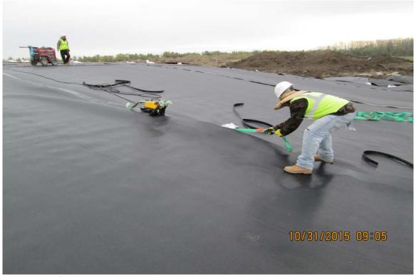
Photograph 17 ^ - View of fusion-welding two HDPE geomembrane panels on Ash Pond A, looking west.
