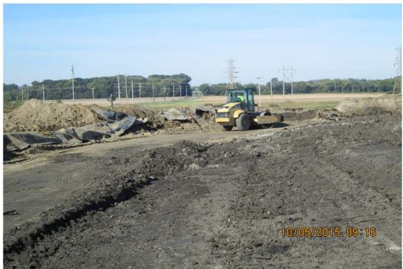
Photograph 2 A - View of smooth drum roller compacting dry soil over wet ash at the western corner of Ash Pond A.
