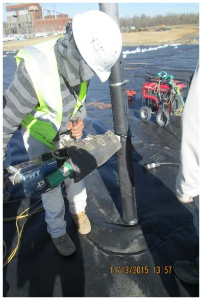
Photograph 3 A - View of extrusion welding boots on a vent pipe in ash Pond A with a wire in place for spark testing.
