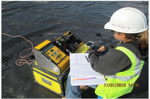
Photograph 6 A - Trial fusion weld tests on Ash Pond A.
