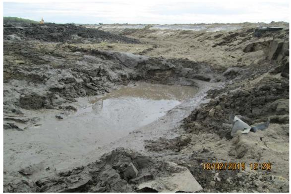
Photograph 22 A - View of saturated ash level at the western corner of Ash Pond A.
