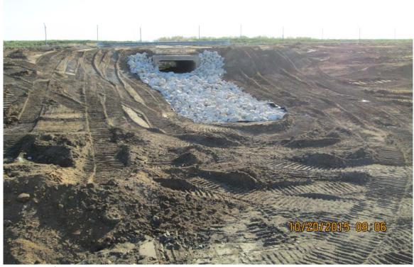
Photograph 4 A - View of rip-rap apron at culvert in the east levee of Ash Pond C.
