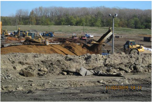
Photograph 8 A - Placing excess material from Ash Pond B into a stockpile in the south corner of the Coal Yard, looking west.
