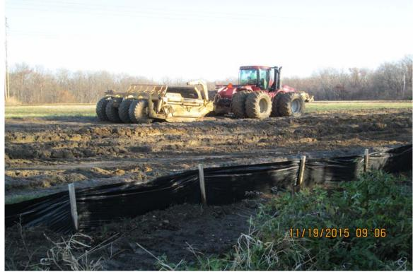
Photograph 7 A - View of scraping topsoil at the borrow field, looking north.
