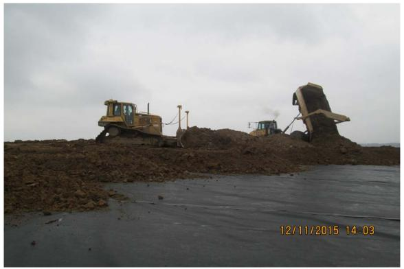
Photograph 6 ▲ - View of Ash Pond A protective cover placement, looking southeast.
