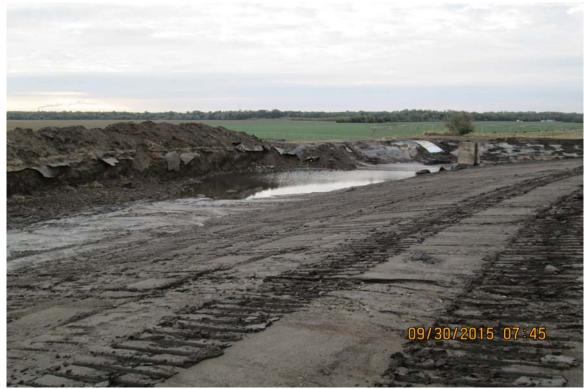
Photograph 9 A - View of southeast corner of Ash Pond A after rain, showing ponded water.
