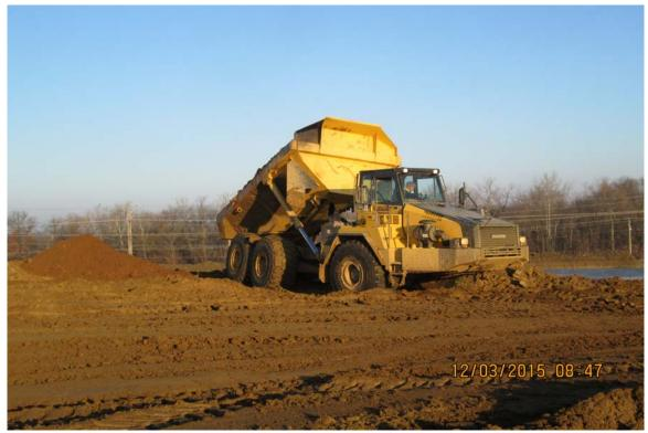
Photograph 18 A - View of Ash Pond A protective cover placement, looking west.
