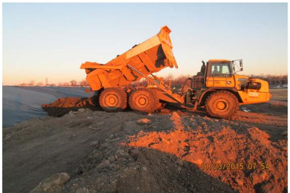
Photograph 2 A - View of protective cover placement on Ash Pond A, looking west.
