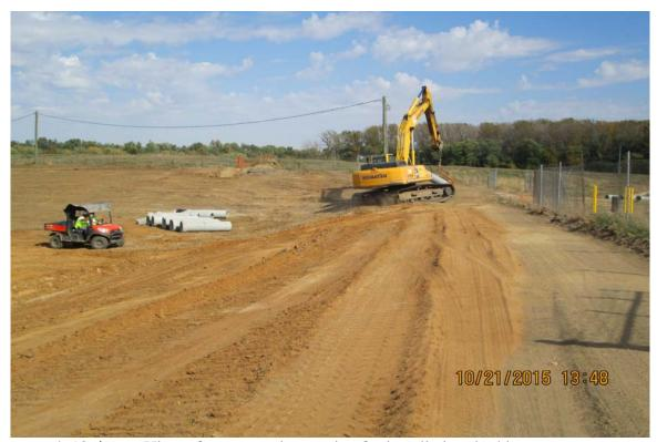
Photograph 10 A - View of concrete pipe staging for installation, looking east.
