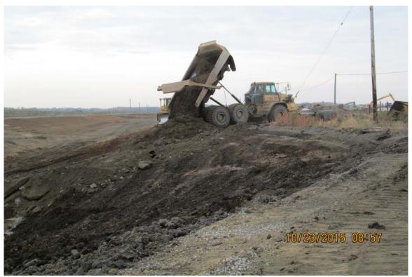
Photograph 14 ^ - View of placing material with cementitious material blocks at the Bottom Ash Pond, looking south.
