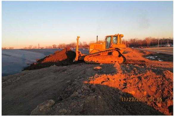
Photograph 3 A - View of protective cover placement on Ash Pond A, looking west.
