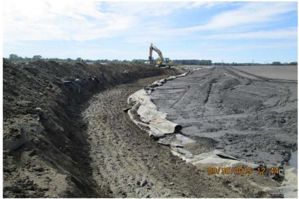
Photograph 15 A - View of liner demolition and anchor trench construction at the southeast corner of Ash Pond A.
