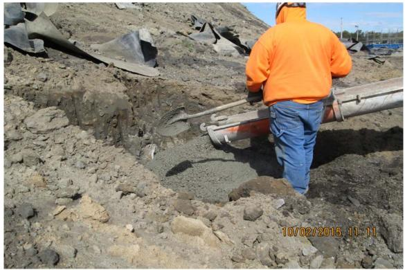
Photograph 21 A - View of concrete placement to plug the Ash Pond A outfall pipe.
