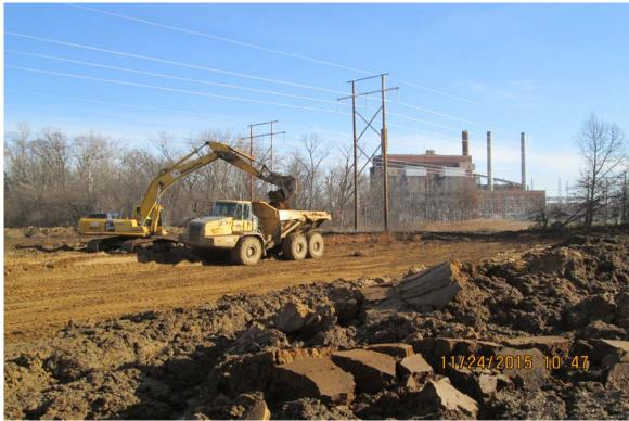
Photograph 5 ^ - View of excavating borrow field material for use as protective cover, looking northeast.
