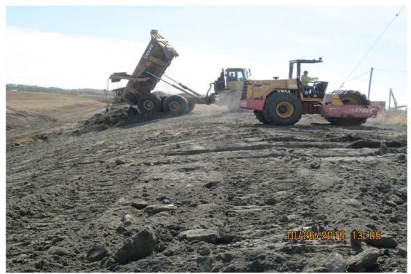
Photograph 4 ^ - View of placing, grading, and compacting material from the Ash Pond Levee at the southwest corner of the Bottom Ash Pond, looking south.
