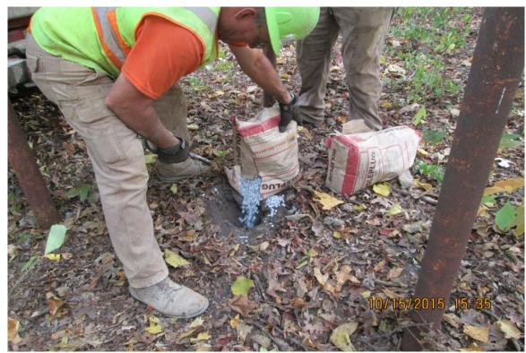
Photograph 16 A - View of Monitoring Well MW-1 abandonment backfill.
