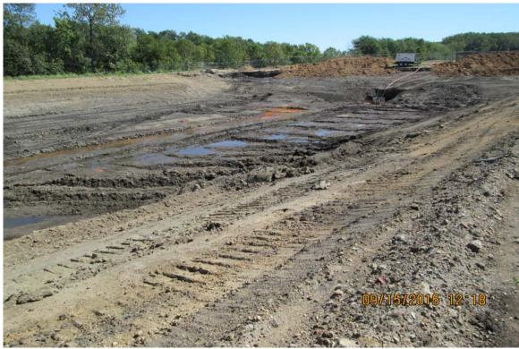
Photograph 1 A - View of the north portion of the Bottom Ash Pond looking southeast, showing groundwater leaching and subsequent dewatering.
