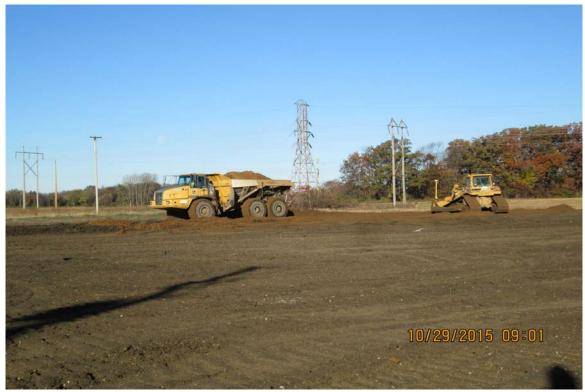
Photograph 11 ^ - View of placing and grading material at the former CCW stockpile outside the gate, looking north.
