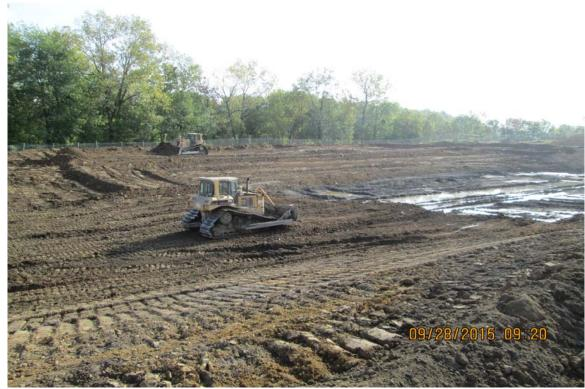
Photograph 1 A - View of Bottom Ash Pond grading, looking east.
