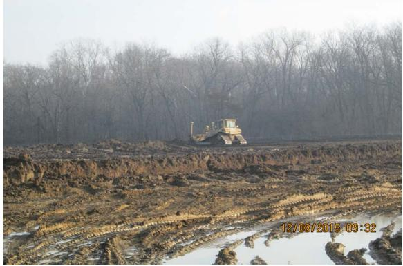
Photograph 3 A - View of topsoil removal at the borrow field, looking northeast.
