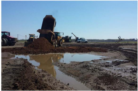
Photograph 5 A - View of sandy soil placement as backfill for removed soil at the former fuel tank location, looking south.
