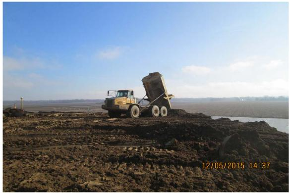
Photograph 25 A - View of Ash Pond A protective cover placement, looking south.
