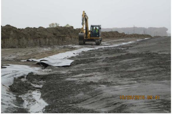
Photograph 7 ^ - View of excavator moving soil to allow drainage of Ash Pond A looking west, showing wet conditions on Ash Pond A.
