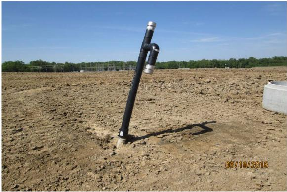
Photograph 12 A - View of typical Ash Pond A vent well, prior to placement of protective barrier.
