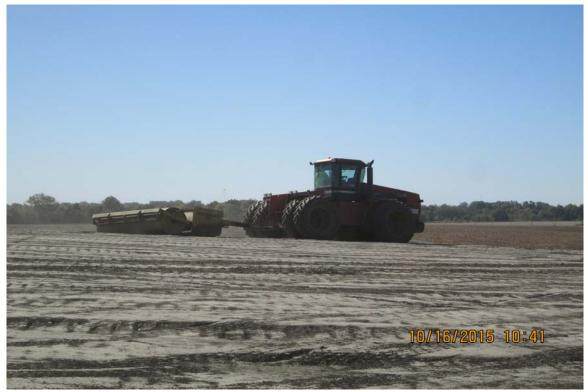
Photograph 17 A - View of smooth drag roller on Ash Pond A, looking west.
