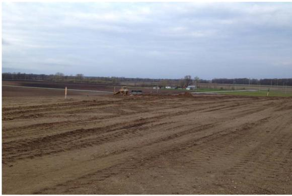
Photograph 11 A - View of cover soil placement on Ash Pond A, looking southwest.
