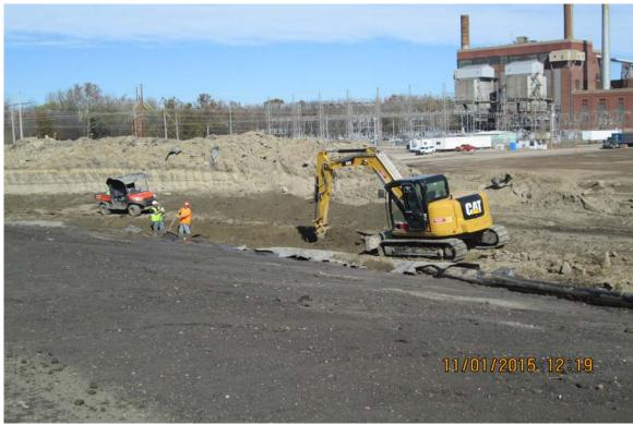
Photograph 3 A - Anchor trench excavation at the northeast corner of Ash Pond A, looking north.
