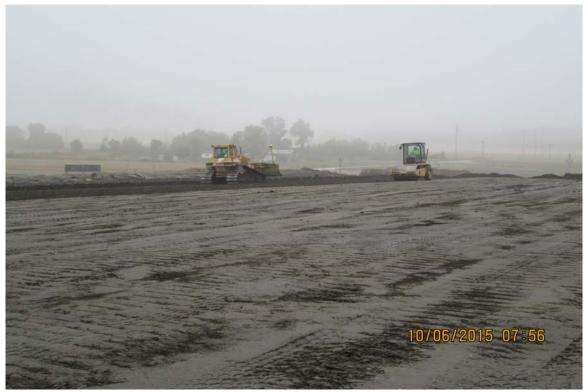
Photograph 6 A - View of grading and smooth drum rolling on Ash Pond A, looking west.
