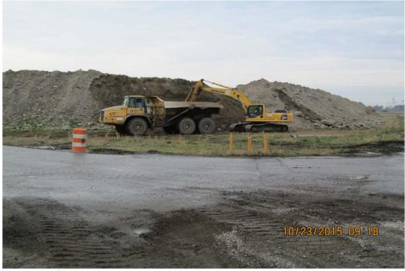
Photograph 15 ^ - View of loading material with cementitious material blocks at Ash Pond A, looking south.
