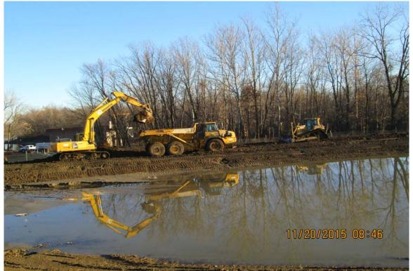
Photograph 8 ^ - View of loading out Bottom Ash Pond levee material for use as protective cover, looking north.
