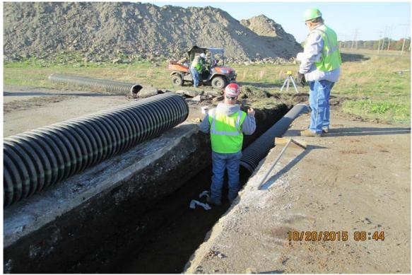
Photograph 1 A - View of culvert placement under the road between Ash Pond A and the Coal Yard.
