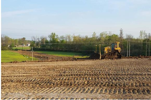
Photograph 1 A - View of topsoil grading on Ash Pond A, looking north.
