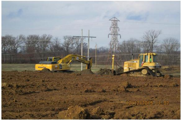
Photograph 7 - View of Ash Pond A levee material placement and incorporation, looking west.
