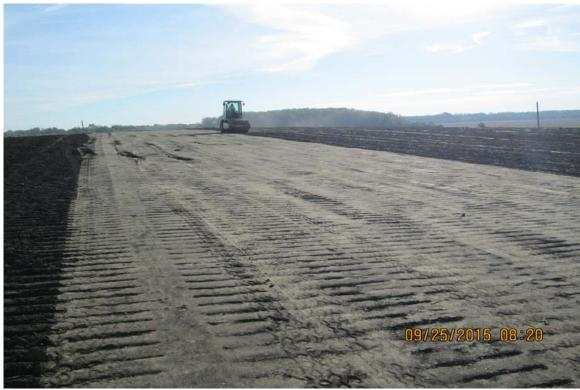
Photograph 18 ^ - View of a smooth-drum roller compacting material on Ash Pond A, looking northeast.
