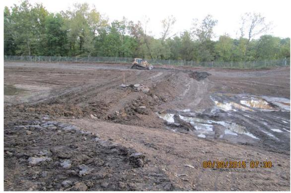
Photograph 7 A - View of the siltation levee at the Bottom Ash Pond nearing completion.
