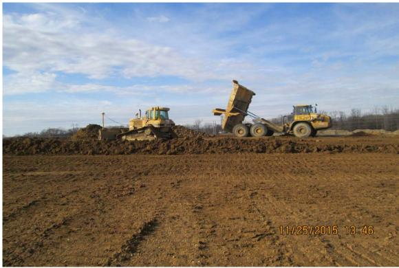
Photograph 9 A - View of placing and grading protective cover on Ash Pond A, looking west.
