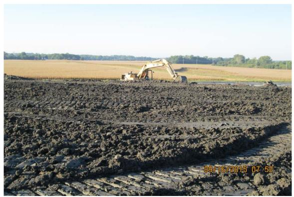
Photograph 12 A - View of an excavator moving material to promote drying of wet material on Ash Pond A, looking southwest.
