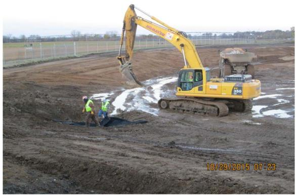
Photograph 9 ^ - View of installation of filter fabric and rip-rap at the RCP inlet at the southeast corner of Ash Pond B.
