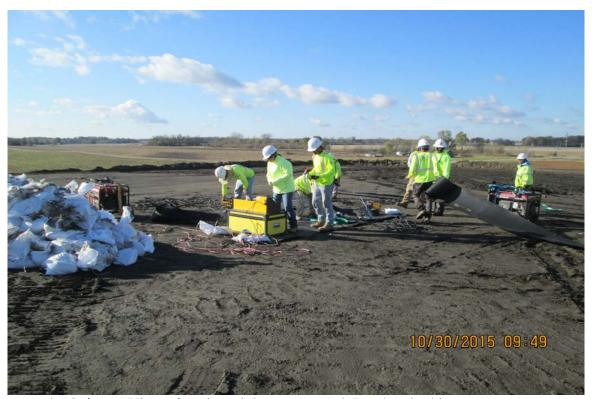
Photograph 12 A - View of testing trial seams on Ash Pond A, looking west.
