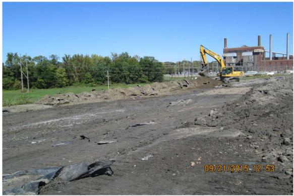
Photograph 3 A - View of anchor trench excavation at Ash Pond A, northwest embankment.
