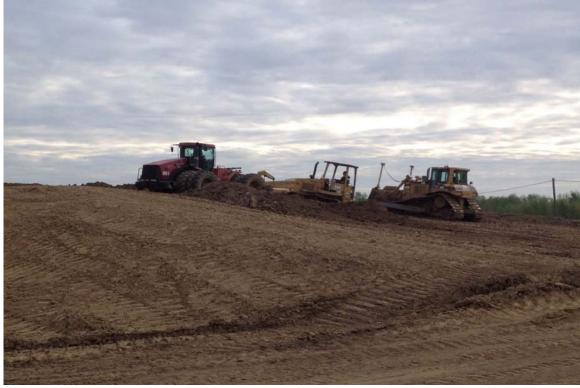
Photograph 8 ^ - View of tractor with elevating pan conducting soil moving activities at the topsoil staging location, looking north.
