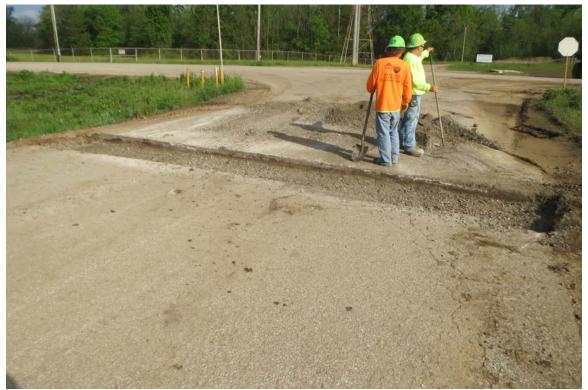
Photograph 6 ^ - View of roadway surface, prepared for concrete replacement on the northeast side of Ash Pond A.
