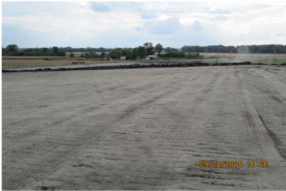
Photograph 5 A - View of the western side of Ash Pond A, looking west, showing the smooth-rolled top of Ash Pond A and the wet ash in the western corner of Ash Pond A.
