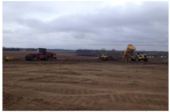
Photograph 12 A - View of cover soil placement on Ash Pond A, looking southeast.
