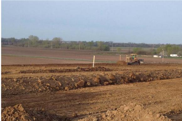
Photograph 7 A - View of surface shaping prior to placement of topsoil in the southern portion of Ash Pond A, looking south.
