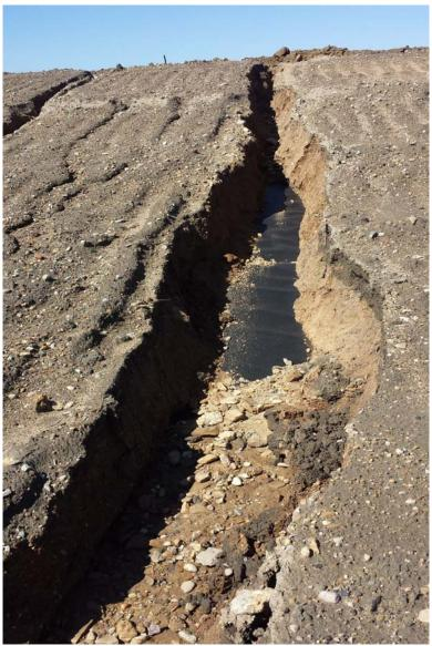
Photograph 6 A - View of typical exposed liner at a rill on Ash Pond A, Looking west. (Observed at two locations.)
