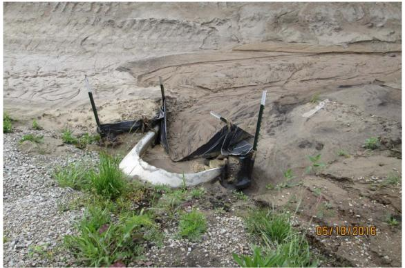
Photograph 2 A - View of a silt fence around the culvert on the south side of the north access road, looking southeast.
