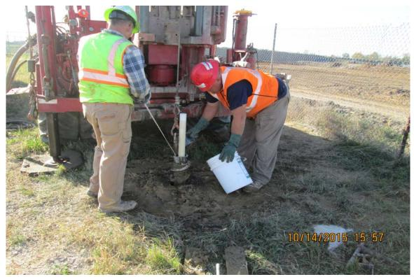
Photograph 9 A - View of placing bentonite seal in Monitoring Well MW-22D annular space.
