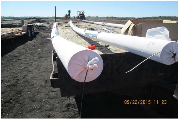
Photograph 8 A - View of the 4-inch HDPE vent pipes enclosed in socks with centralizers for Ash Pond A.
