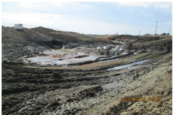
Photograph 9 ^ - View of perforated pipe installed to control seepage in the Bottom Ash Pond, looking south.
