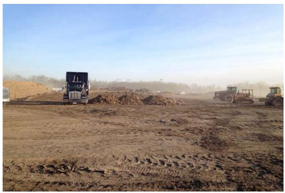
Photograph 2 A - View of topsoil staging activities on the southern portion of the coal yard, looking north.
