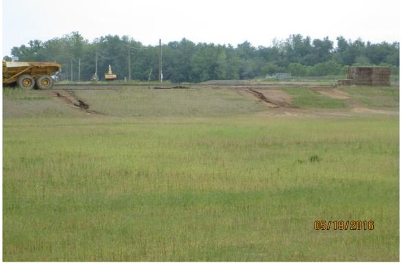
Photograph 5 A - View of Ash Pond B and erosion on the northern slope, looking north-northeast.
