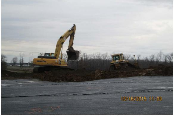
Photograph 2 A - View of folding and grading Ash Pond A levee material on Ash Pond A, looking west.
