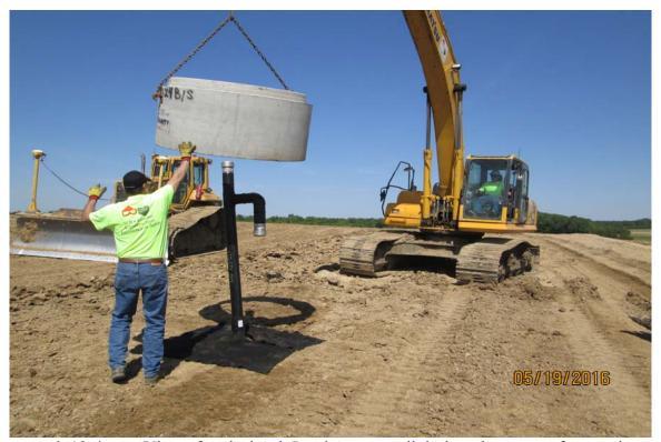
Photograph 13 A - View of typical Ash Pond A vent well during placement of protective barrier.
