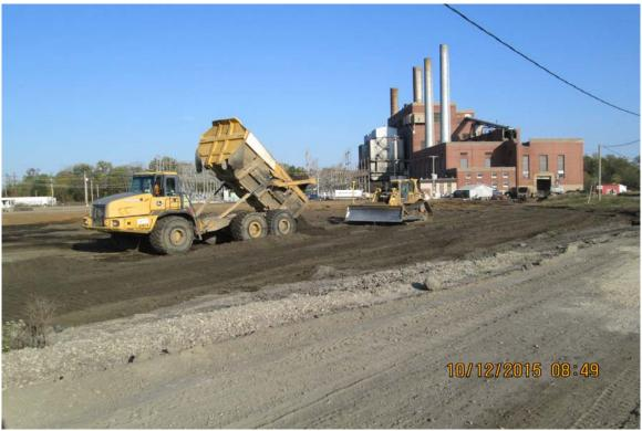
Photograph 1 A - View of placing and grading material at the Coal Yard, looking northwest.
