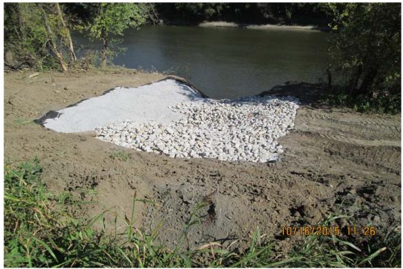
Photograph 20 A - View of outfall construction showing filter fabric, gravel liner, and rip rap.
