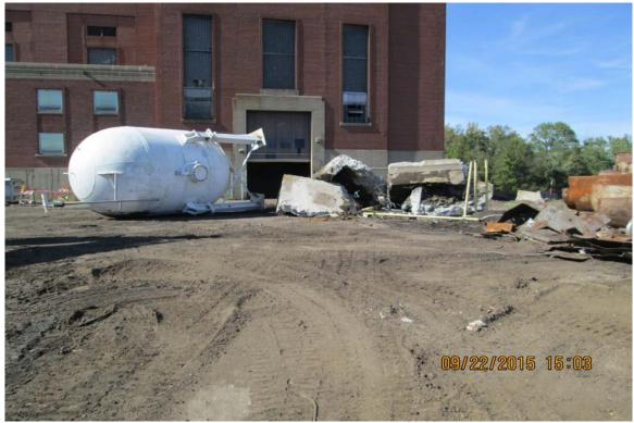
Photograph 12 A - View of hydrogen tank and foundation demolition at the northwest corner of the Bottom Ash Pond.
