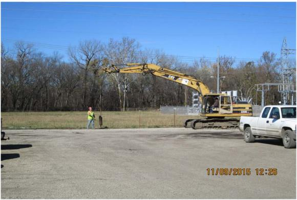
Photograph 1 ^ - View of excavator removing fencing around the parking area on site, looking north.
