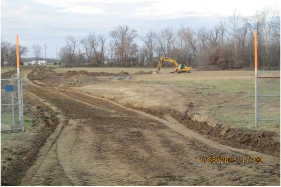
Photograph 10 A - View of excavating a drainage sump for the haul road in anticipation of rain.
