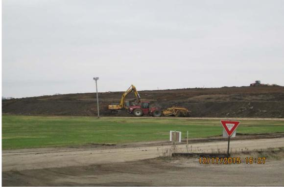
Photograph 3 ^ - View of Ash Pond A north ramp removal for placement as protective cover, looking south.
