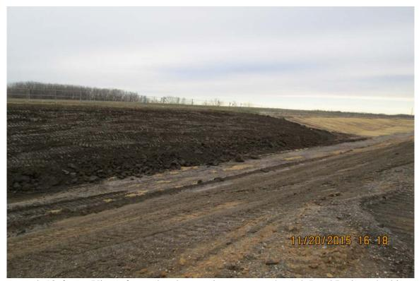
Photograph 10 ^ - View of completed protective cover on the Ash Pond D slope, looking southwest.
