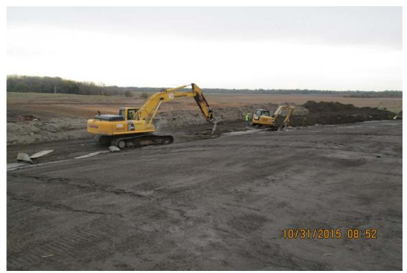
Photograph 16 ^ - View of anchor trench excavation at the east levee of Ash Pond A, looking east.
