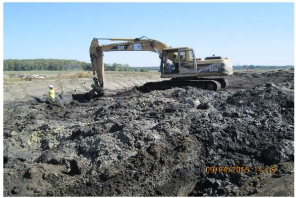
Photograph 16 ^ - View of wet ash drying activities at the northwest corner of Ash Pond A, looking east.
