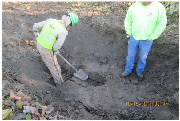
Photograph 13 A - View of hand-exposing power lines at the outfall location.
