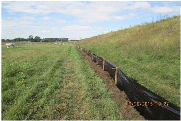
Photograph 13 A - View of silt fence installed south of Ash Pond A.
