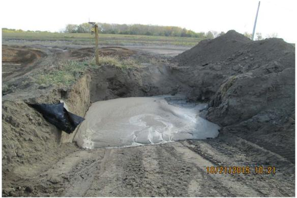
Photograph 8 A - View of flowable fill placed over the demolished lift station at Ash Pond C.
