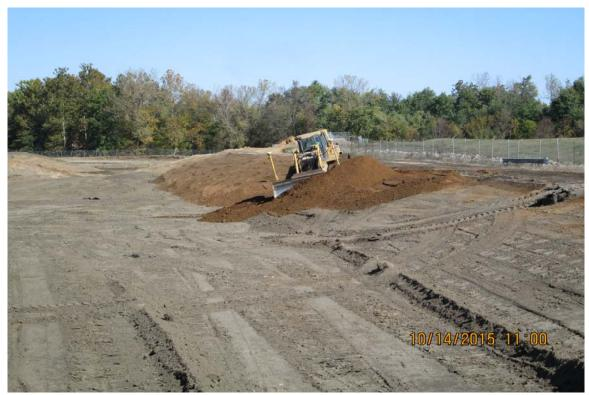
Photograph 6 ^ - View of grading the two feet of material placed on the Ash Pond C levees, looking northeast.
