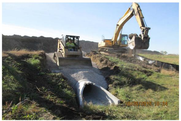
Photograph 2 A - Placing gravel over RCP culvert under the main access road near the northeast corner of Ash Pond A, looking south.
