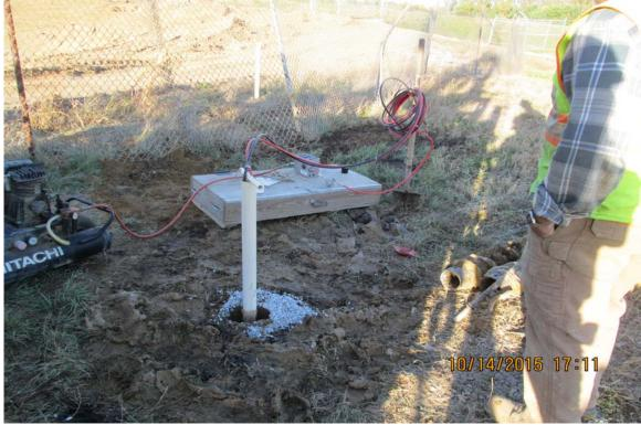
Photograph 10 A - View of setup for monitoring well development.
