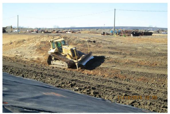
Photograph 2 A - View of bulldozer grading material in the Bottom Ash Pond.
