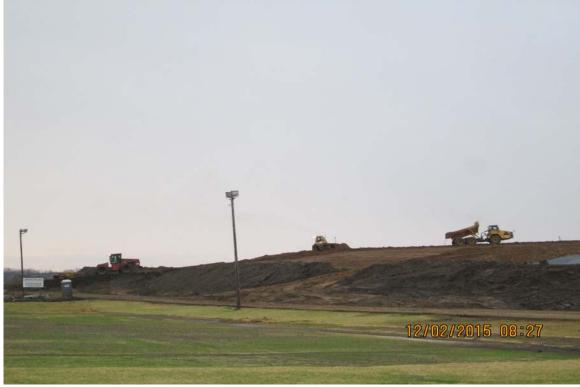
Photograph 11 A - View of Ash Pond A protective cover placement, looking east.
