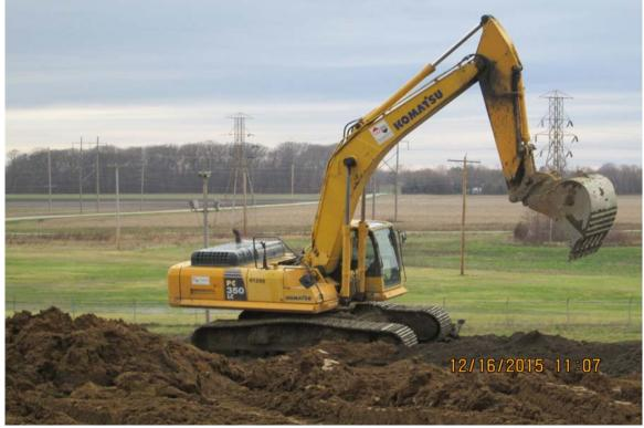
Photograph 1 A - View of excavator on Ash Pond A levee folding levee material with protective cover, looking west.
