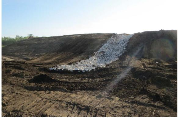
Photograph 2 A - View of placed rip-rap and geofabric at the southwest corner of Ash Pond A, looking east.
