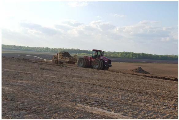
Photograph 2 A - View of topsoil placement on Ash Pond A, looking southwest.
