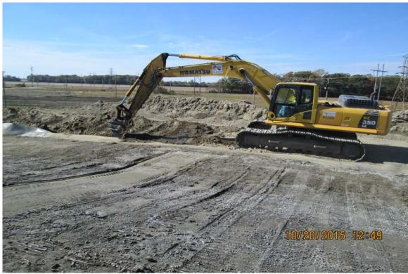
Photograph 5 A - View of anchor trench construction on the west edge of Ash Pond A.
