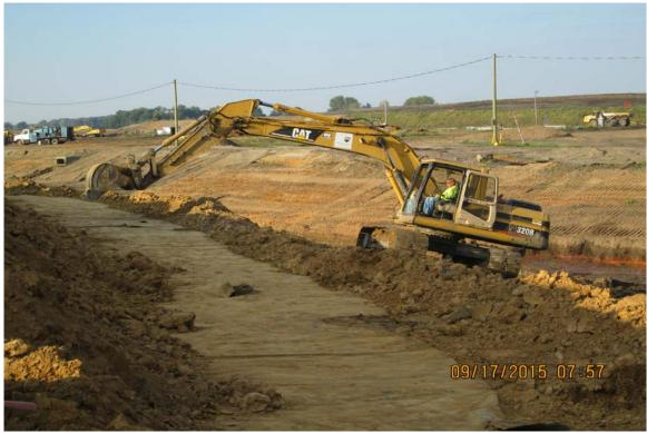
Photograph 15 A - View of exposing the Ash Pond D liner at the Bottom Ash Pond, looking southwest.
