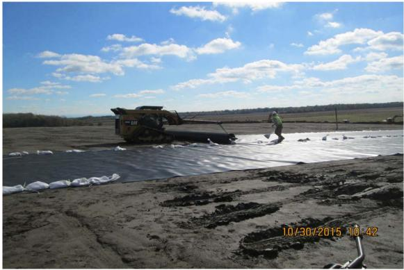
Photograph 13 A - View of placing panels on Ash Pond A, looking southeast.
