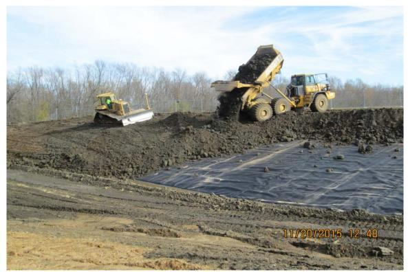
Photograph 9 A - View of placing and grading protective cover on the Ash Pond D slope, looking northeast.
