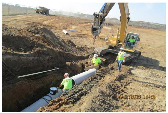
Photograph 12 ^ - View of placing concrete pipe at the Ash Pond B outfall location, looking southwest.
