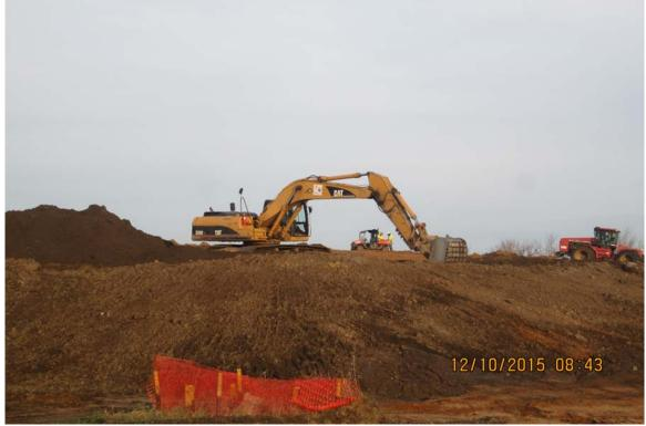
Photograph 5 A - View of Ash Pond A levee material placement, looking west.
