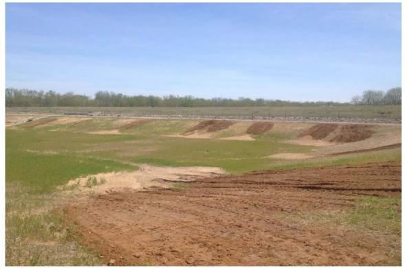
Photograph 4 A - View of erosion repairs at Ash Pond C, looking north-northeast.
