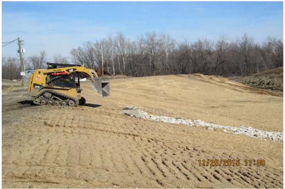
Photograph 8 ^ - View of placing additional rip rap at the west Ash Pond C box culvert, looking north.
