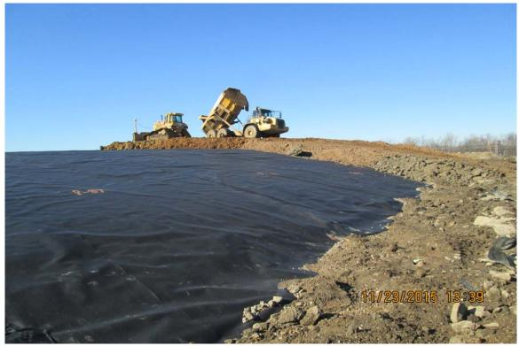
Photograph 4 A - View of protective cover placement on Ash Pond A, looking west.
