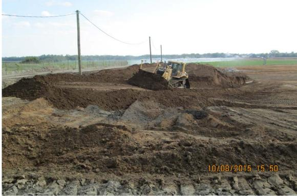
Photograph 9 A - View of grading soil over ash at the northeast corner of Ash Pond B, looking south.
