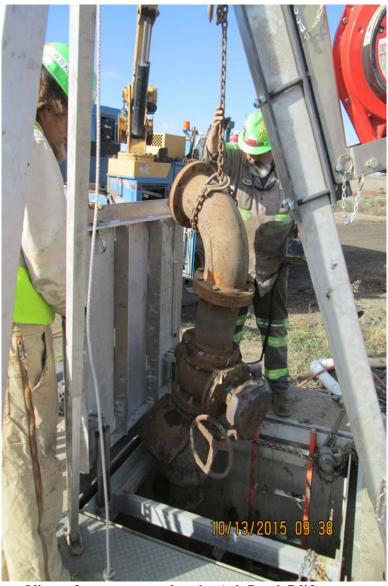
Photograph 3 A - View of pump removal at the Ash Pond C lift structure.
