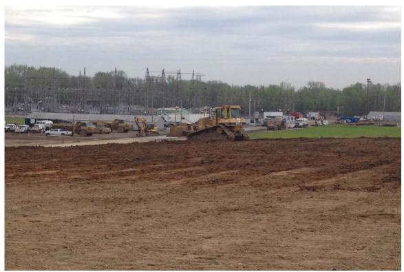
Photograph 10 ^ - View of surface shaping of the northern portion of Ash Pond A prior to placement of topsoil, looking north-northwest.
