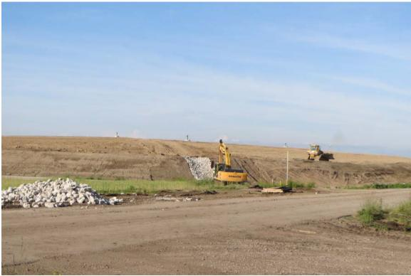
Photograph 3 A - View of rip-rap and geofabric placement at the northern corner of Ash Pond A, looking west.
