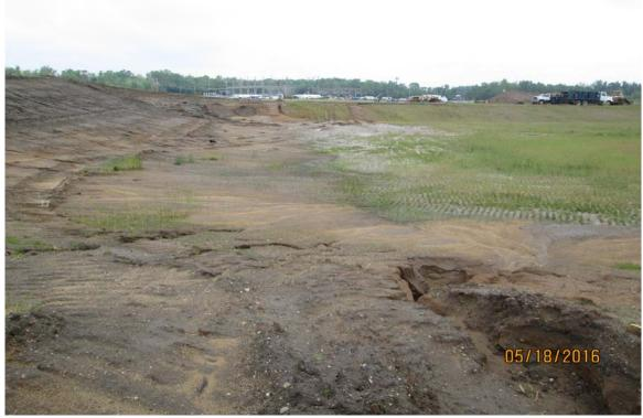
Photograph 4 A - View of Ash Pond B and erosion on the southwestern slope, looking north.
