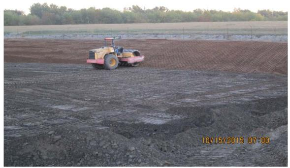
Photograph 11 A - View of compacting soil at the Ash Pond C levees, looking northeast.
