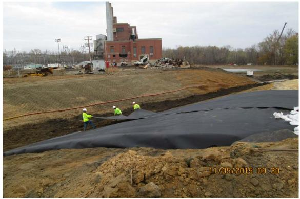
Photograph 11 A - Placing HDPE geomembrane on the Ash Pond D slope, looking northeast.
