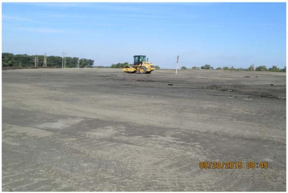
Photograph 2 A - View of smooth drum roller compacting Ash Pond A, looking north.
