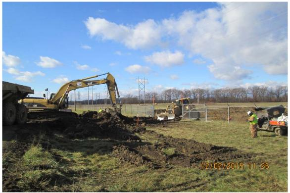
Photograph 14 ^ - View of haul road ramp soil removal after repair of internet cable, looking southwest.
