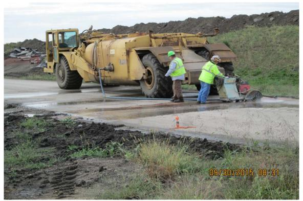
Photograph 12 ▲ - View of road sawcuts for HDPE culvert installation.
