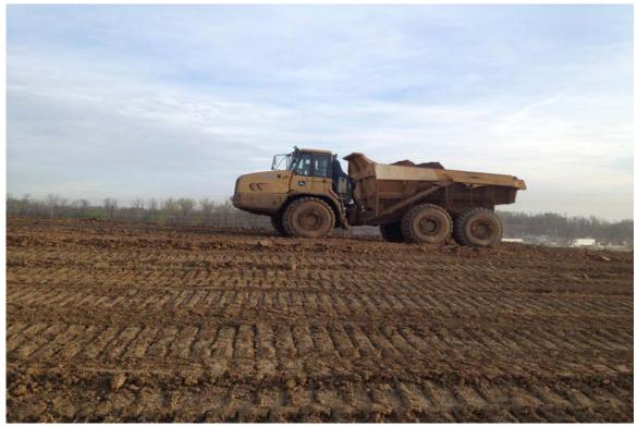
Photograph 6 A - View of hauling of topsoil to place on Ash Pond A, looking north.
