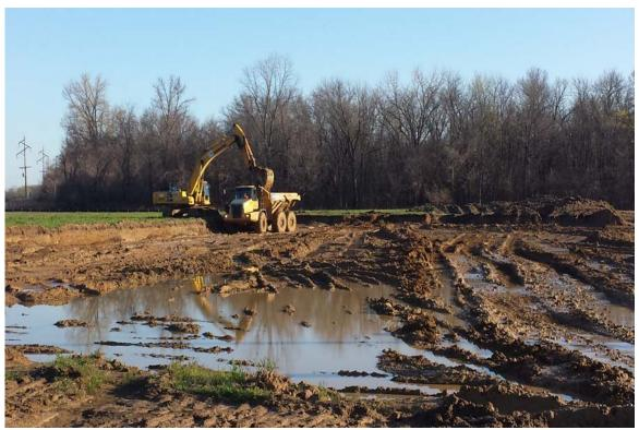
Photograph 2 A - View of material excavation from the borrow field for placement on Ash Pond A, looking northeast.
