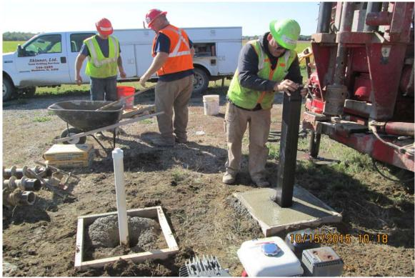
Photograph 14 A - View of installing well covers at Monitoring Wells MW-22S and MW-22D.
