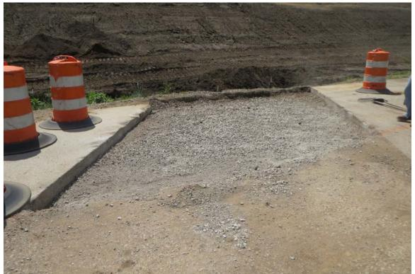
Photograph 8 ^ - View of the roadway surface, prepared for concrete replacement on the north side of Ash Pond A, looking south.
