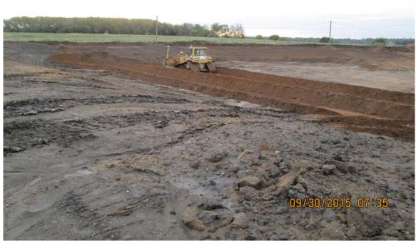
Photograph 8 A - Typical view of smooth-rolled portions of Ash Pond A after rain, showing rill development.
