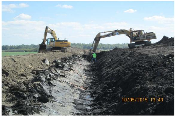
Photograph 4 ^ - View of excavators cleaning the liner at the Ash Pond A levees, looking northeast.
