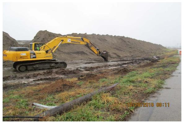
Photograph 6 ^ - View of excavation of ditch between installed culverts at the intersection north of Ash Pond A, looking south.
