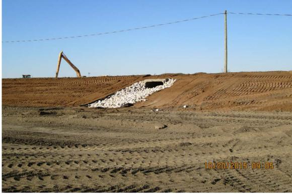
Photograph 3 A - View of rip-rap apron at culvert in the west levee of Ash Pond C.
