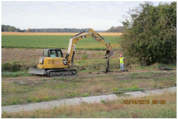
Photograph 5 A - View of silt fence removal around Ash Pond D.
