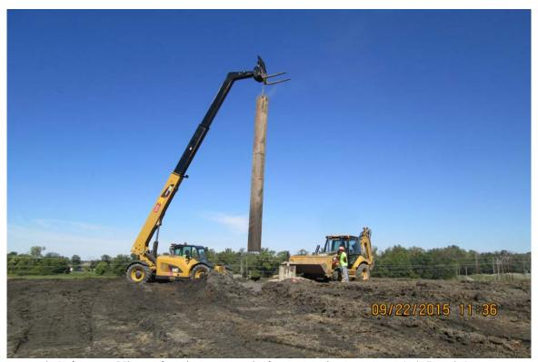
Photograph 9 A - View of casing removal after vent placement on Ash Pond A.
