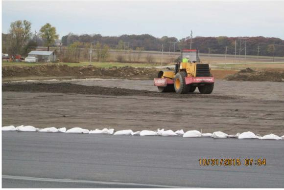
Photograph 15 ^ - View of smooth-roller on the southwest corner of Ash Pond A, looking southwest.
