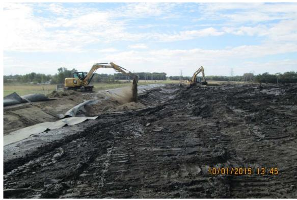
Photograph 17 A - View of placing dry soil to bridge over wet ash at the west corner of Ash Pond A.
