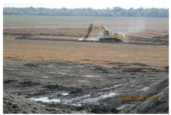
Photograph 2 A - Excavating drainage swale in Ash Pond B, looking south.
