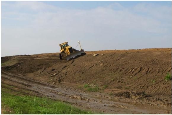
Photograph 5 A - View of grading/drying soils on the east slope of Ash Pond A, looking southwest.
