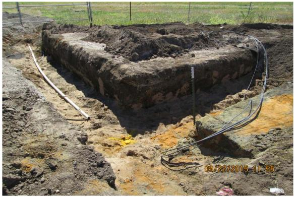
Photograph 10 ^ - View of electrical conduit trench adjacent to the southeast corner of Ash Pond B, looking south.
