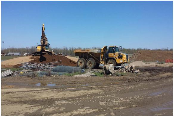
Photograph 4 A - View of sandy soil for use as backfill for removed soil at the former fuel tank location, looking east.
