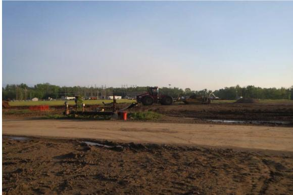
Photograph 15 ^ - View of tractor with pan moving soil to Ash Pond A for berm placement, looking north.
