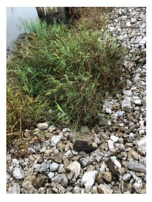
Figure 2 - Excess vegetation around secondary spillway inlet.
