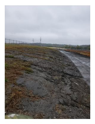
Figure 5 – Minor erosion and poor sod cover on the north side of the impoundment.
