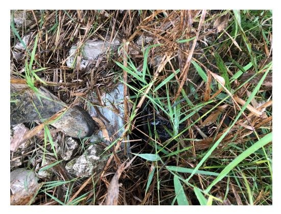
Figure 3 - Excess vegetation around secondary spillway inlet.
