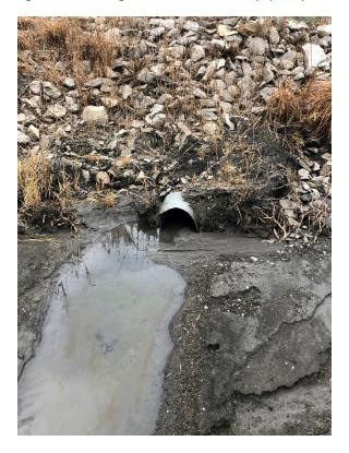
*Figure 4 - Secondary spillway approximately 1/4 to 1/3 full of sediment.*
