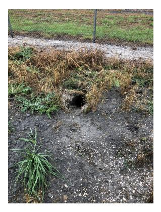
*Figure 9 – Large animal burrow was observed on the crest near the center of the north section of the embankment.*
