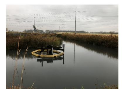
Figure 1 – Principal spillway skimmer, pipe supports and stoplogs.
