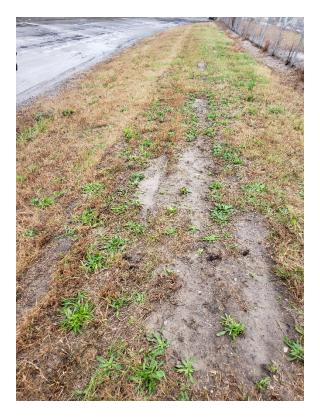
Figure 7 – Sparse vegetative cover on downstream slope.
