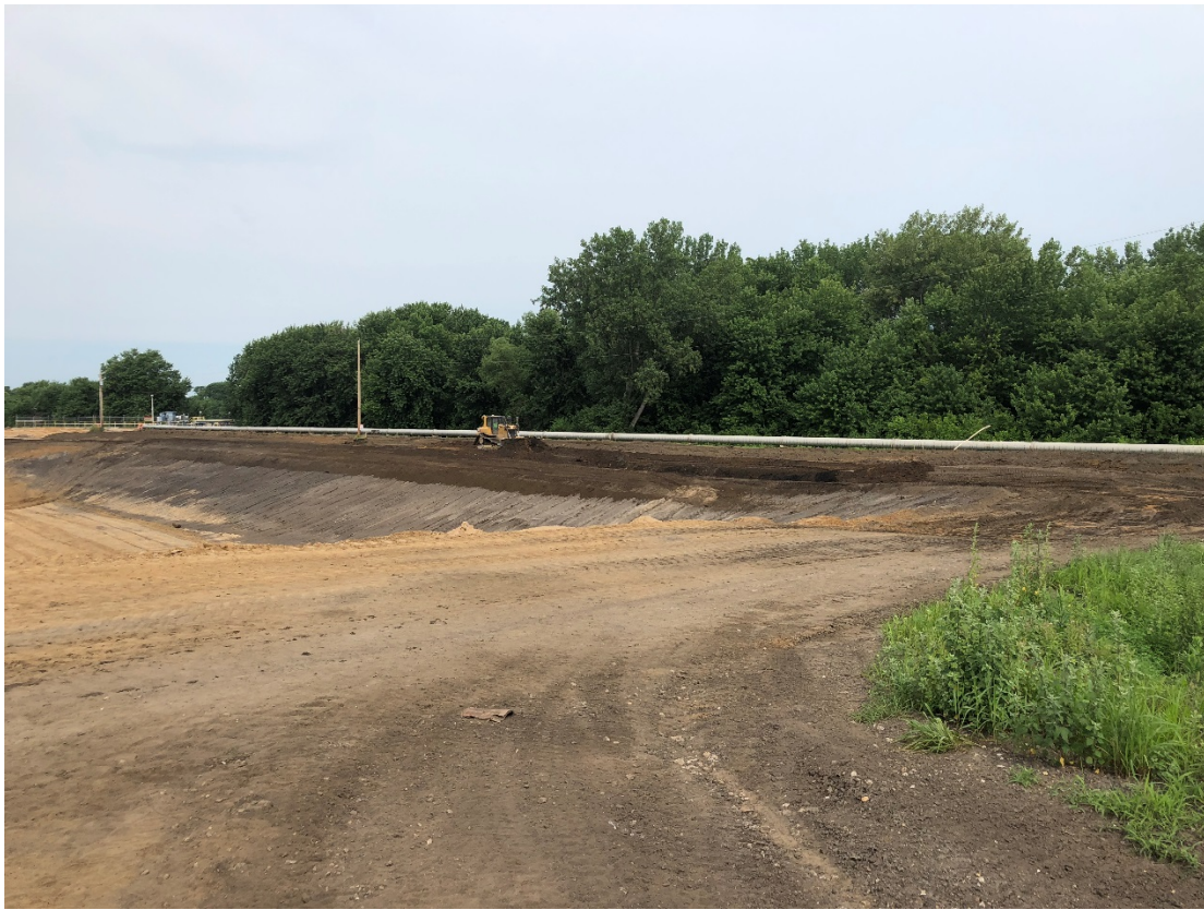
Photograph 1 ▲ - View of Bottom Ash Pond berm backfill and grading activities, looking west.
