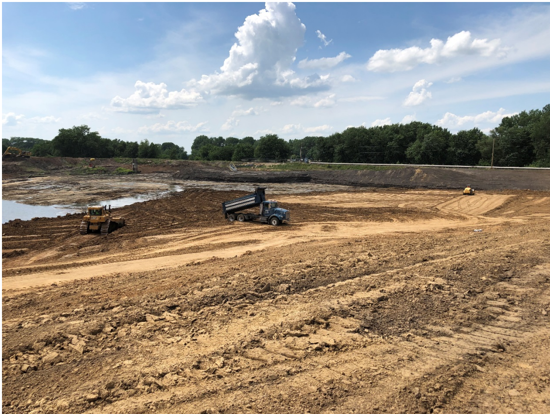
Photograph 1 ▲ - View of borrow soil placement at the Bottom Ash Pond, looking west.
