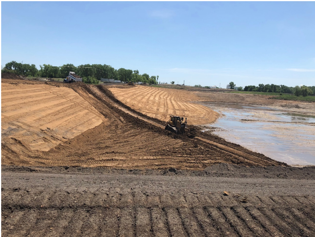
Photograph 7 ▲ - View of borrow soil placement at the Bottom Ash Pond on May 24, 2018, looking east.
