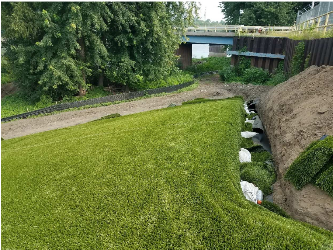
Photograph 4 ▲ - View of anchor trench at the Bottom Ash Berm, looking northwest.
