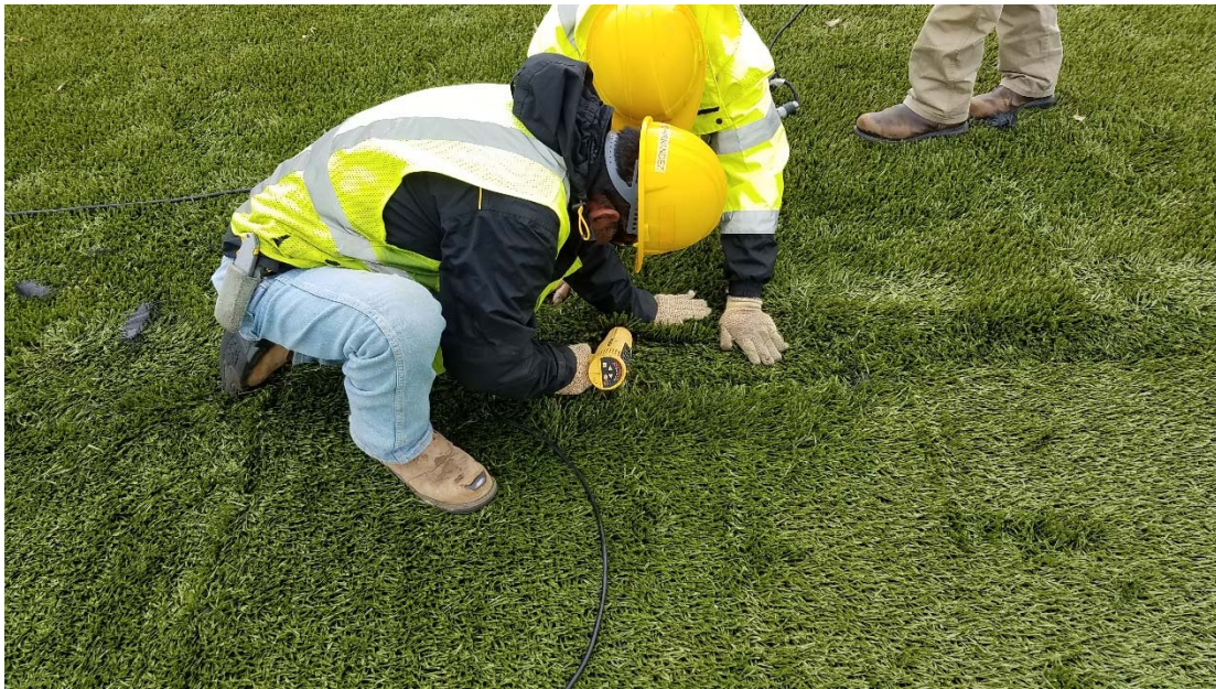
Photograph 1 ▲ - View of typical repair of the engineered turf geosynthetics.
