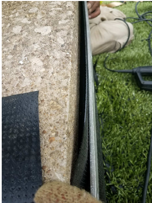
Photograph 6 ▲ - View of pipeline seal detail at Bottom Ash Berm.
