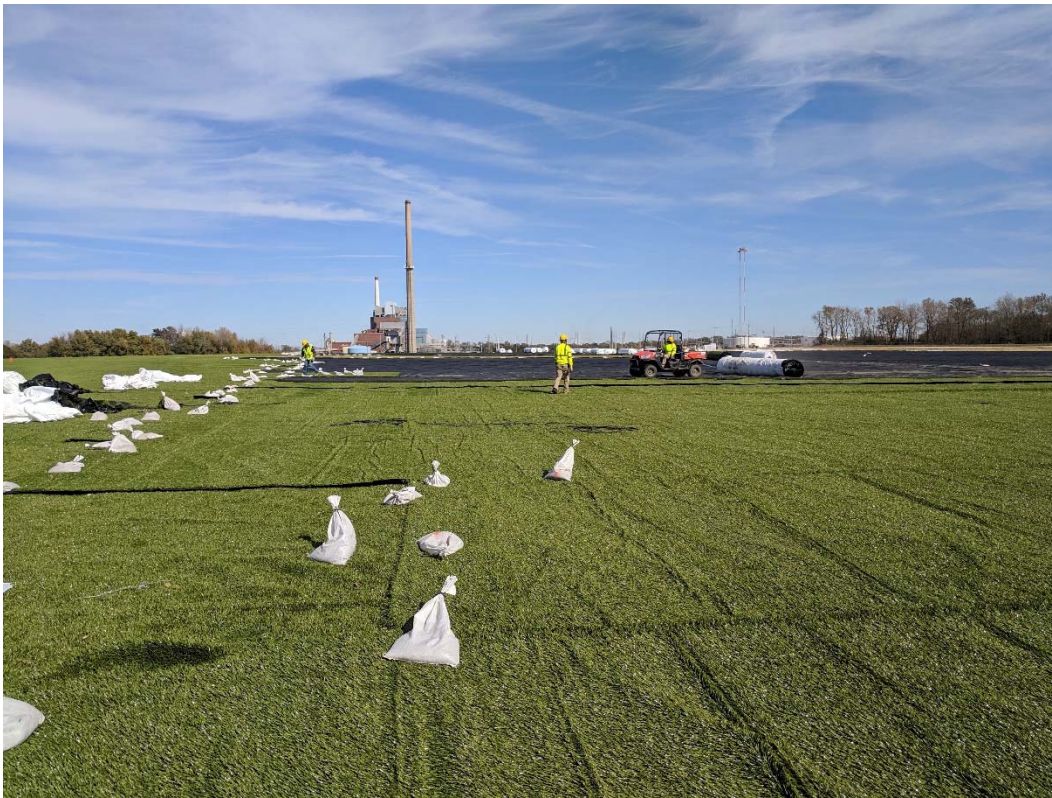
Photograph 1 ▲ - View of typical placement of the engineered turf geotextile, facing north.
