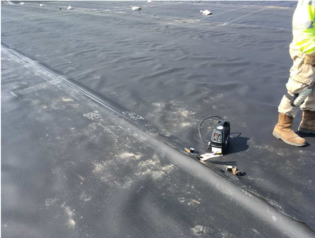
Photograph 3 ▲ - Typical view of air testing at the Fly Ash Pond.
