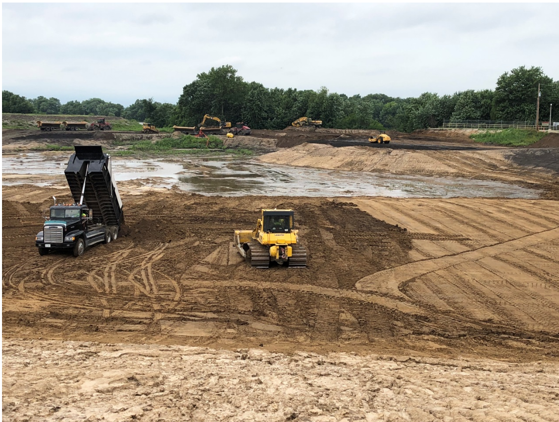
Photograph 2 ▲ - View of Bottom Ash Pond floor fill activities, looking west.
