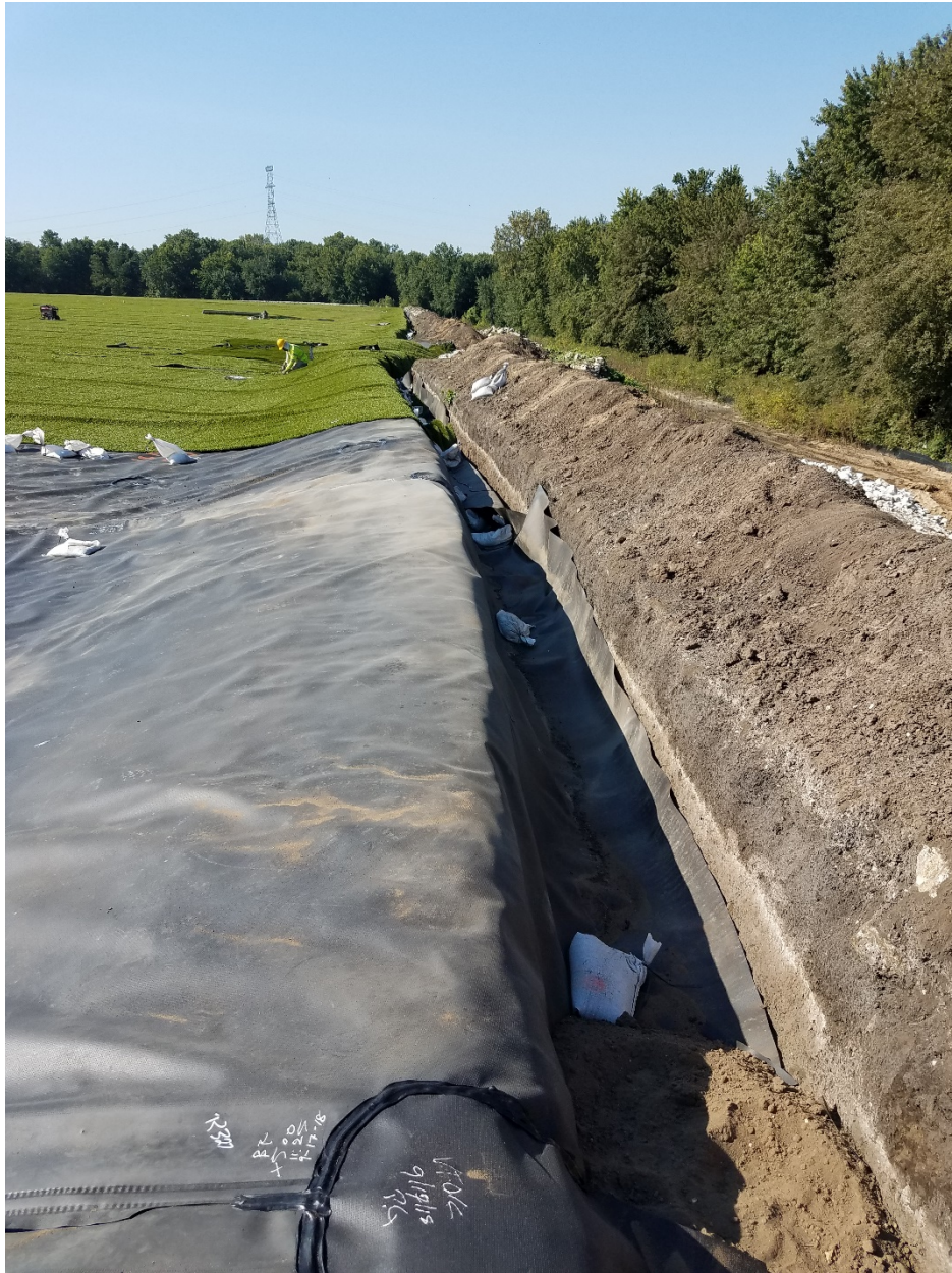
Photograph 1 ▲ - View of anchor trench at the Fly Ash Pond, looking southwest.
