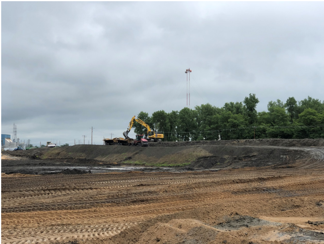
Photograph 5 ▲ - View of removal of the fly ash stockpile material, looking northeast.
