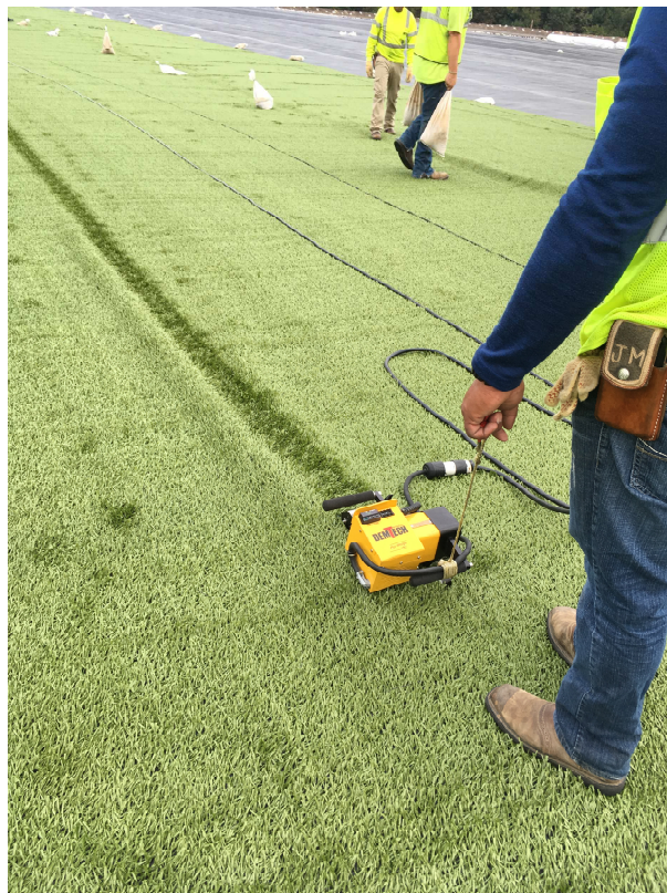
Photograph 2 ▲ - Typical view of turf welding at the Fly Ash Pond.
