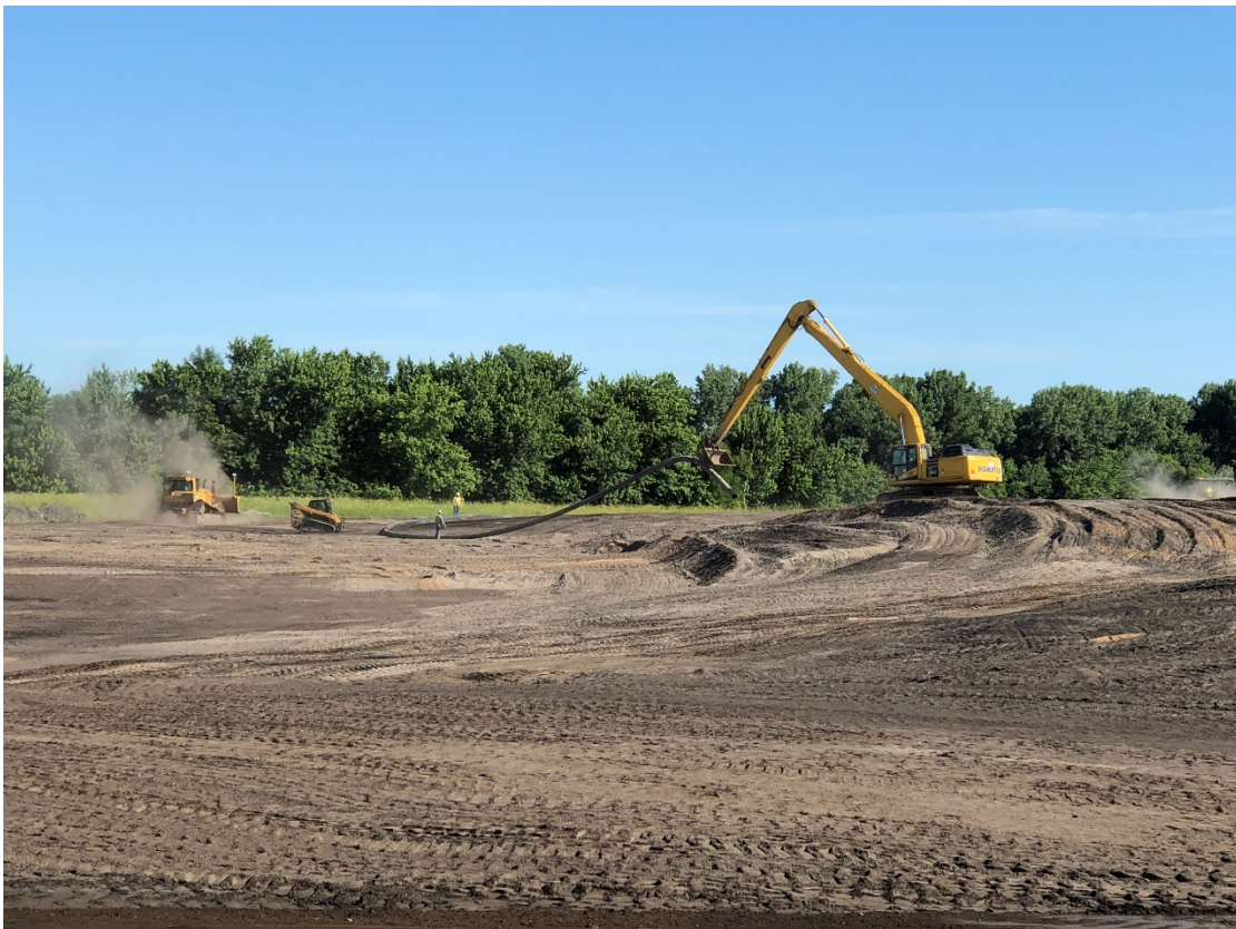
Photograph 2 ▲ - View of a long-reach excavator moving the Bottom Ash Pond discharge pipe, looking northwest.
