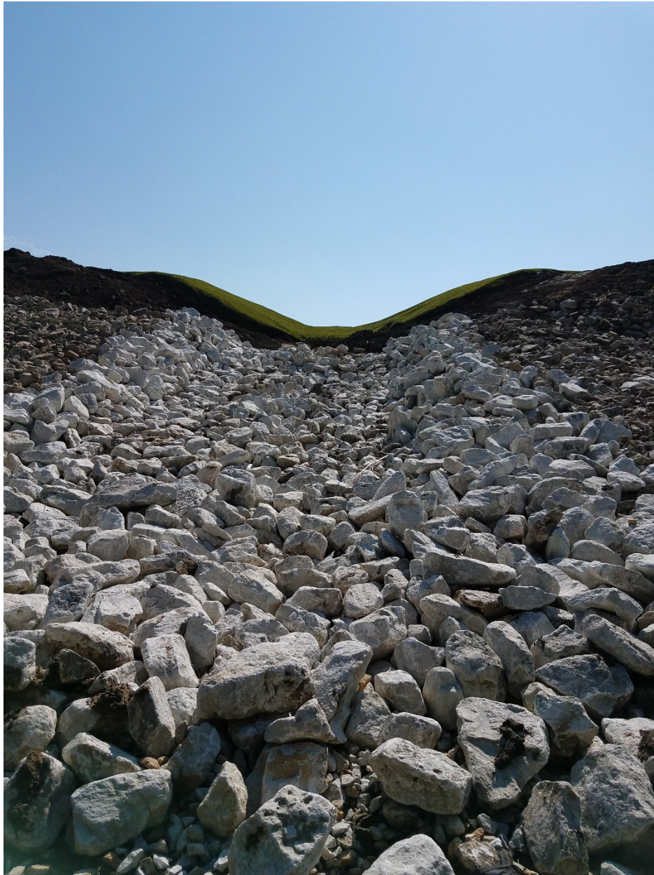
Photograph 2 ▲ - View of downlet structure at the Fly Ash Pond, facing north.
