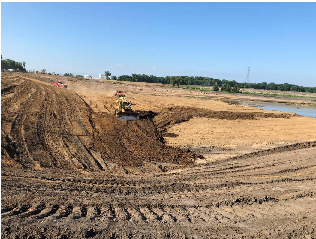
Photograph 2 ▲ - View of Bottom Ash Pond floor fill activities, looking south.
