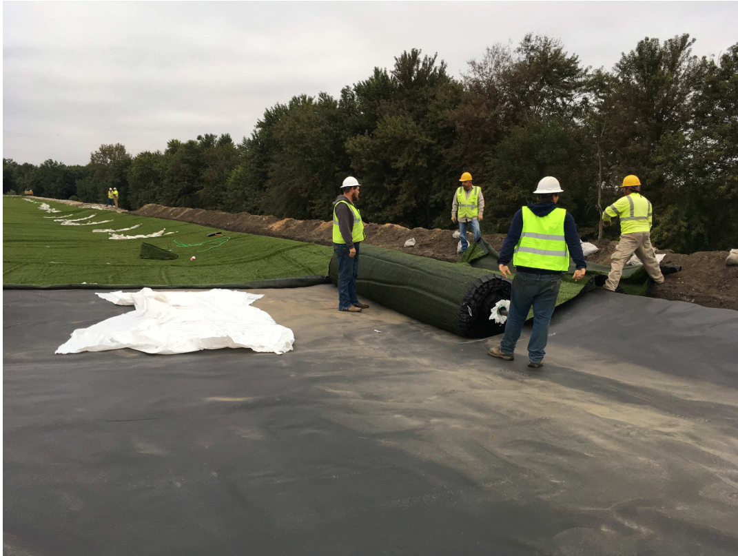
Photograph 1 ▲ - View of typical turf placement at the Fly Ash Pond, looking southwest.
