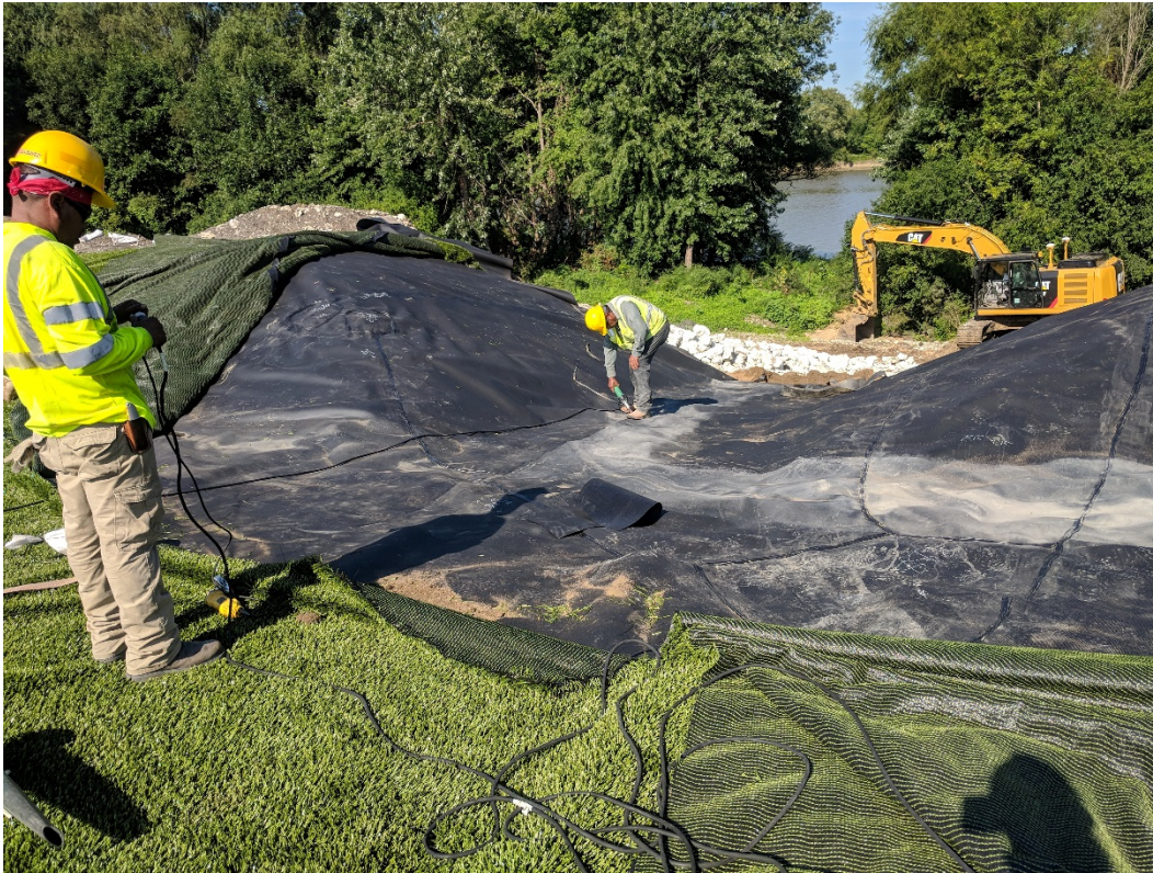
Photograph 3 ▲ - View of geomembrane repair at the eroded downchute, looking northwest.
