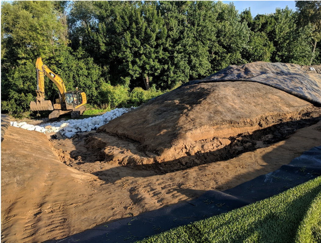
Photograph 1 ▲ - View of downchute erosion under the ClosureTurf at the Fly Ash Pond, looking north.
