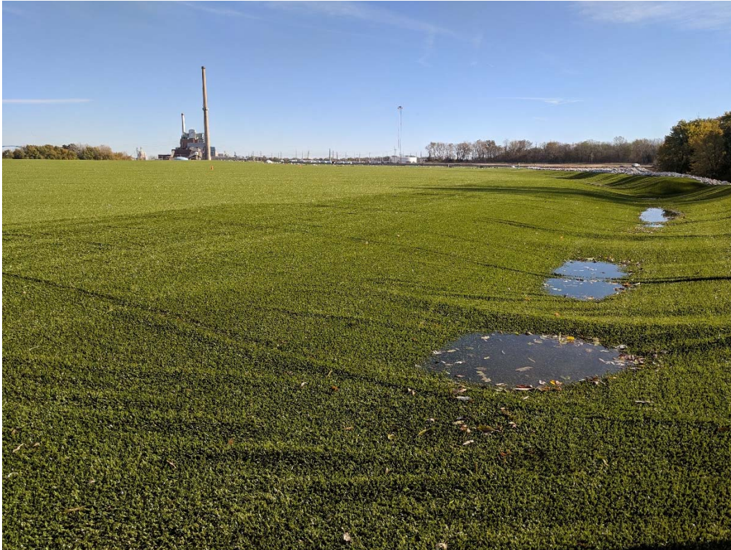
Photograph 4 ▲ - View of ponding on suspended HDPE geomembrane in the perimeter ditch, looking northeast.
