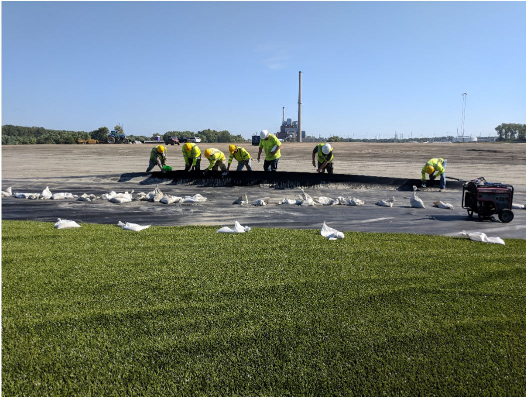
Photograph 5 ▲ - Typical view of liner cleaning activities prior to additional geomembrane installation, looking northeast.
