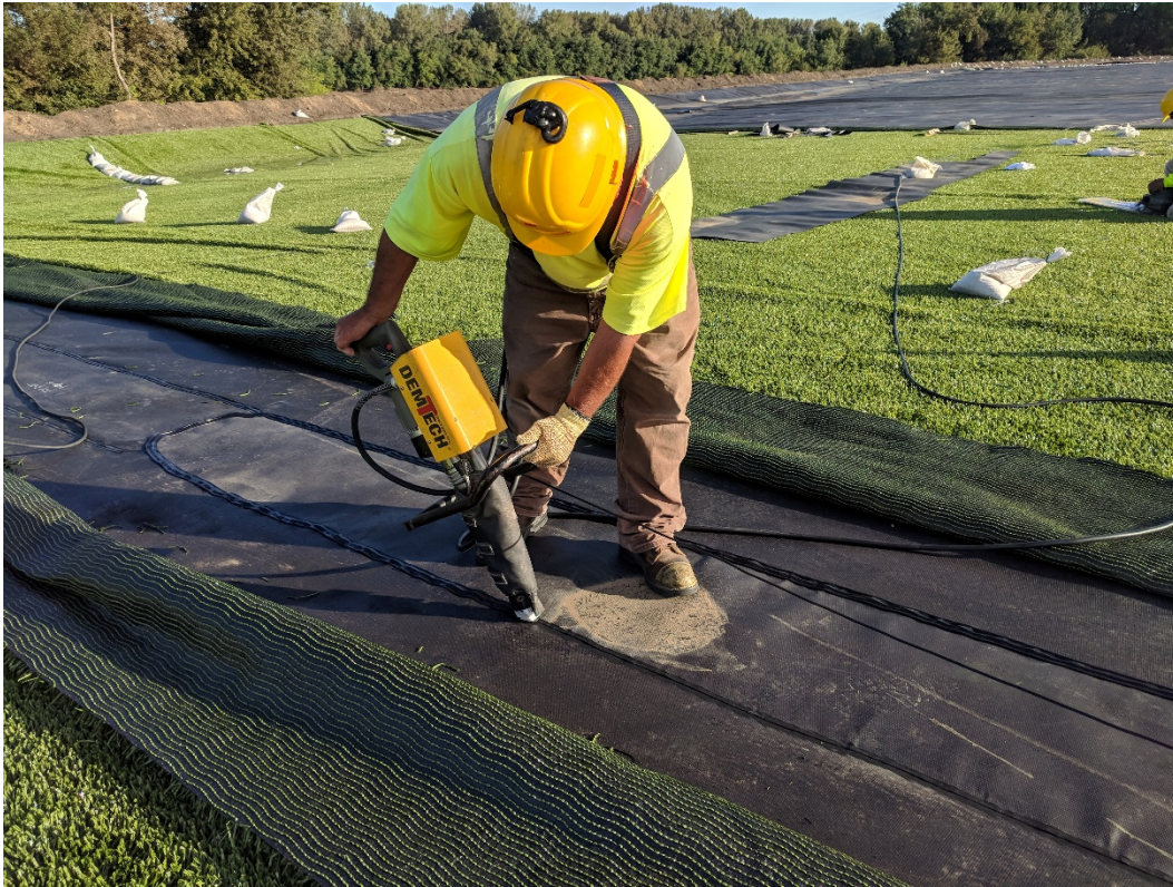
Photograph 3 ▲ - View of HDPE geomembrane repair activities at the Fly Ash Pond, facing north.
