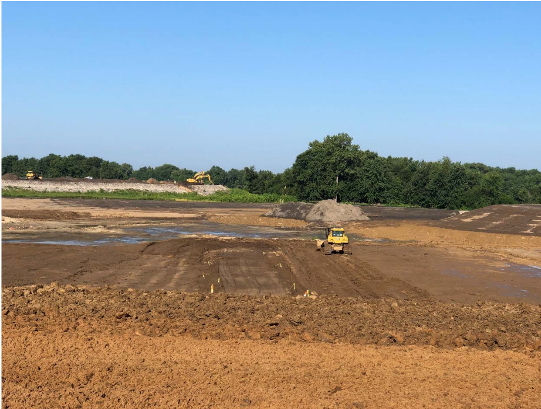
Photograph 1 ▲ - View of Bottom Ash Pond floor fill activities, looking northwest.
