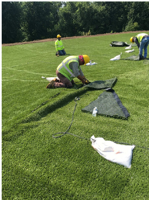
Photograph 6 ▲ - Typical view of turf repair at the Fly Ash Pond, looking northwest.
