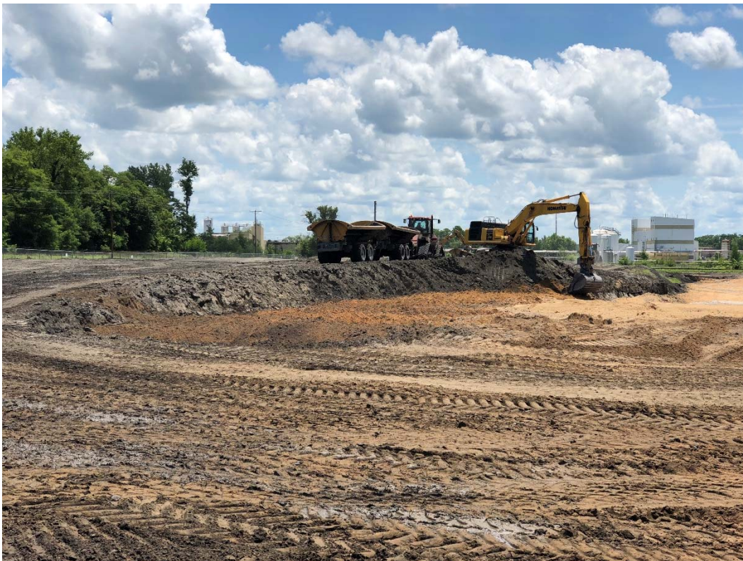
Photograph 4 ▲ - View of removal of the fly ash stockpile material, looking south.
