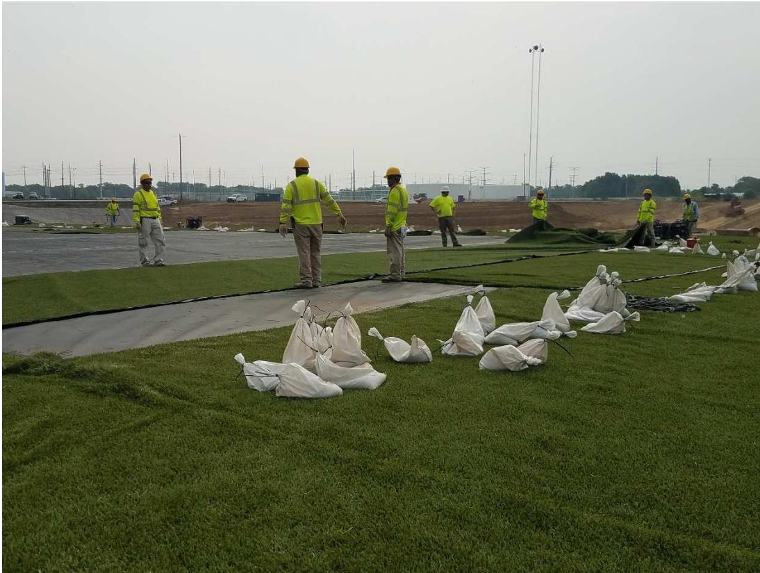
Photograph 7 ▲ - View of turf placement activities at the Bottom Ash Berm, looking northeast.
