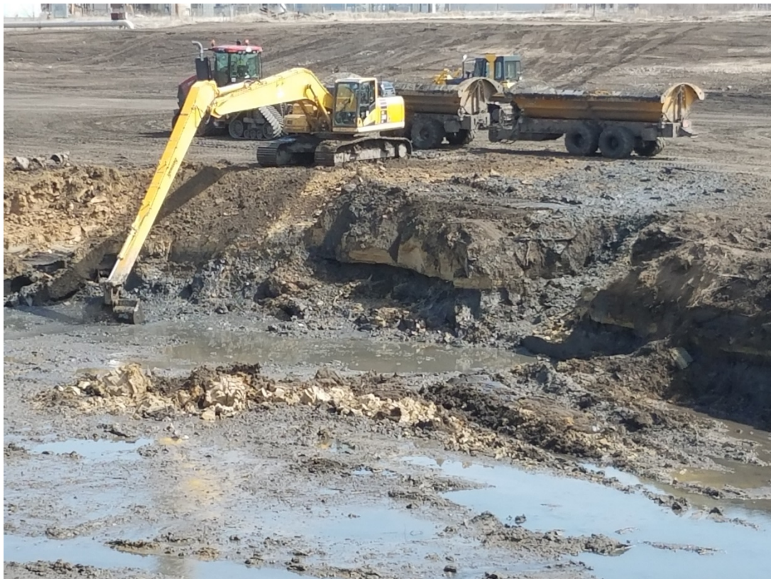
Photograph 4 ▲ - View of bottom ash removal operations observed April 11, 2018, looking northeast.
