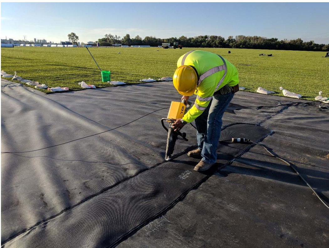
Photograph 4 ▲ - View of typical HDPE geomembrane repair activities, facing northwest.
