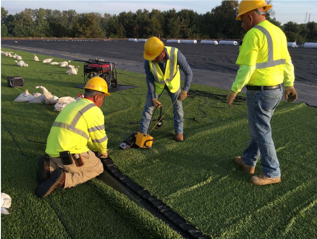
Photograph 1 ▲ - Typical view of engineered turf welding at the Fly Ash Pond, facing north.
