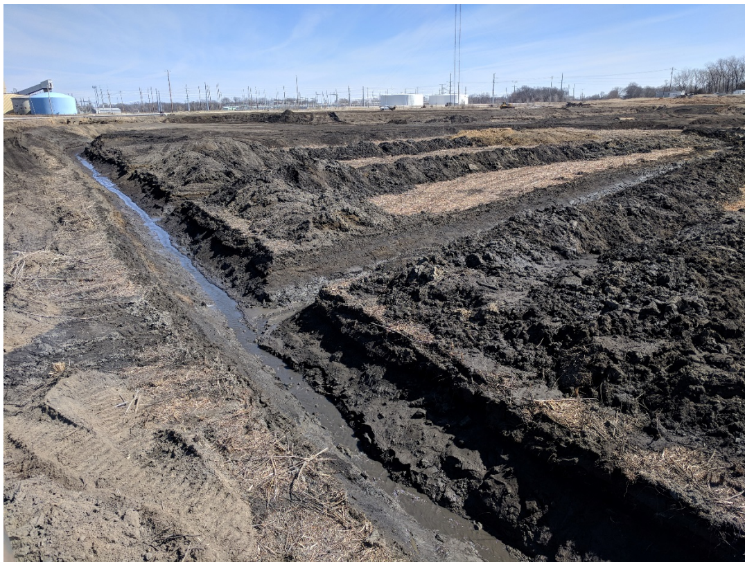
Photograph 2 ▲ - View of drainage ditches for dewatering the Bottom Ash Pond as observed March 14, 2018, looking east northeast.
