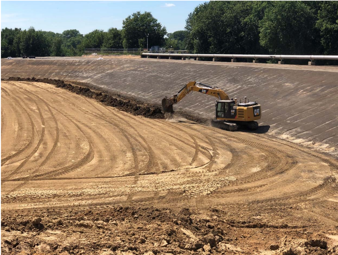
Photograph 3 ▲ - View of anchor trench excavation activities at the Bottom Ash Berm, looking west.
