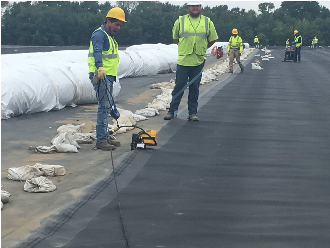
Photograph 4 ▲ - View of typical HDPE geomembrane welding activities, facing northwest.
