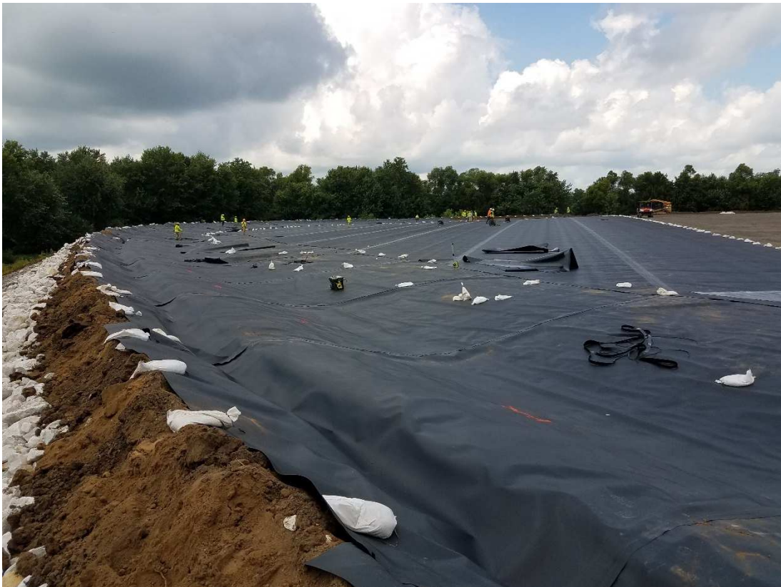
Photograph 12 ▲ - View of geomembrane installation at the Fly Ash Pond, looking northeast.
