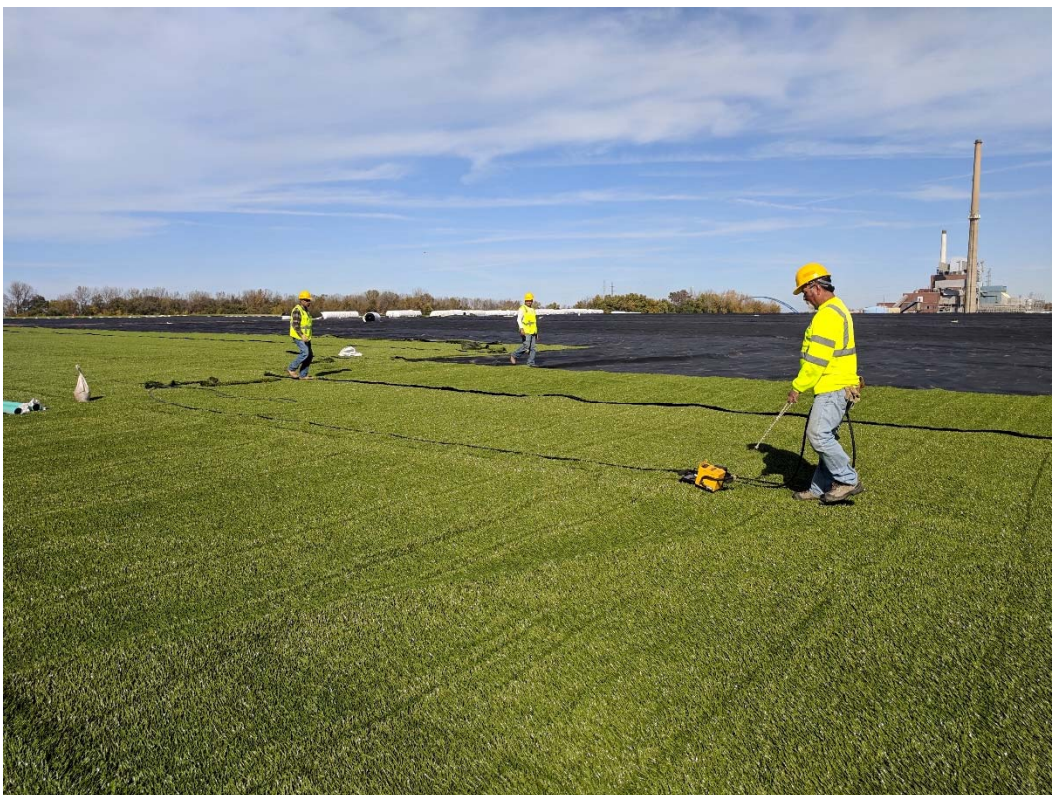
Photograph 2 ▲ - View of typical welding of the engineered turf geotextile, facing north.
