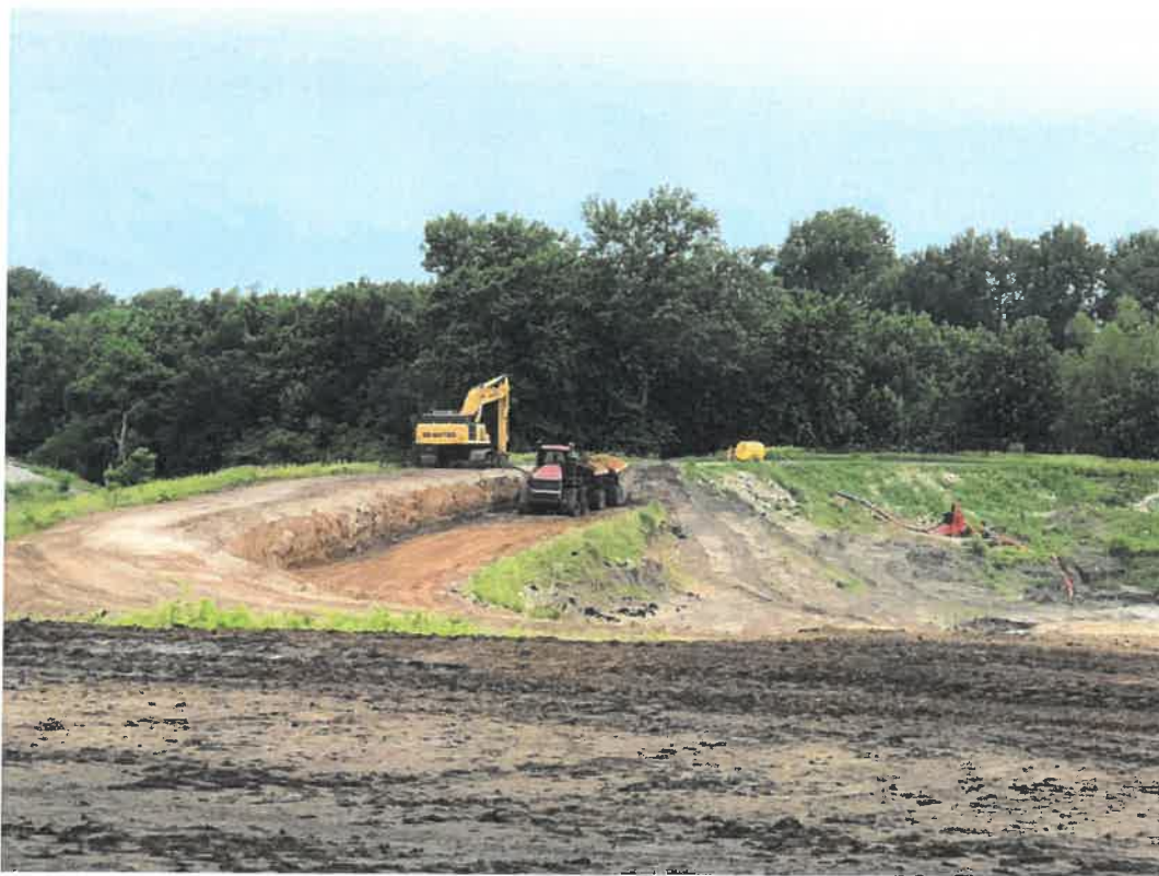
Photograph 6 ▲ - View of removal of the southwest berm of the Bottom Ash Pond, looking west.
