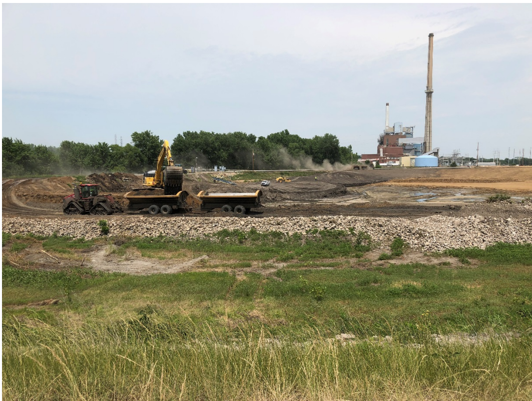
Photograph 6 ▲ - View of removal of the southwest berm of the Bottom Ash Pond, looking northeast.
