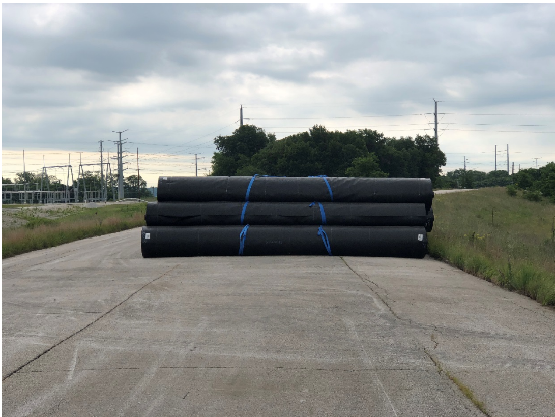
Photograph 6 ▲ - View of geomembrane (40-mil HDPE MicroSpike) storage on site, looking southeast.
