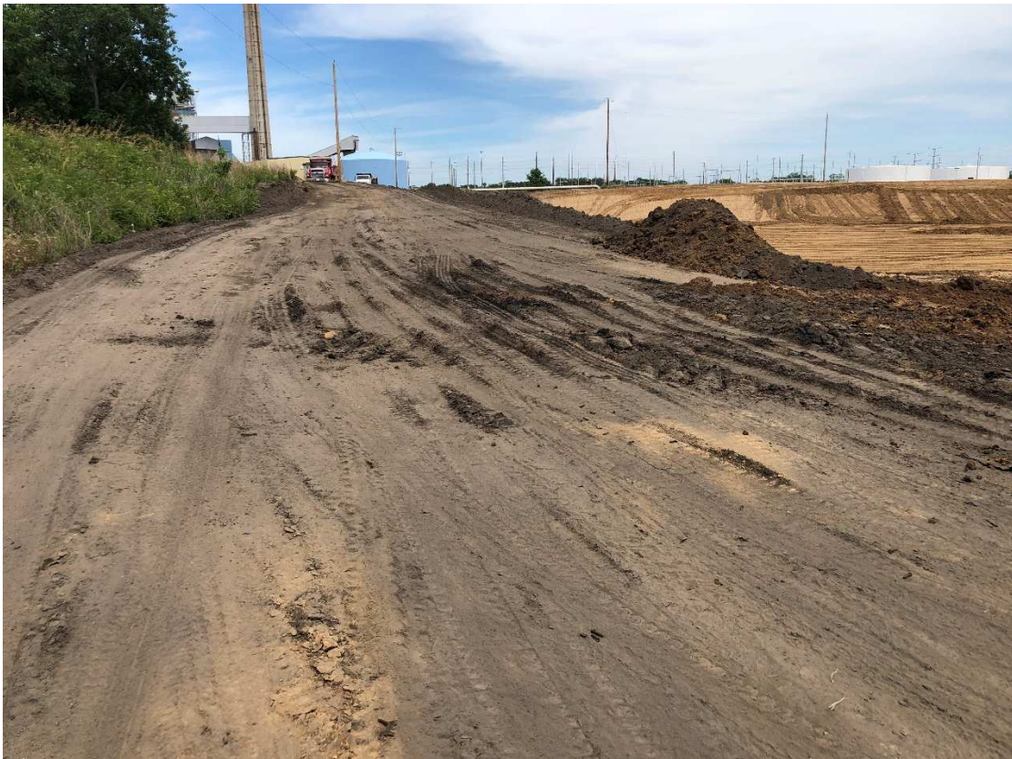
Photograph 4 ▲ - View of Bottom Ash Pond berm backfill activities with pumping subgrade (repaired next day), looking east.
