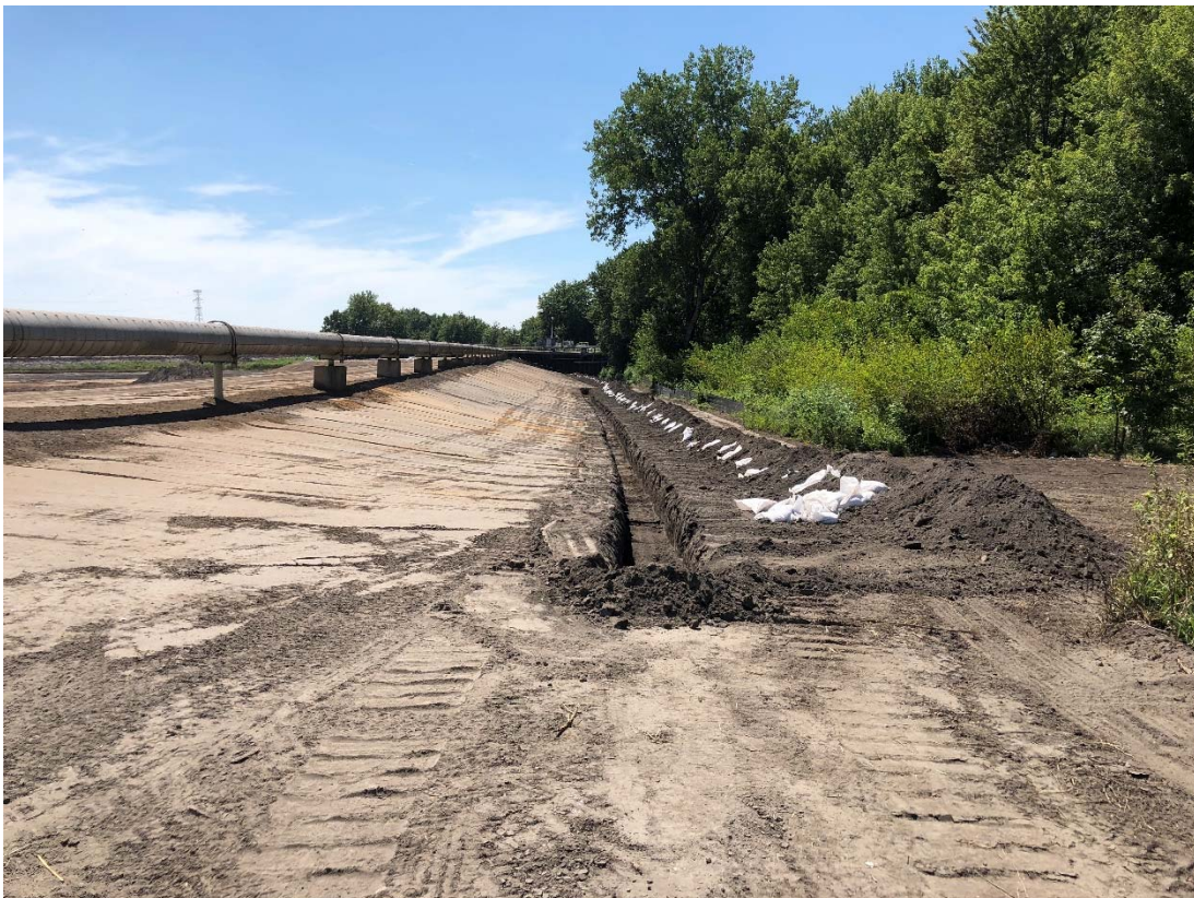
Photograph 4 ▲ - View of anchor trench at the Bottom Ash Berm, looking west.
