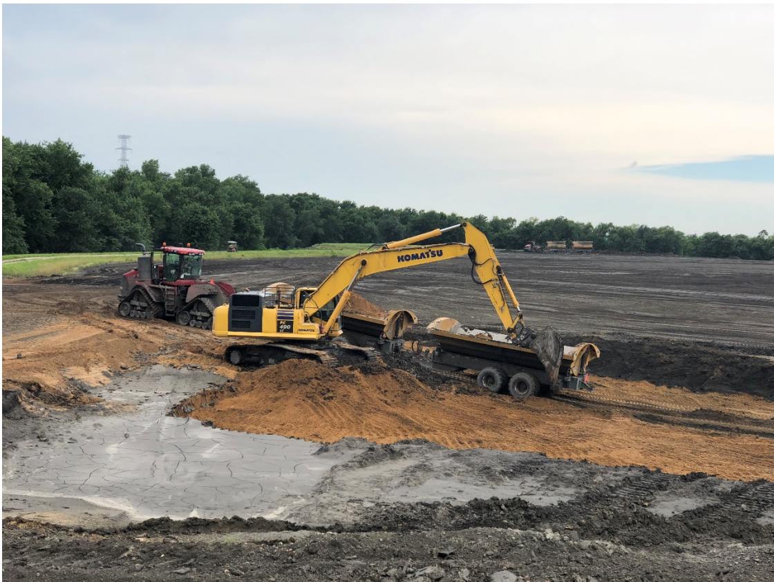
Photograph 4 ▲ - View of removal of the fly ash stockpile material, looking northeast.
