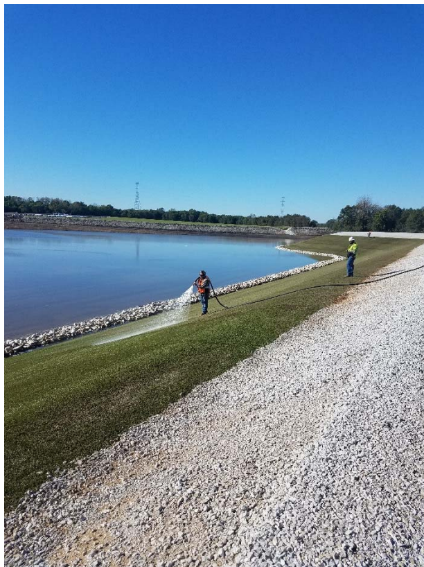
Photograph 4 ▲ - View of ArmorFill placement activities at the Bottom Ash Pond berm, facing west.
