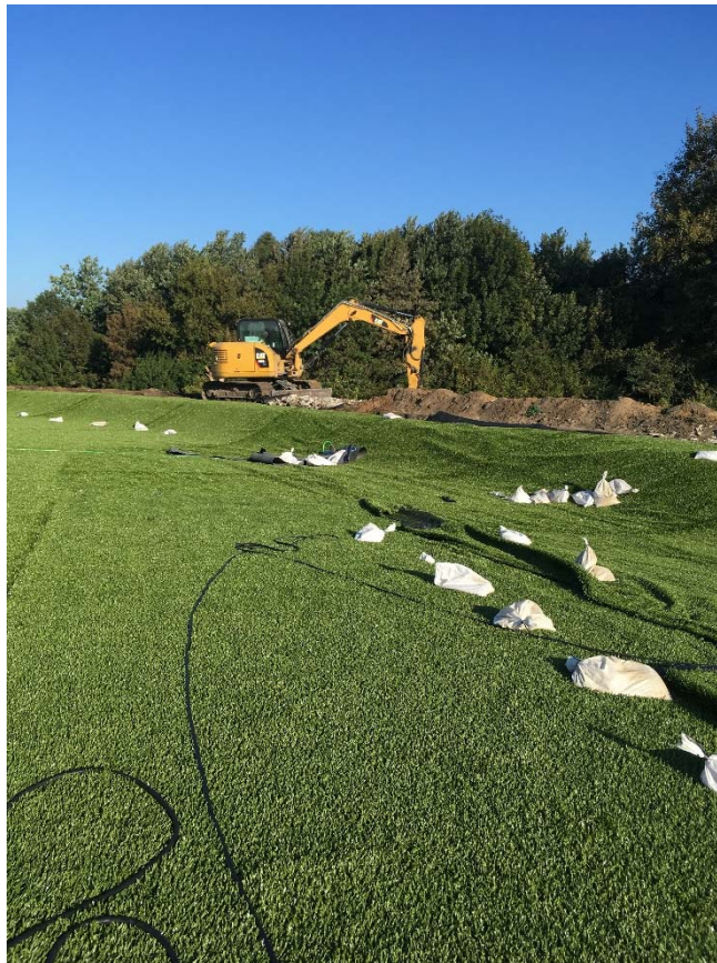
Photograph 5 ▲ - View of typical anchor trench backfill at the Fly Ash Pond, facing west.
