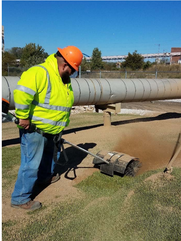
Photograph 3 ▲ - View of sand brushing at the Bottom Ash Pond berm, facing northeast.
