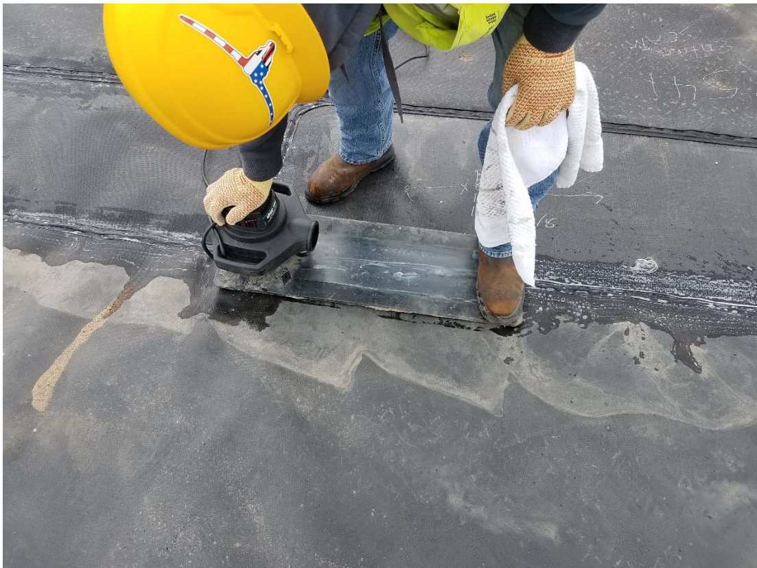
Photograph 4 ▲ - View of typical vacuum box testing of the 40-mil HDPE geomembrane.
