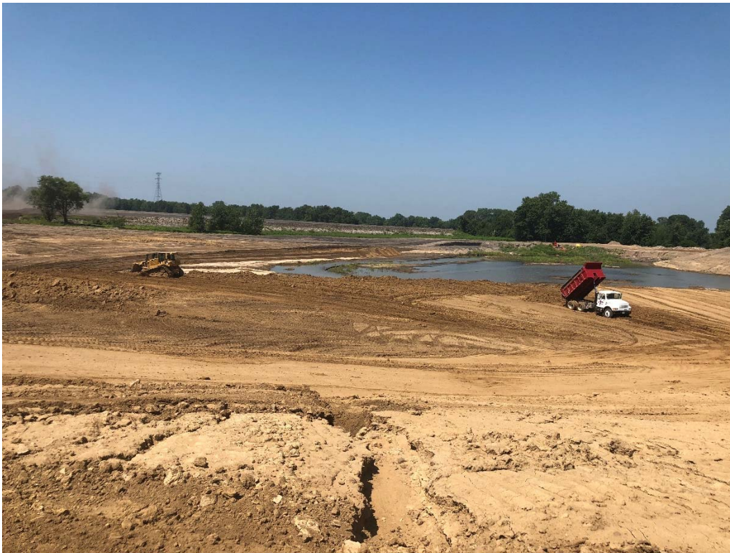
Photograph 1 ▲ - View of Bottom Ash Pond floor fill activities, looking south.
