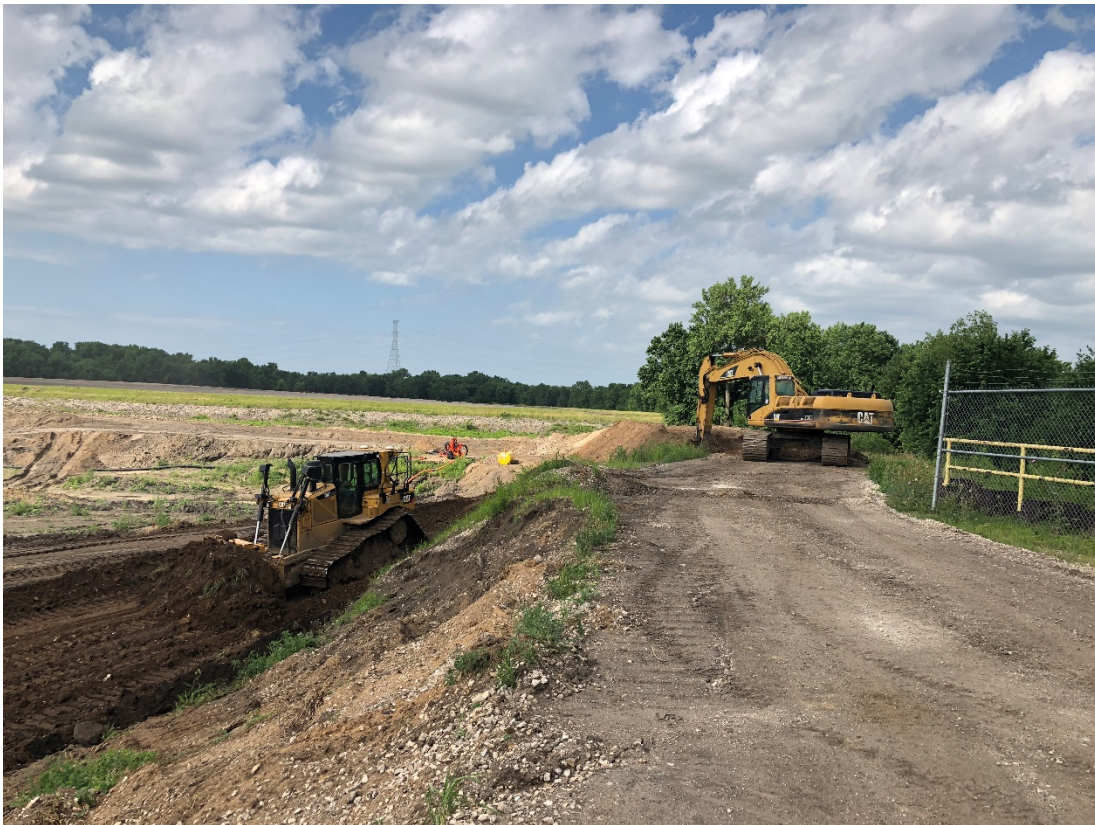
Photograph 1 ▲ - View of Bottom Ash Pond berm backfill and grading activities, looking southwest.
