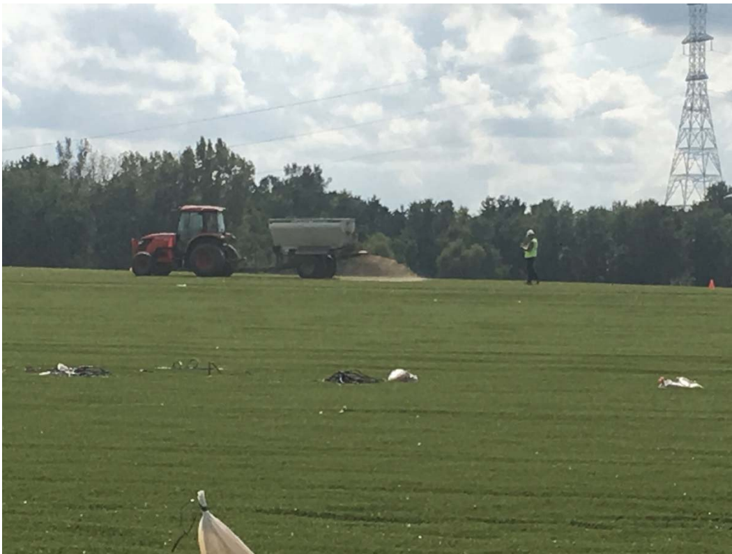
Photograph 6 ▲ - View of typical sand placement at the Fly Ash Pond, facing south.
