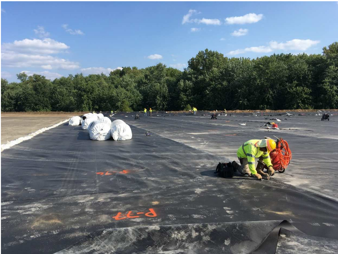
Photograph 4 ▲ - Typical view of geomembrane installation and testing, looking southwest.
