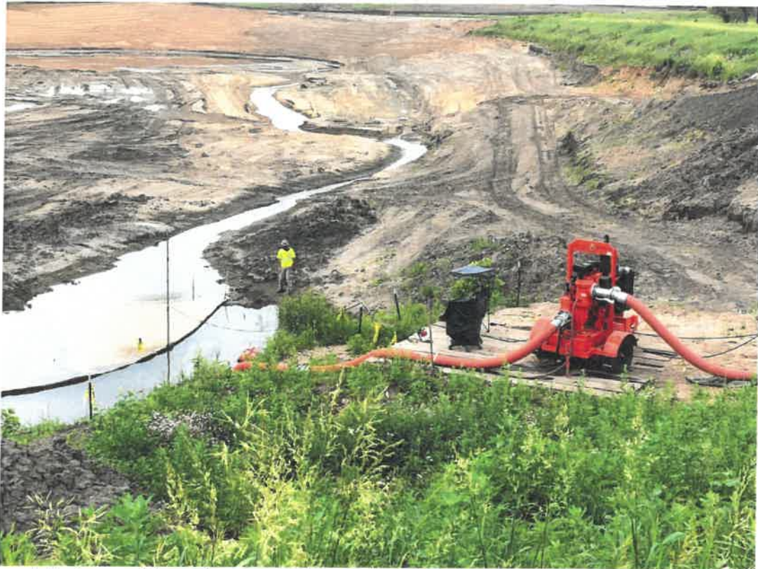
Photograph 5 ▲ - View of supervised pumping of water from the Bottom Ash Pond, looking east.
