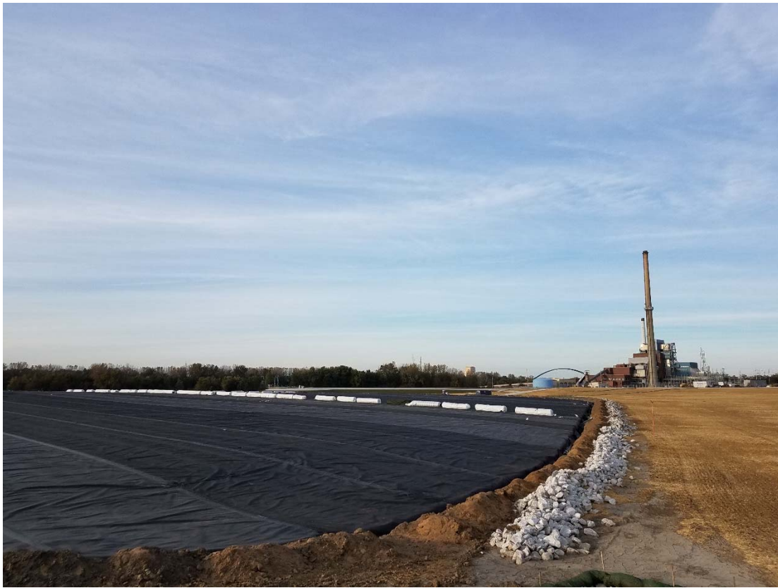
Photograph 3 ▲ - View of the Fly Ash Pond with 40 mil HDPE geomembrane and the seeded former Fly Ash Stockpile, looking north.
