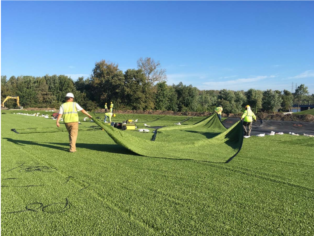
Photograph 2 ▲ - Typical view of engineered turf placement at the Fly Ash Pond, facing north.
