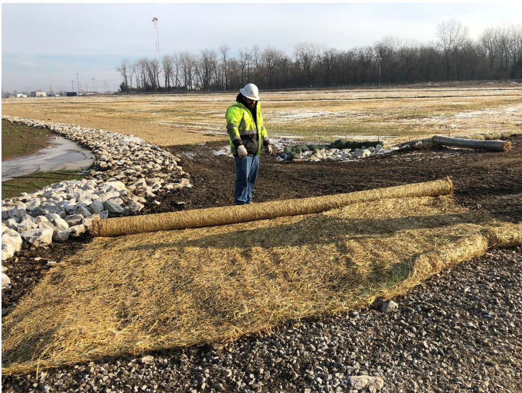
Photograph 2 ▲ - View of straw blanket placement near the Fly Ash Pond, facing northeast.
