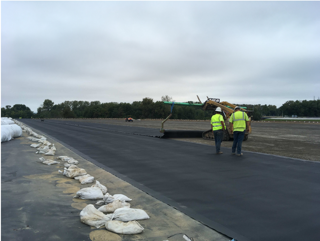
Photograph 3 ▲ - View of HDPE geomembrane placement at the Fly Ash Pond, facing west.
