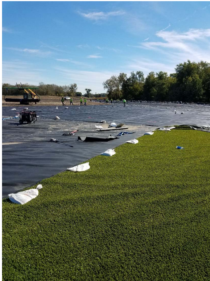
Photograph 5 ▲ - View of HDPE geomembrane placement at the Fly Ash Pond, facing southeast.
