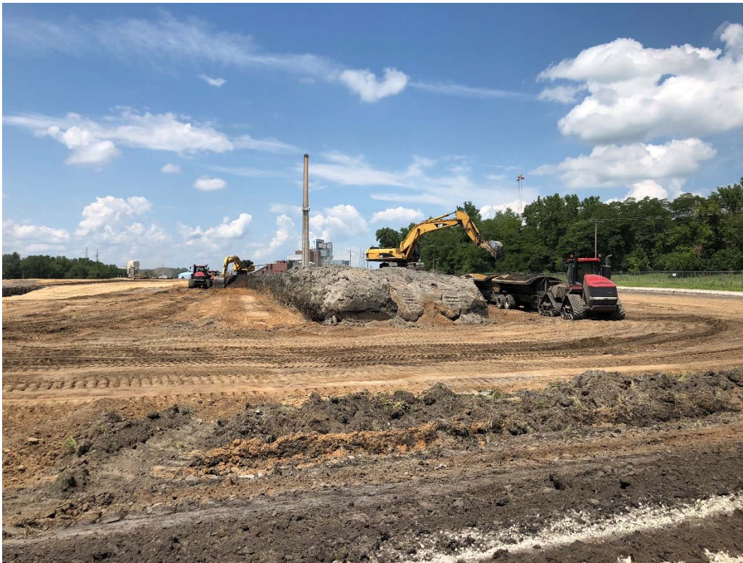
Photograph 3 ▲ - View of removal of the fly ash stockpile material, looking north.
