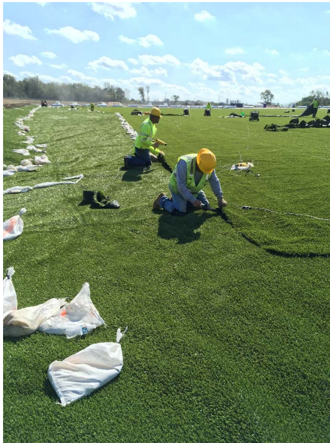
Photograph 3 ▲ - Typical view of engineered turf hand welding at the Fly Ash Pond, facing southeast.
