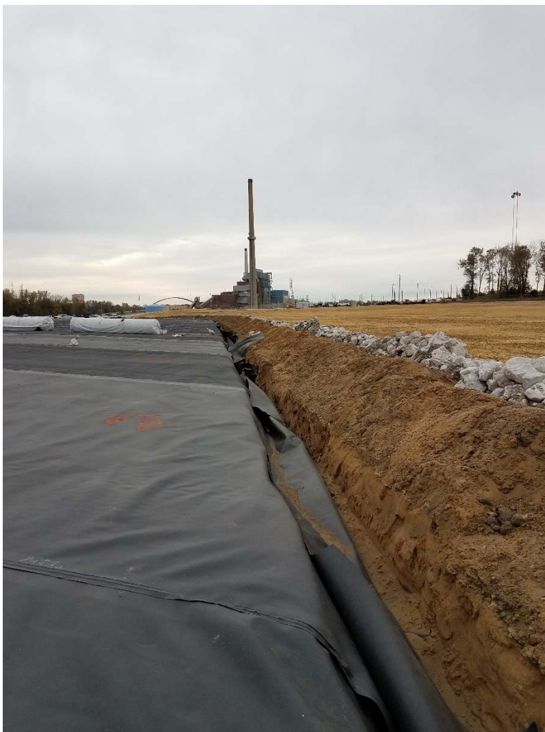
Photograph 2 ▲ - View of the eastern anchor trench at the Fly Ash Pond, facing northeast.
