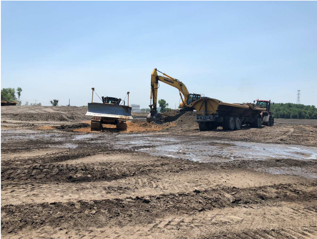
Photograph 5 ▲ - View of removal of the southwest berm of the Bottom Ash Pond, looking north.
