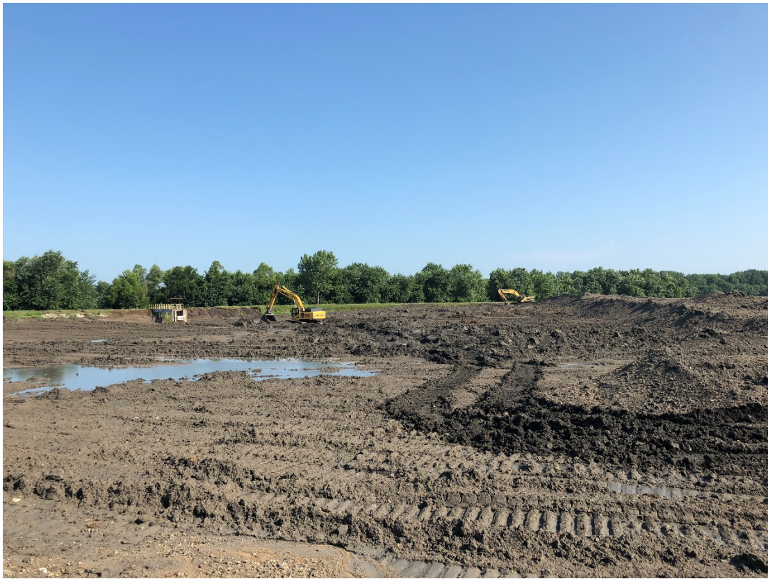
Photograph 5 ▲ - View of fly ash spreading activities at the Fly Ash Pond to facilitate drying, looking northwest.
