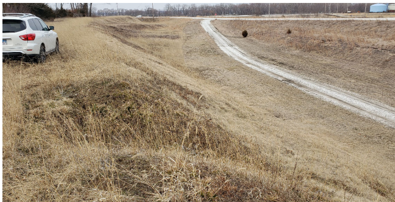
Old East Pond Berm washout
