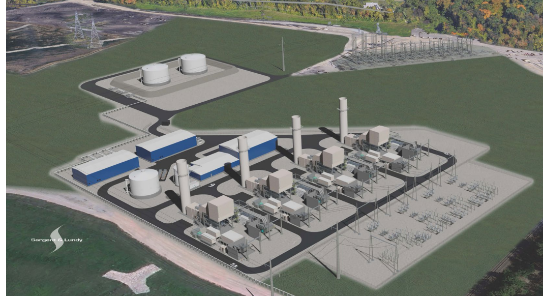
The Castle Bluff Energy Center, an 800-MW natural gas simple-cycle facility, will serve as a backup source of energy, ready to use when customers need it most. It's designed to bolster grid reliability and can be used to deliver energy on the hottest summer days, the coldest winter days or when renewable energy is not generating as forecasted.
