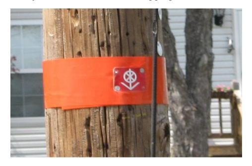
This tag is used for Priority 1 reject poles; red ribbon is also acceptable and wraps around pole twice to avoid fading. This pole will have a job code of RELIP1; once verified that it is a foreign owned pole, it will need to be changed to a RELIJ1.
