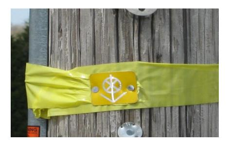
This tag is used for Restorable Poles; wrap ribbon around pole twice to avoid fading (1 piece of steel). This pole will have a job code of RELIP6; once verified that it is a foreign owned pole, it will need to be changed to a RELIJ6.
