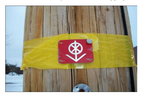
This tag is used for Priority Restorable Reject Poles; wrap ribbon twice around pole to avoid fading (2 pieces of steel). This pole will have a job code of RELIP5; once verified that it is a foreign owned pole, it will need to be changed to a RELIJ5.
