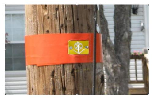
This tag is used for Priority 2 reject poles; red ribbon is also acceptable and wraps around pole twice to avoid fading. This pole will have a job code of RELIP2; once verified that it is a foreign owned pole, it will need to be changed to a RELIJ2.
