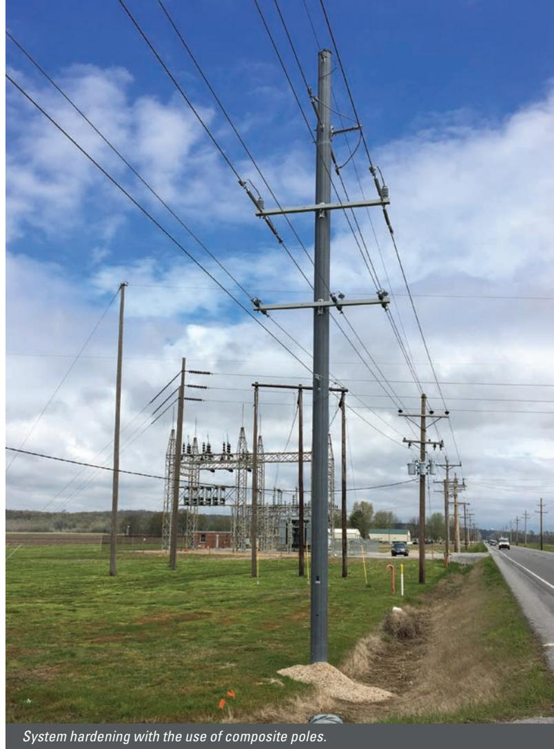
*System hardening with the use of composite poles.*
