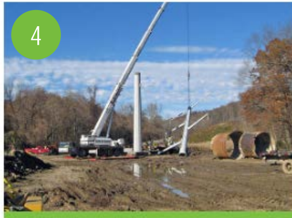
Lift and place structure on foundation
