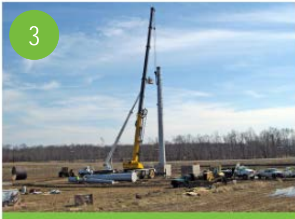
Assemble structure on the ground
