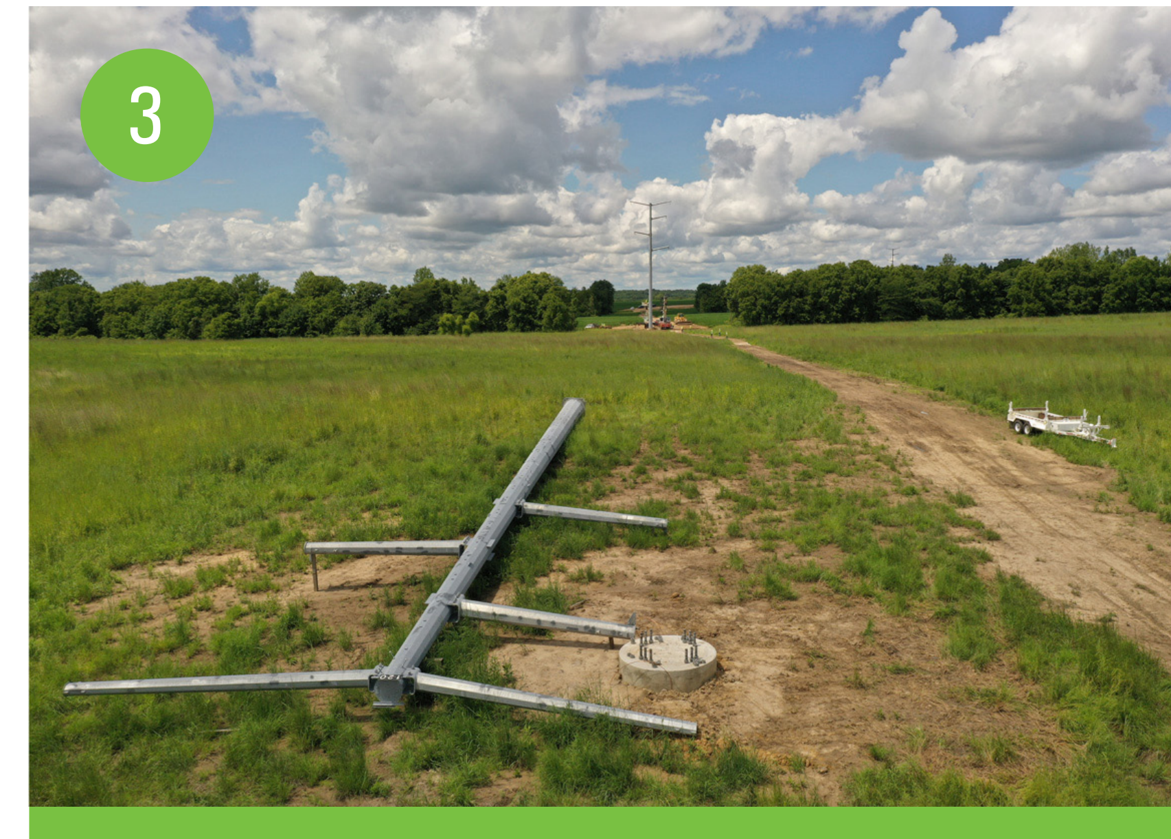
Assemble structure on the ground
