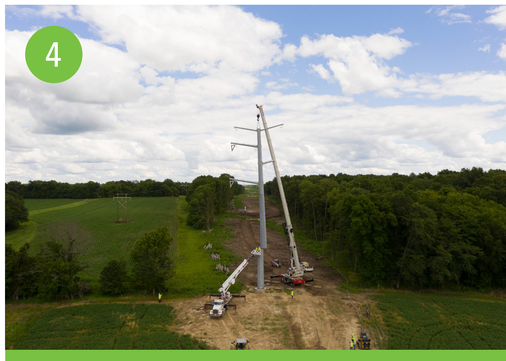
Lift and place structure on foundation
