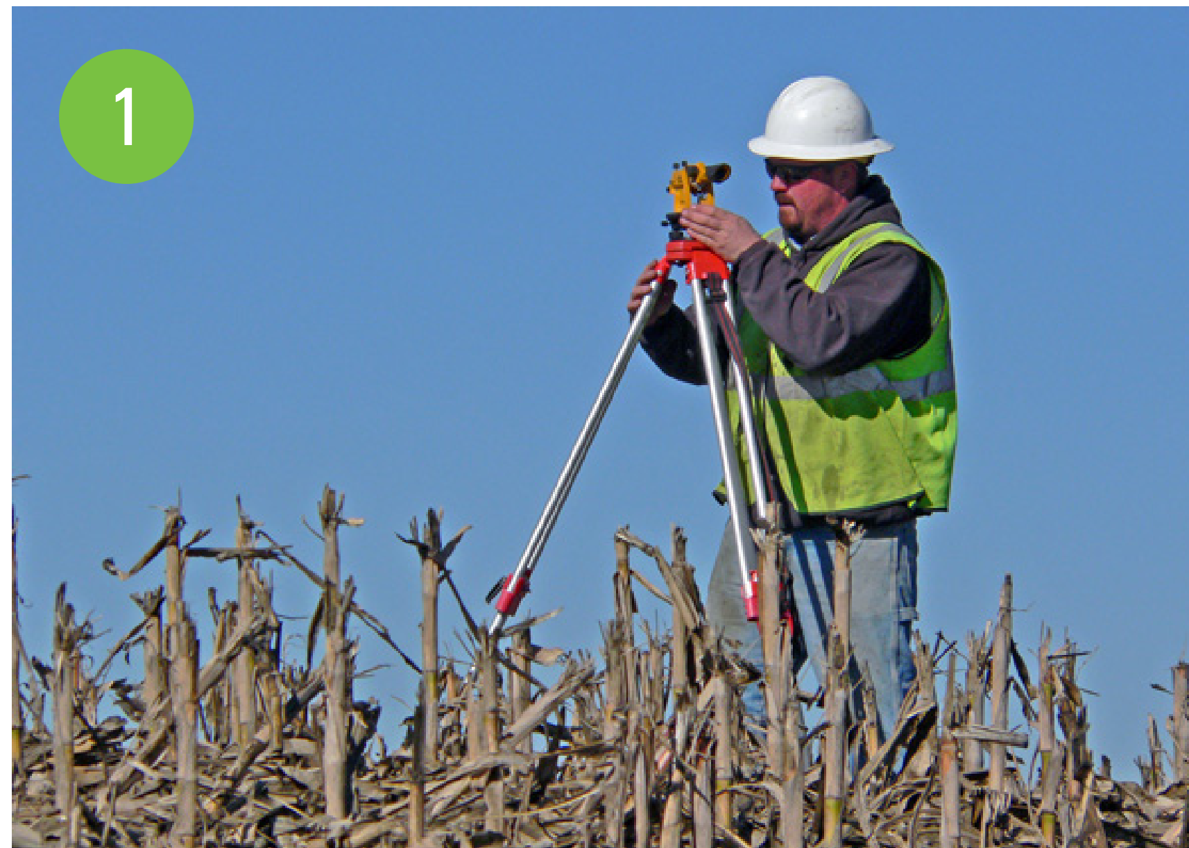
Survey structure locations and vegetation clearing
