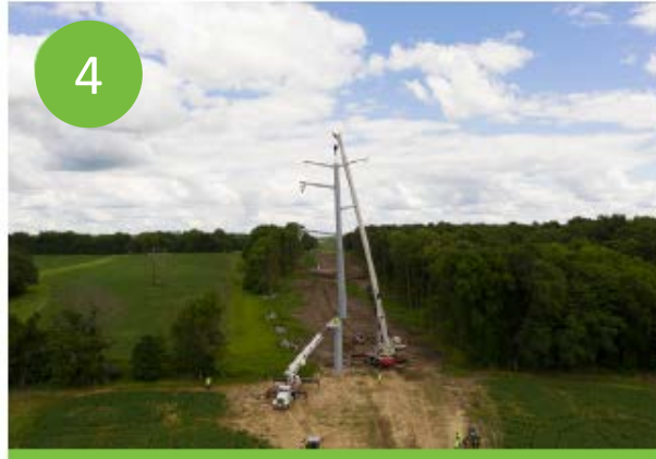
4 Lift and place structure on foundation
