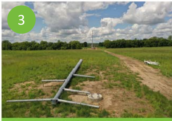
3 Assemble structure on the ground
