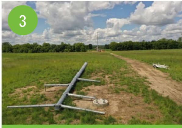
Assemble structure on the ground
