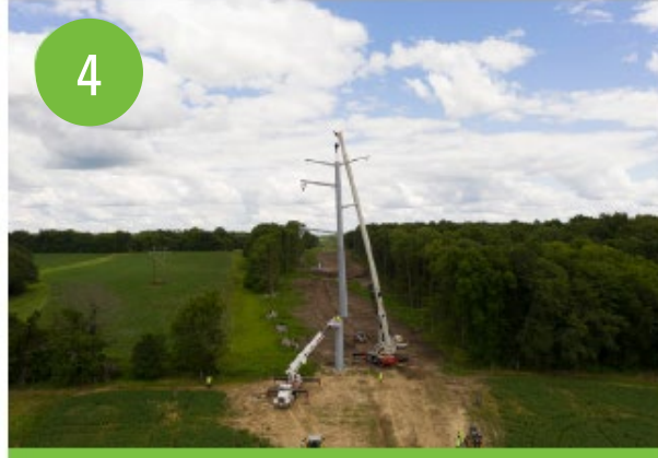
Lift and place structure on foundation
