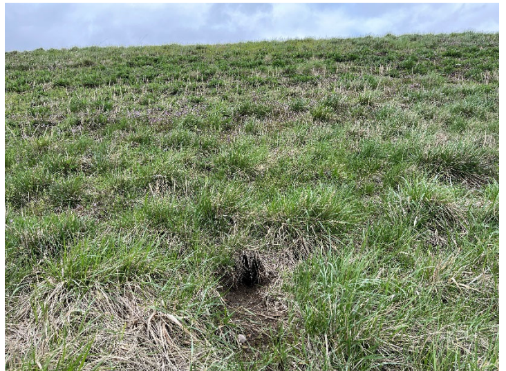
Animal Burrow Observed at Base of Embankment
