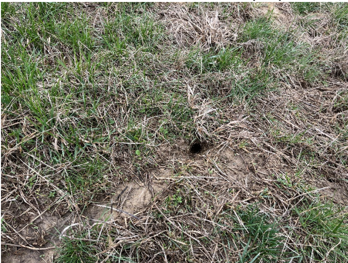
Small Animal Burrow Observed on Cap Top
