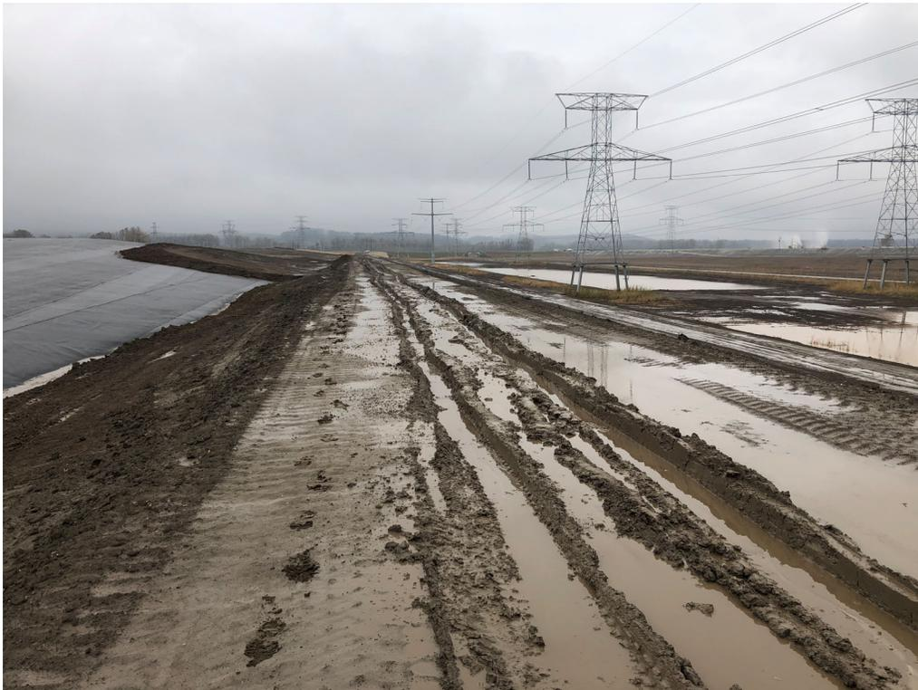
*Figure 2 – LCPB embankment crest with ruts on east side of the impoundment.*
