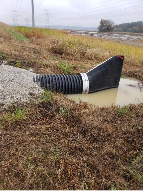
*Figure 9 – There is ponding above the invert of the duckbill valve at Station 21+00.*
