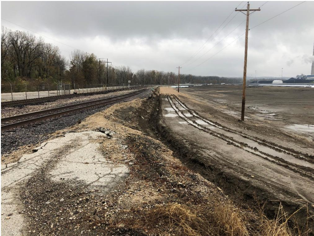
*Figure 4 – Embankment crest on the west side of the impoundment.*
