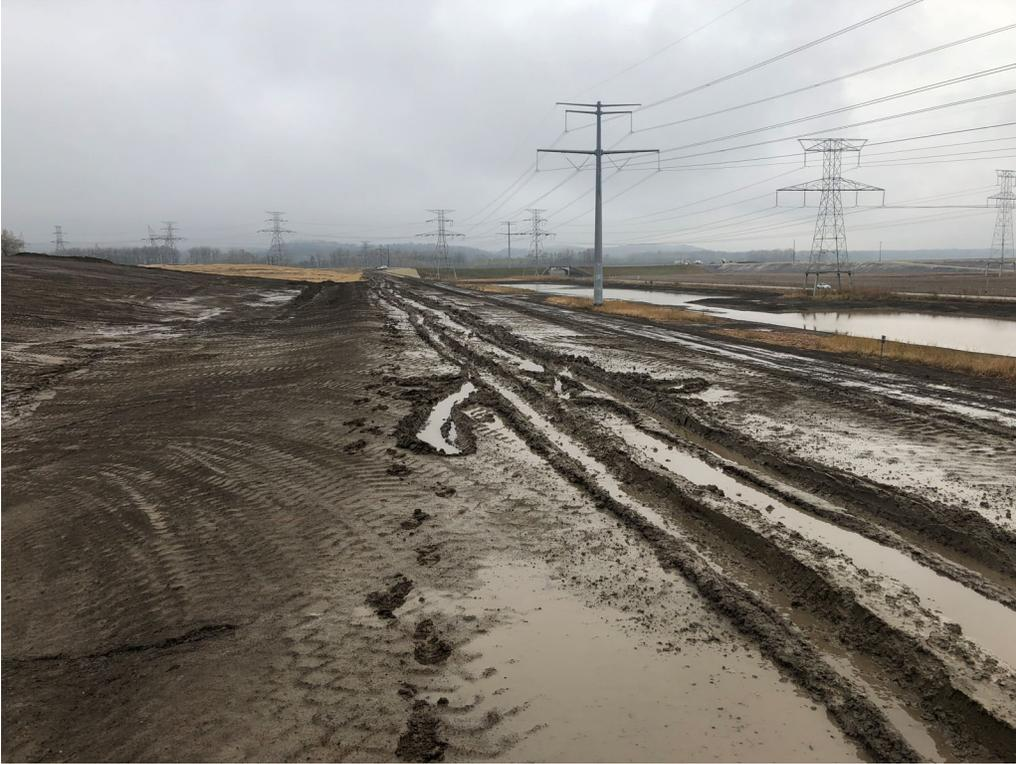
*Figure 3 – LCPB embankment crest with ruts on east side of the impoundment.*
