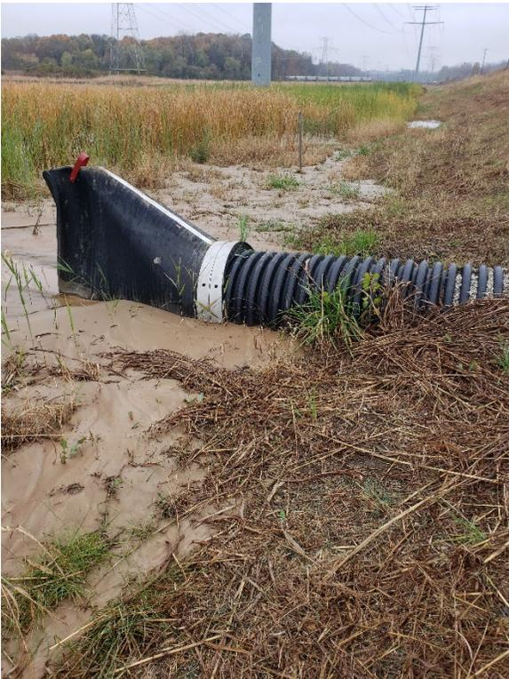
*Figure 8 – The duckbill valve at Station 16+00 is partially buried in sediment.*
