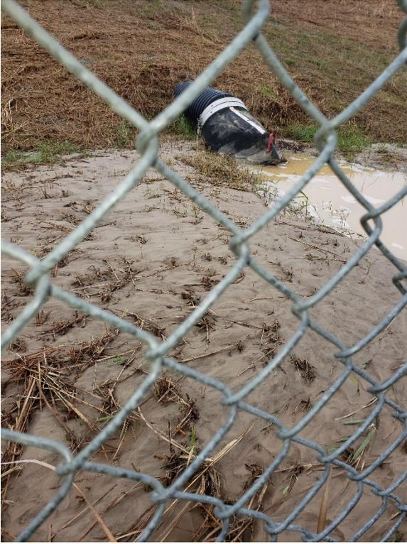
*Figure 7 – Duckbill valve at Station 8+00 is no longer attached.*
