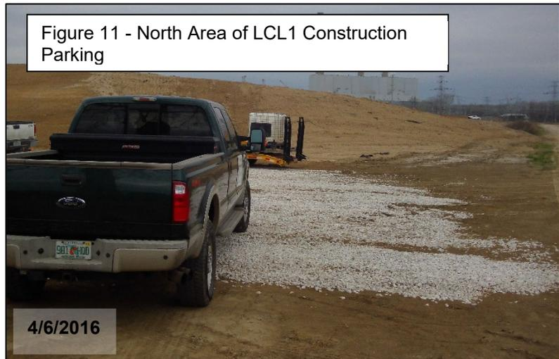
The gravel used for the roadways, under the FCM, and parking lots nearby consists mostly of limestone and dolomite and contains some calcite sourced from nearby quarries. Precipitation and infiltration of surface water through fresh gravel, salting of gravel and road surfaces, and concrete that contains water-soluble salts leach soluble components into the shallow groundwater and can cause an increase in the COIs observed in TMW-2.
