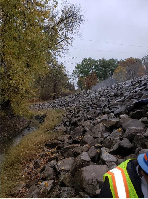
*Figure 7 - Riprap on the downstream perimeter embankment slope.*
