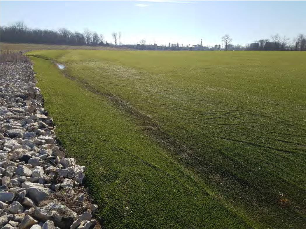
Cap –At Outlet #6 looking Northwest at erosion in ditch beyond toe of berm
