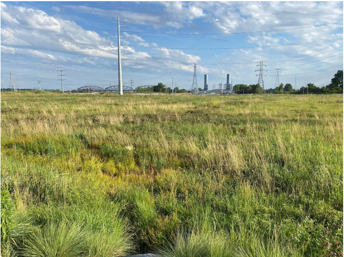
North Pump Station, facing north.
