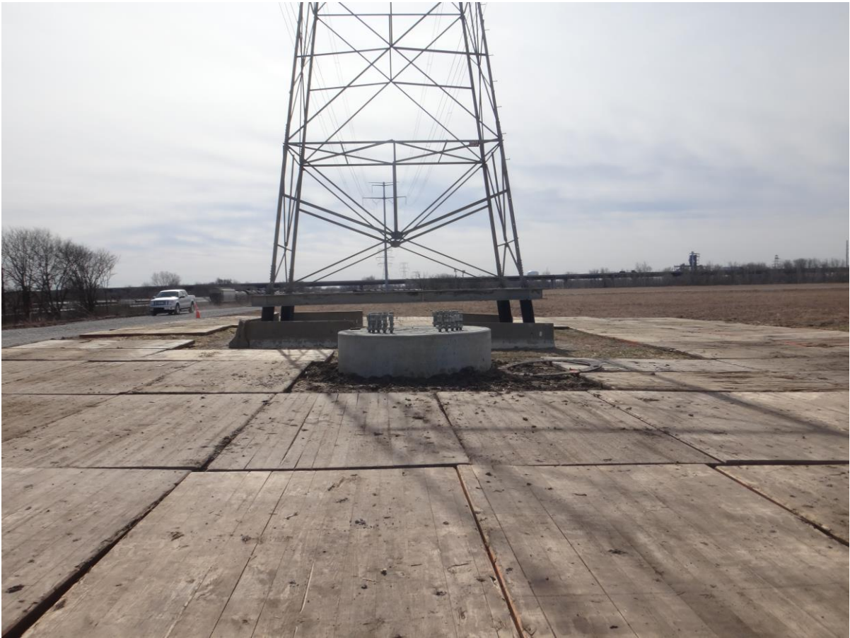
The fall construction for the foundation for the replacement of Structure 161 was completed and the flexible membrane is no longer exposed.
