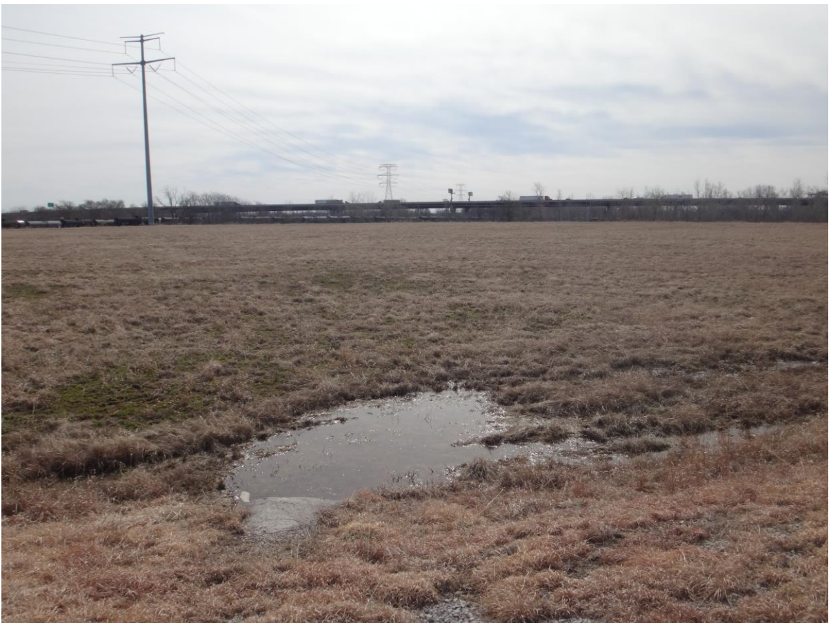
South Pump Station, facing south.
