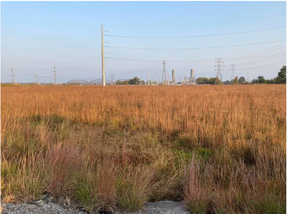
North Pump Station, facing north.
