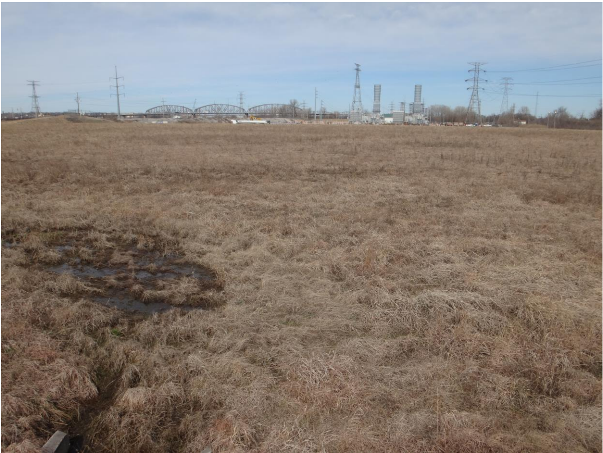
North Pump Station, facing north.
