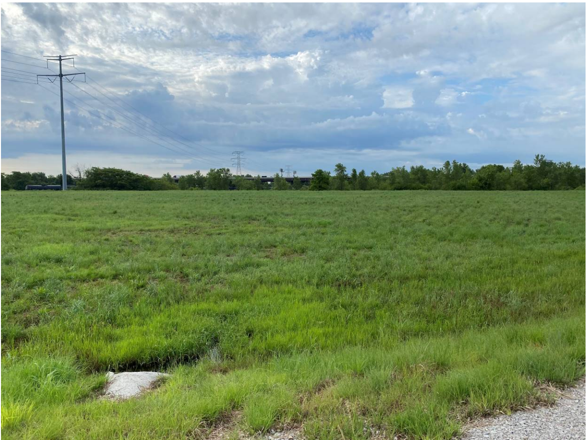
South Pump Station, facing south.
