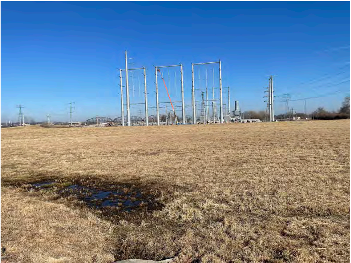
North Pump Station, facing north.
