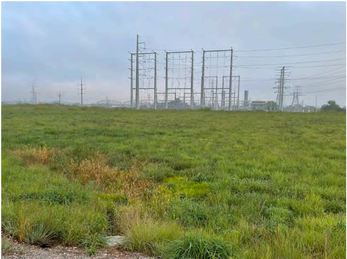
North Pump Station, facing north.
