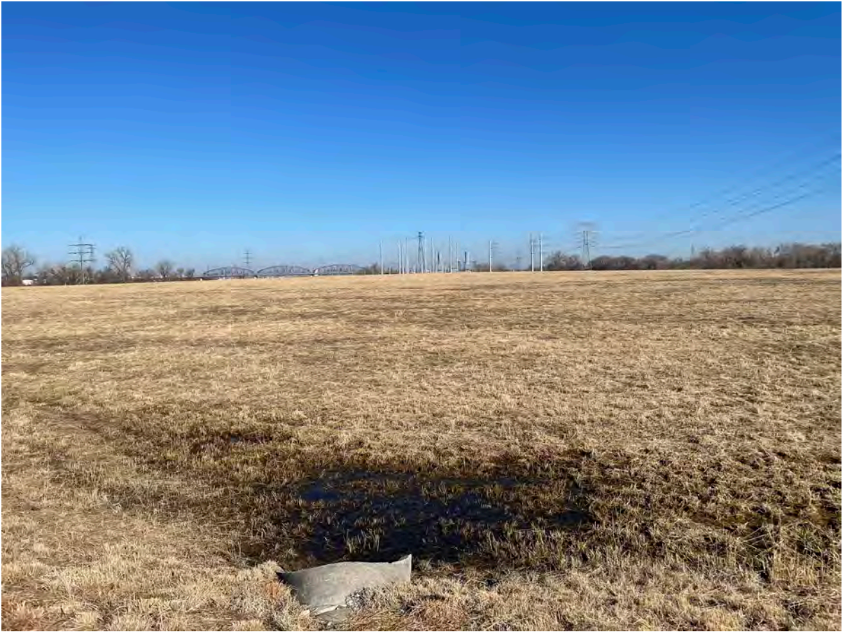
South Pump Station, facing north.
