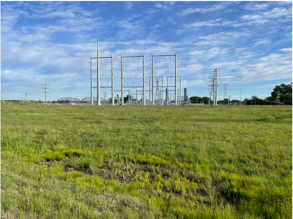
North Pump Station, facing north.
