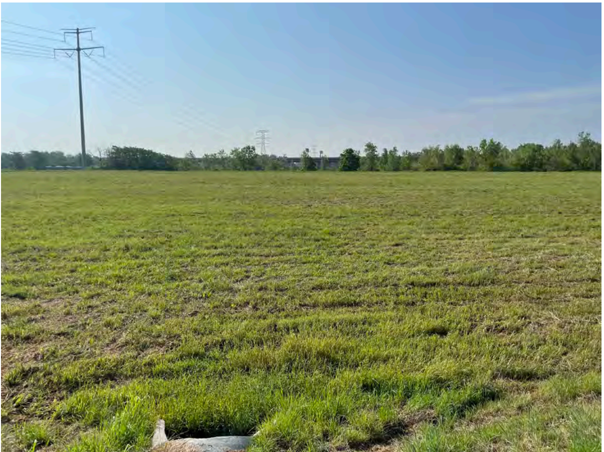
South Pump Station, facing south.
