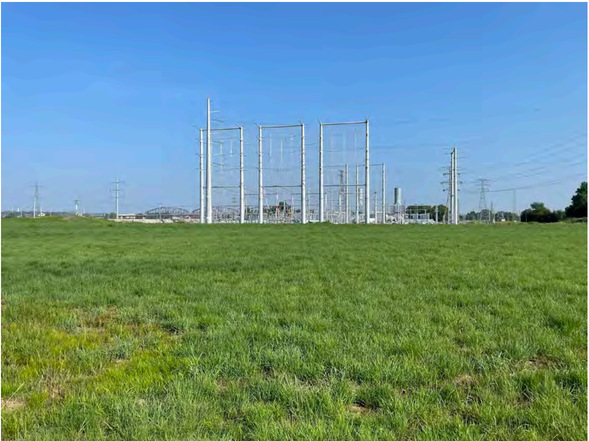
North Pump Station, facing north.
