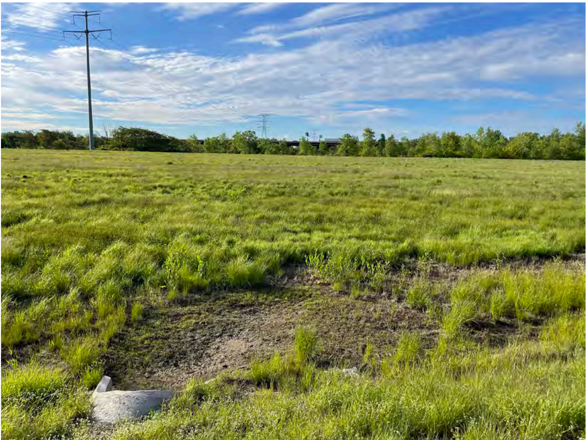
South Pump Station, facing south.
