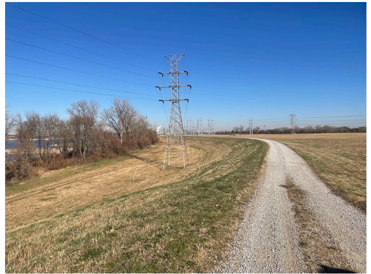
River (West) Embankment – center section
