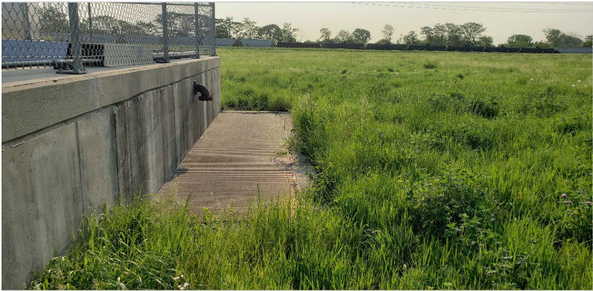
Grating of North Pumps station.
