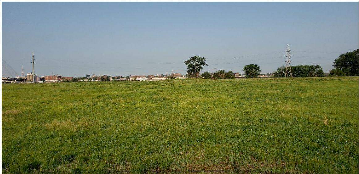
South Pump Station, facing south.
