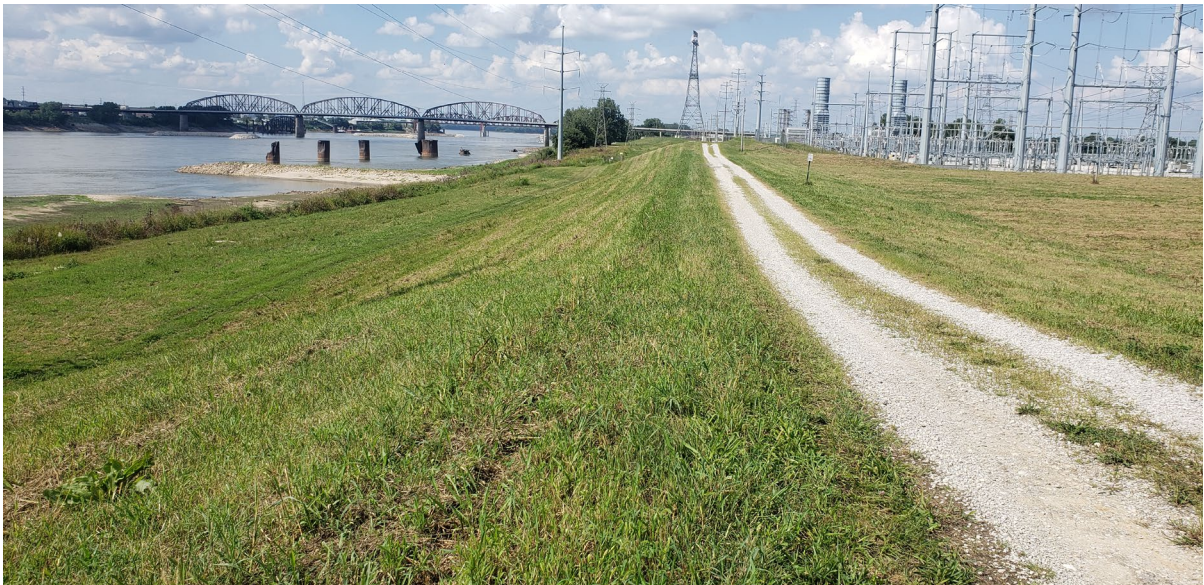
River (West) Embankment – NW section
