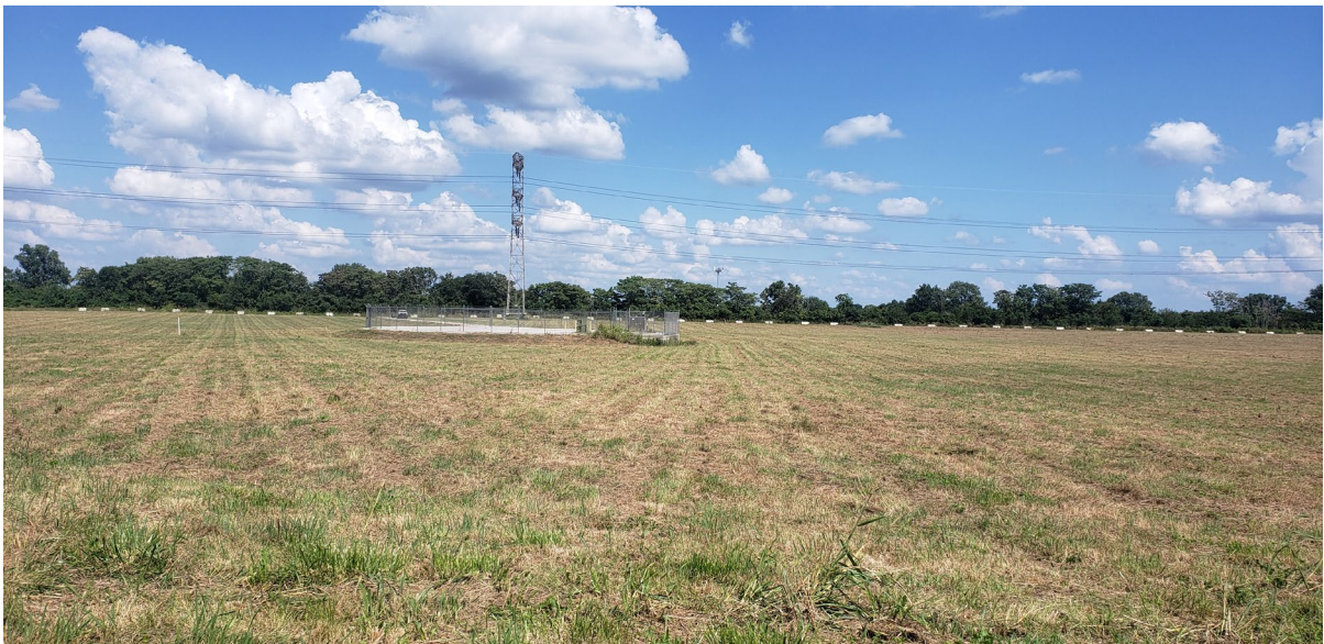
North Pump Station, facing east
