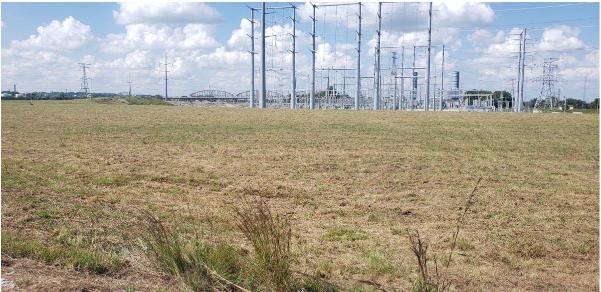
North Pump Station, facing north
