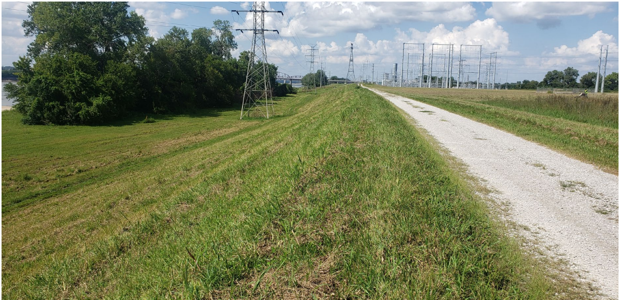
River (West) Embankment – center section
