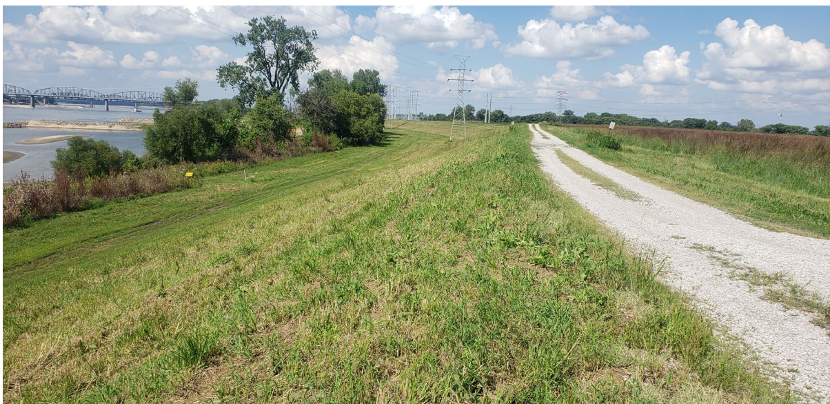
River (West) Embankment – SW section
