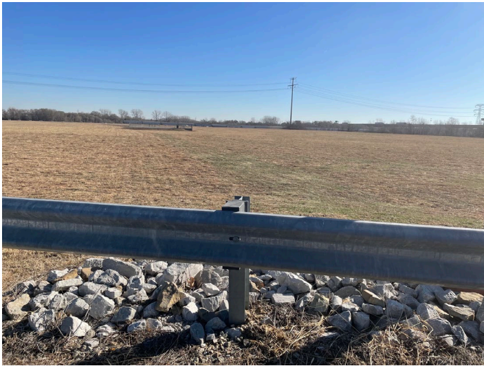
South Pump Station, facing east
