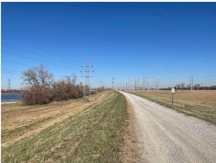
River (West) Embankment – NW section
