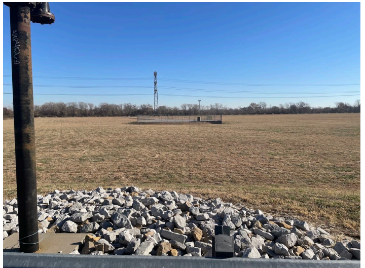
North Pump Station, facing east
