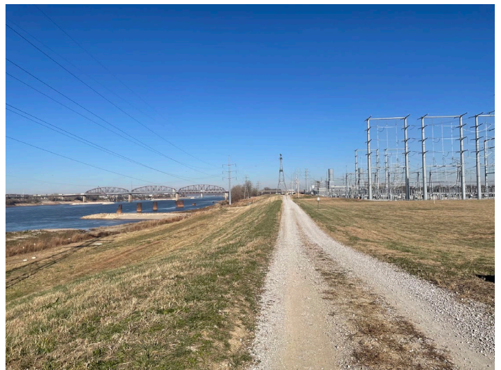
River (West) Embankment – Very Northern most section
