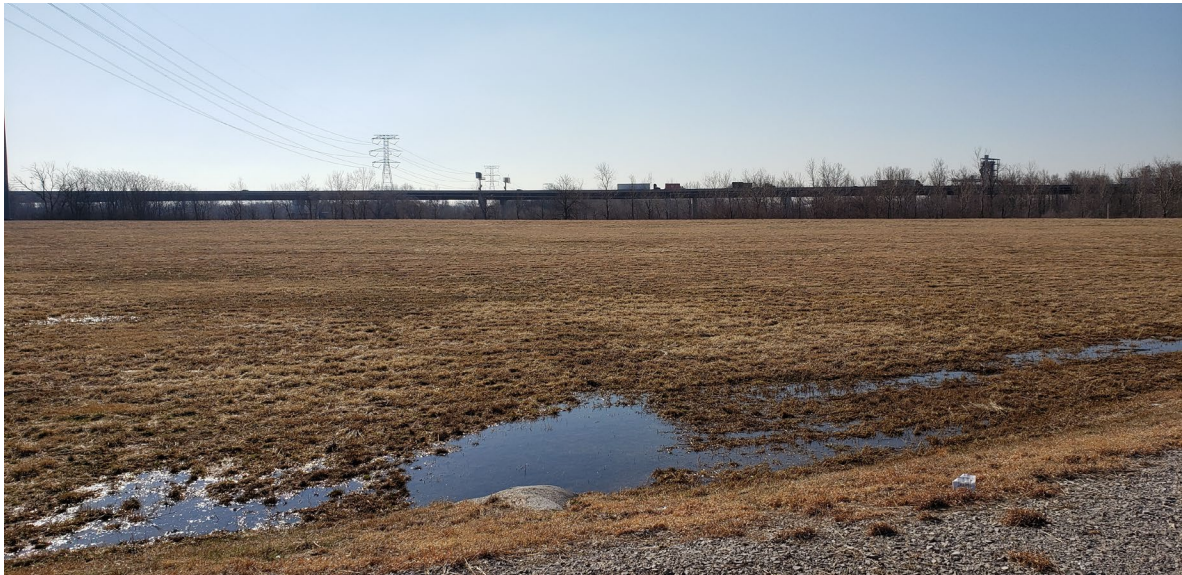
South Pump Station, facing south.
