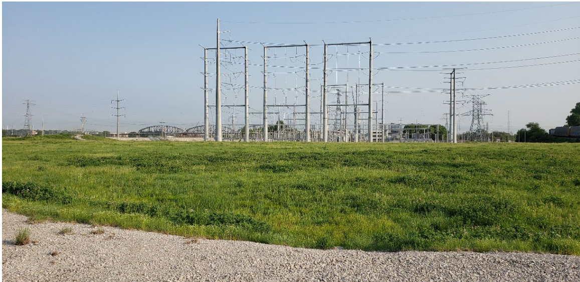
North Pump Station, facing north.
