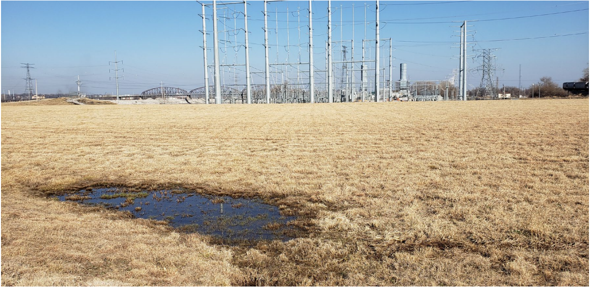
North Pump Station, facing north.
