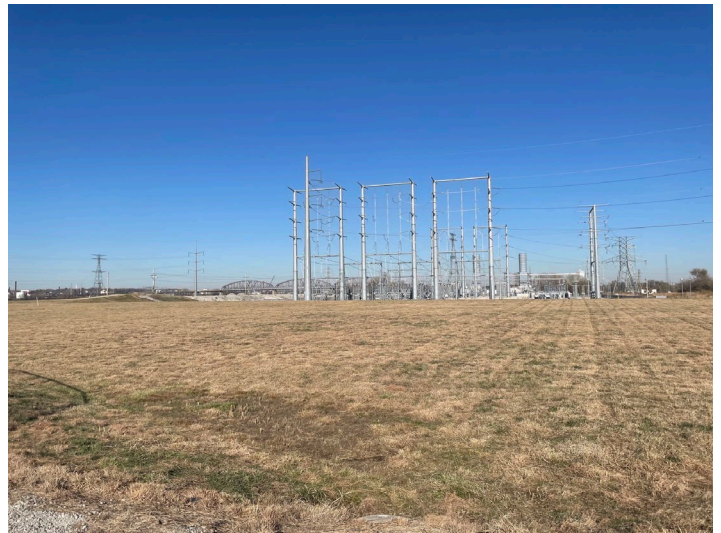
North Pump Station, facing north
