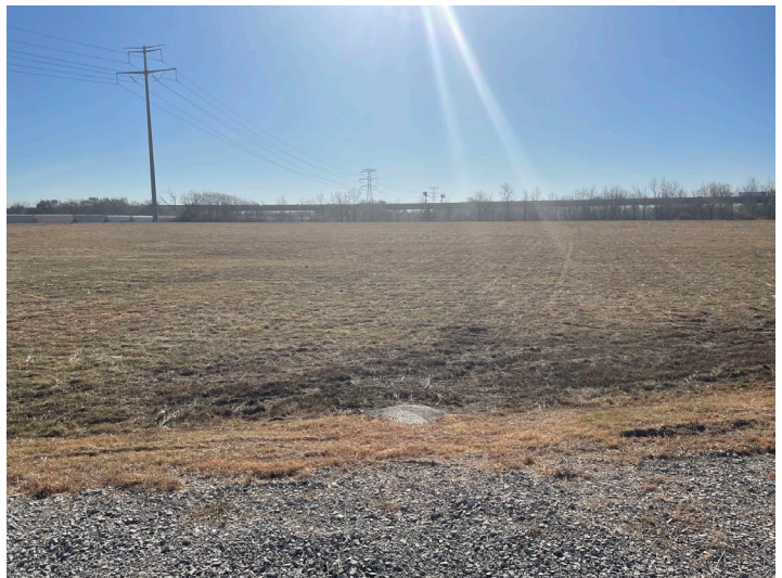
South Pump Station, facing south
