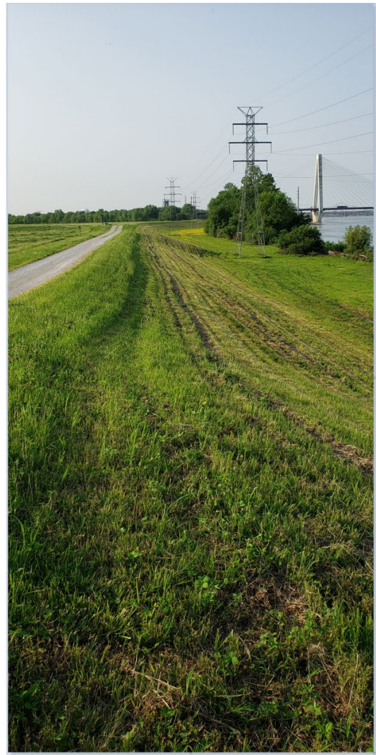
River Side Berm
