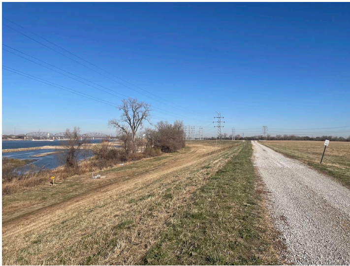
River (West) Embankment – SW section
