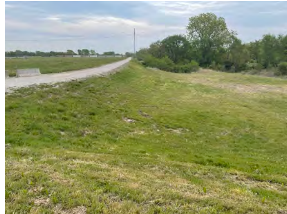
South Embankment, facing east
