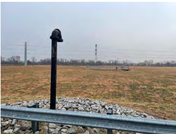
North Pump station, facing east
