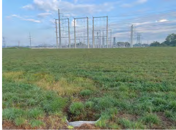
North Pump Station, facing north
