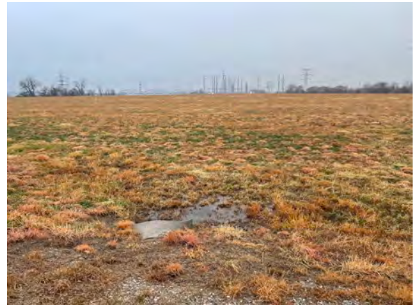
South Pump Station, facing north
