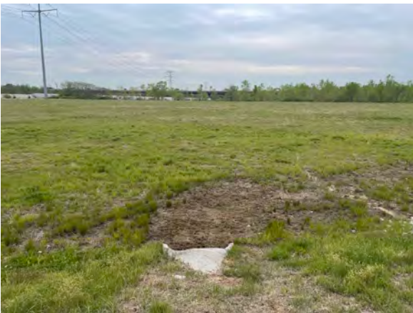
South Pump Station, facing south
