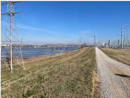
West Embankment, north section
