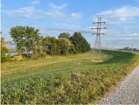
West Embankment, south section
