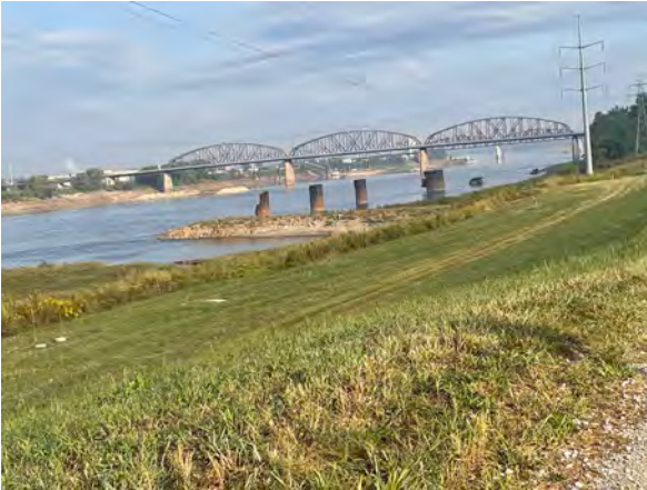
West Embankment, north section
