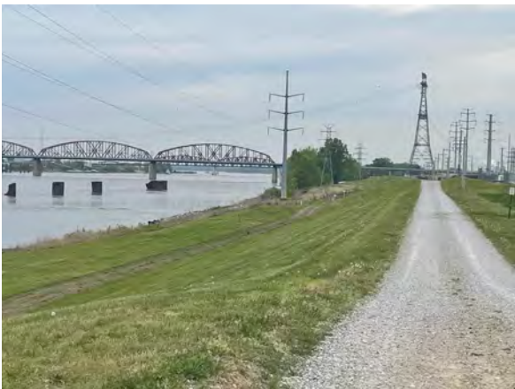
West Embankment, north section
