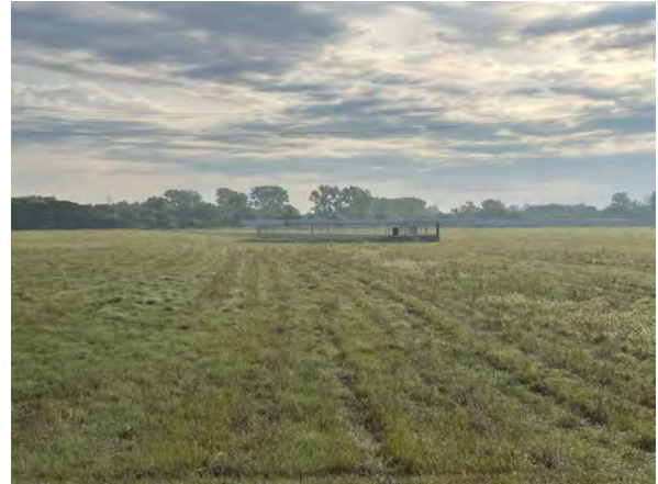
South Pump station, facing east
