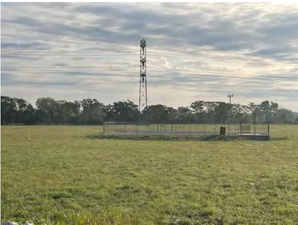
North Pump station, facing east
