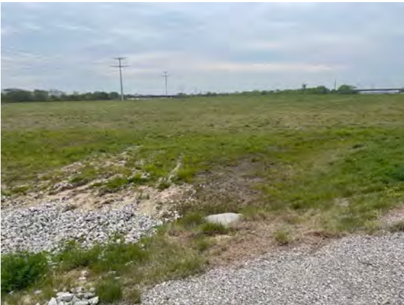
North Pump Station, facing south
