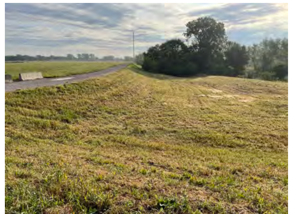
South Embankment, facing east
