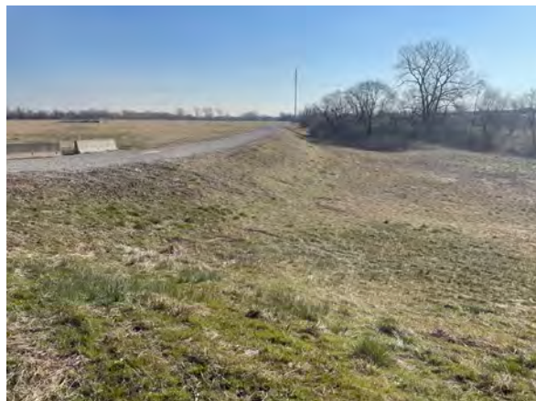
South Embankment, facing east
