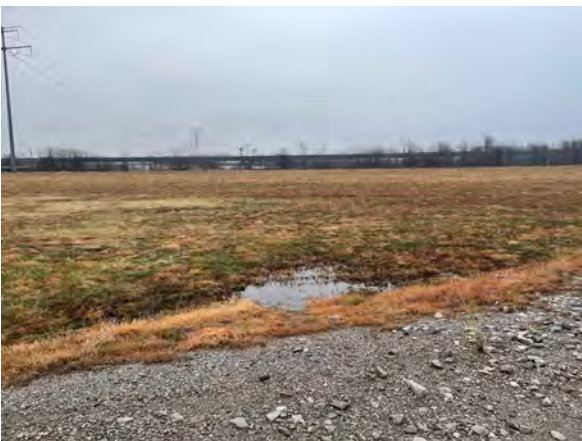
South Pump Station, facing south
