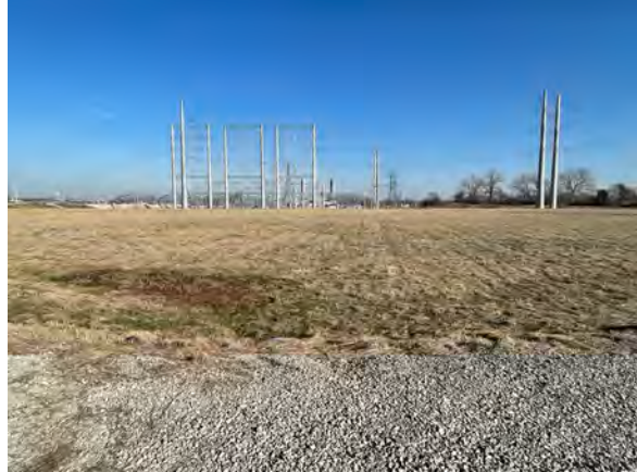
North Pump Station, facing north
