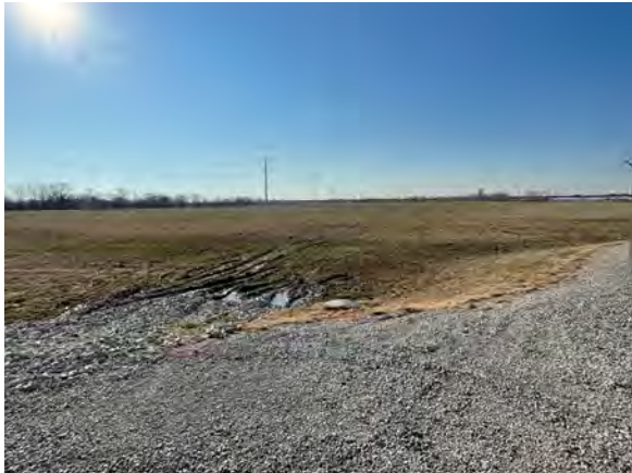
North Pump Station, facing south
