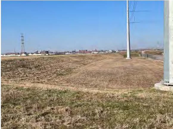
North embankment, facing west
