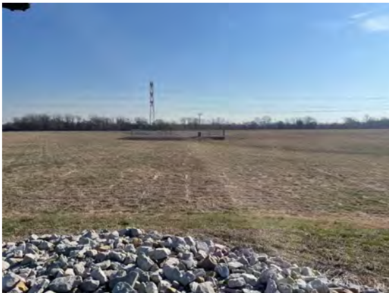
North Pump station, facing east
