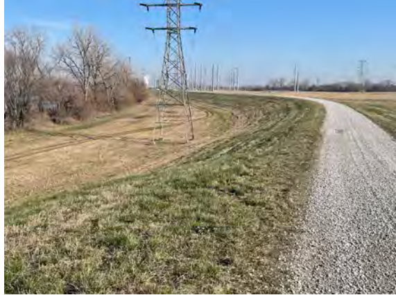
West Embankment, center section
