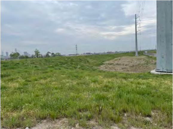
North embankment, facing west
