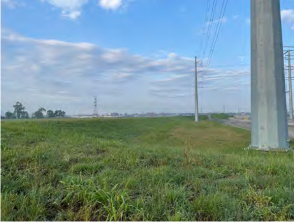
North embankment, facing west
