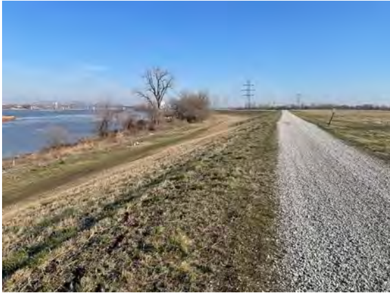
West Embankment, south section
