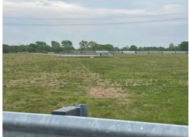
South Pump station, facing east
