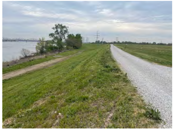
West Embankment, center section
