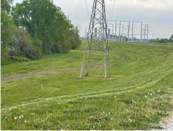
West Embankment, south section
