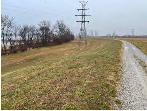
West Embankment, south section
