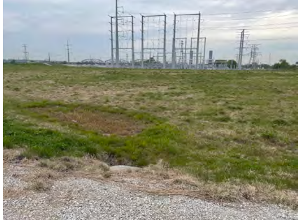
North Pump Station, facing north
