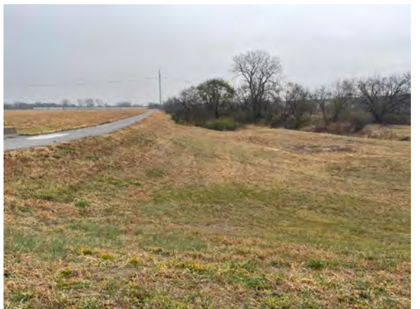
South Embankment, facing east
