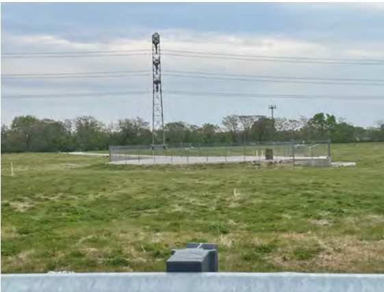
North Pump station, facing east
