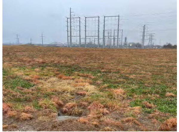
North Pump Station, facing north
