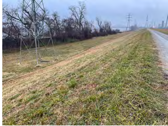
West Embankment, center section
