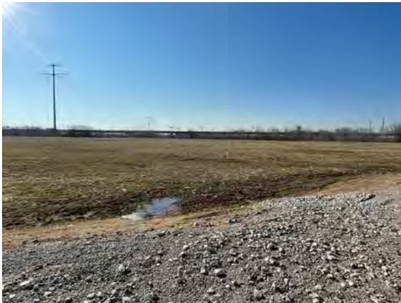
South Pump Station, facing south
