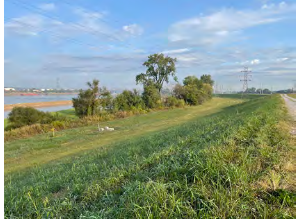
West Embankment, center section
