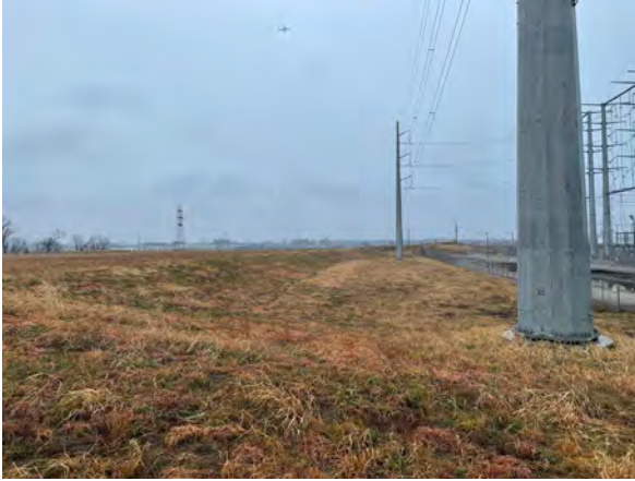
North embankment, facing west
