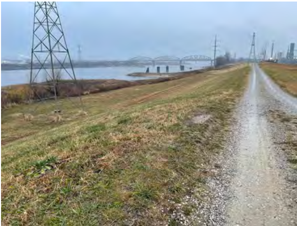
West Embankment, north section
