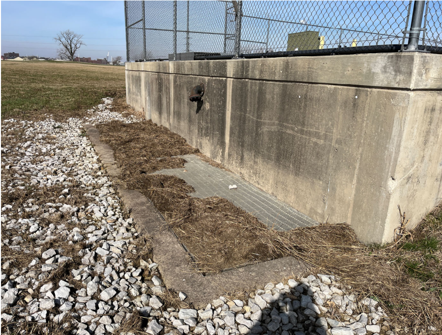
Buildup of grass clippings on grate at south pump station
