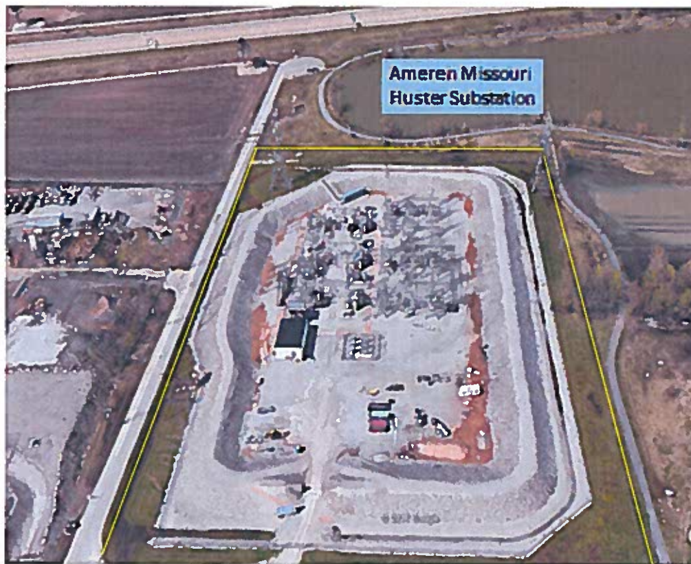
Figure 2 - Huster Substation Perimeter
