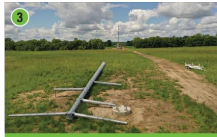
Assemble structure on the ground
