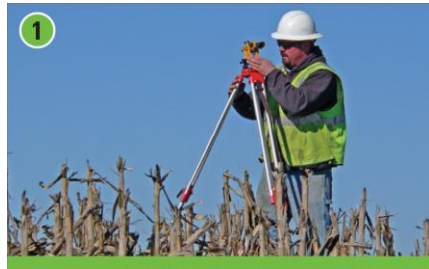
Survey structure locations, soil borings and vegetation clearing
