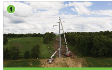
Lift and place structure on foundation
