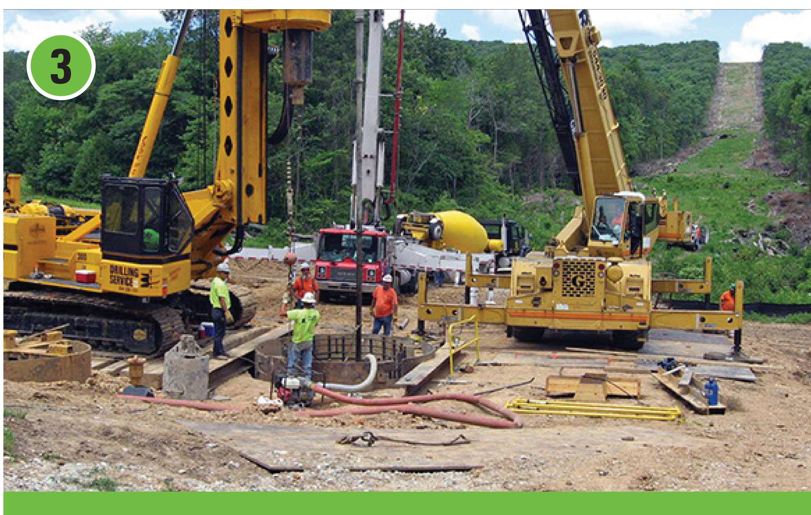
Dig structure holes
