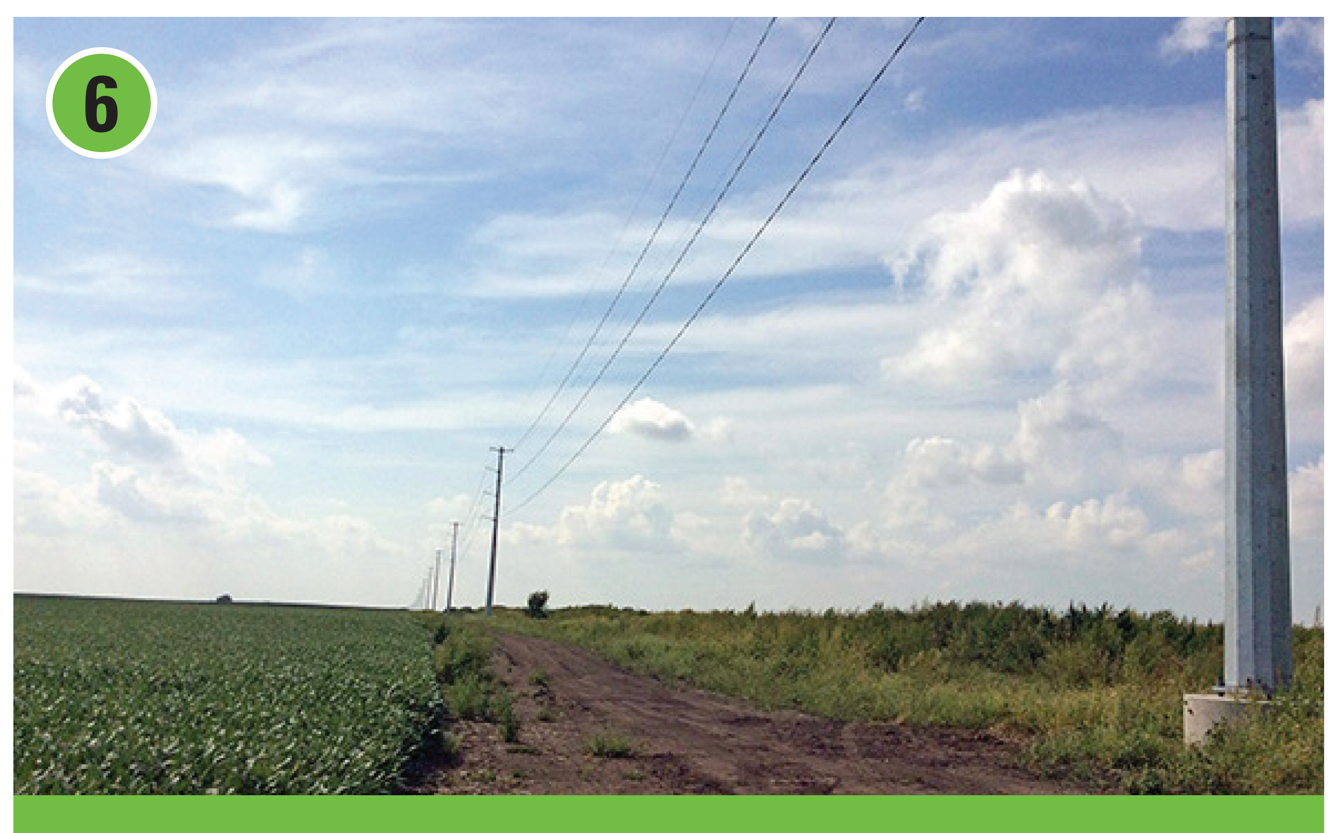
Energize line and restore easement
