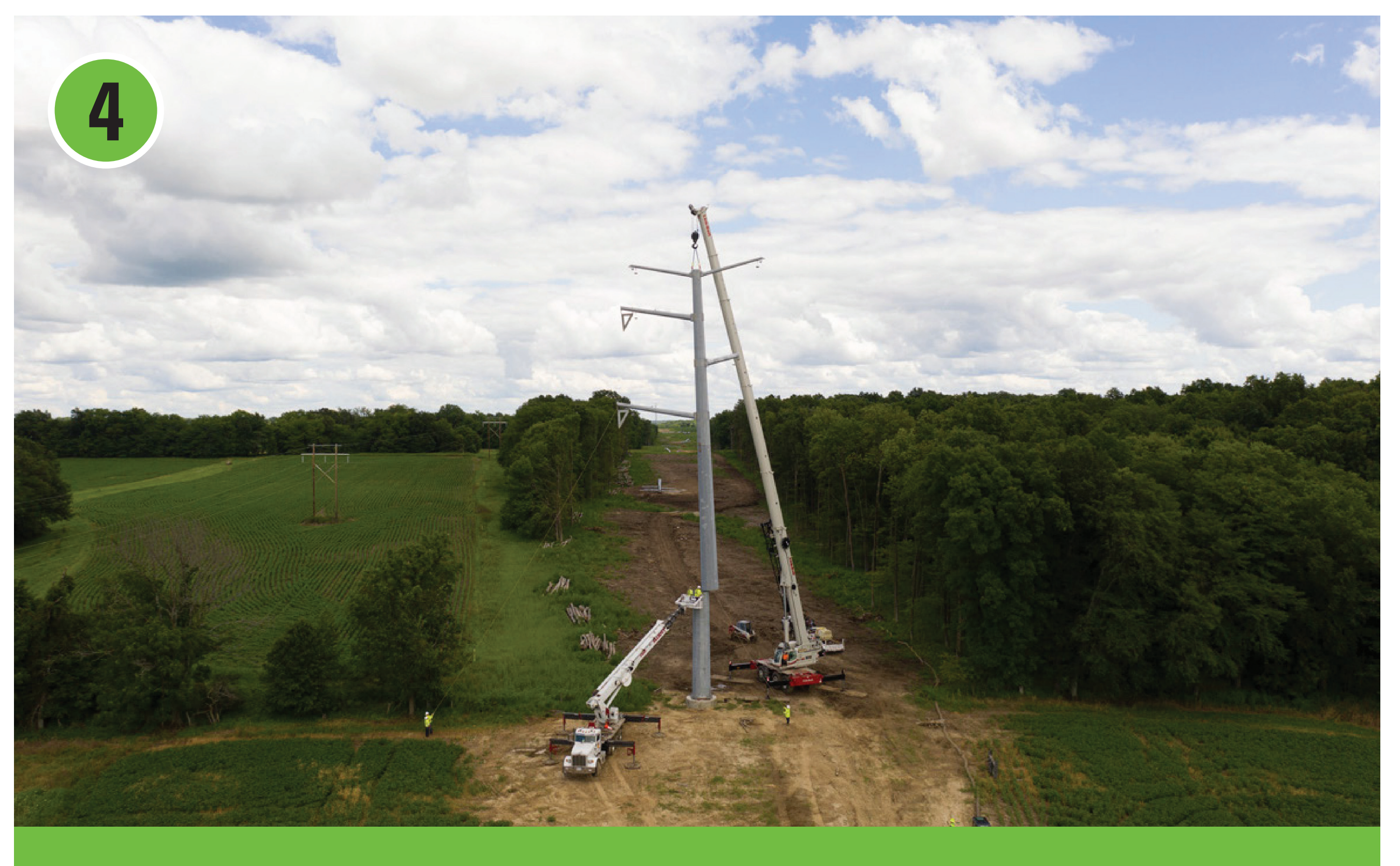
Lift structure into hole and backfill with concrete
