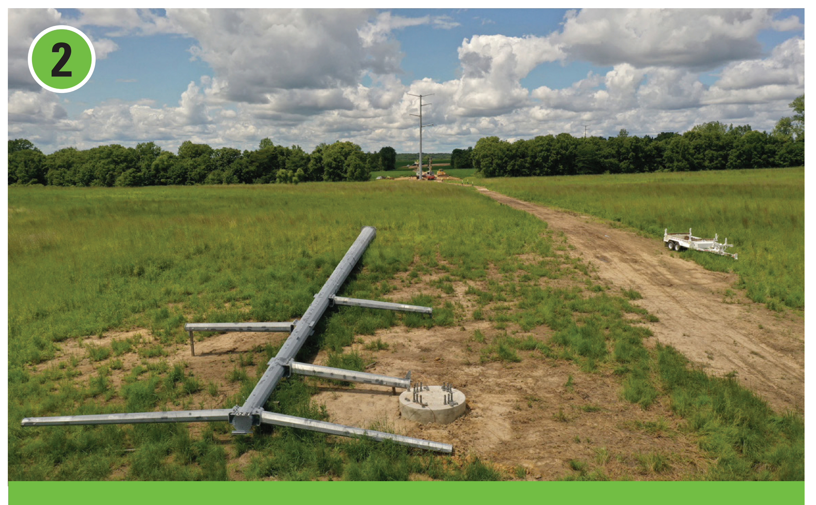
Assemble structure on the ground
