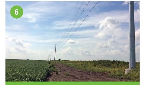
Restore easement and energize line
