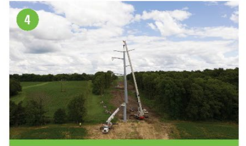
Lift and place structure on foundation
