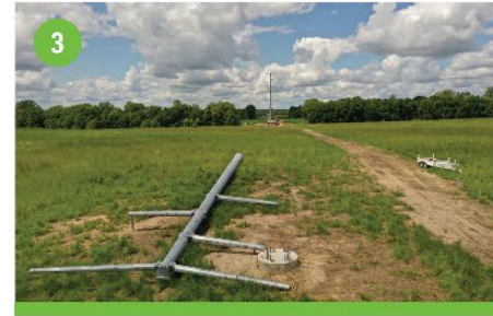
Assemble structure on the ground
