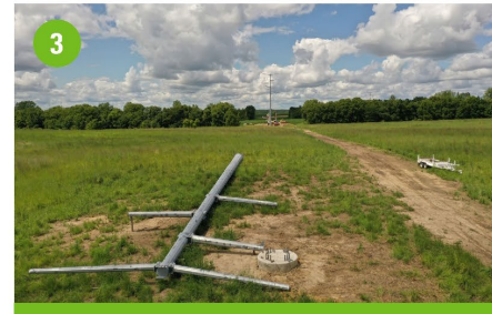
3 Assemble structure on the ground
