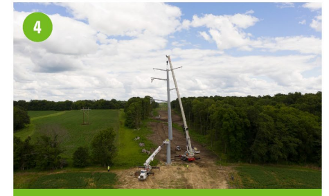
4 Lift and place structure
