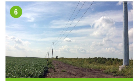
6 Restore easement corridor, energize line and remove temporary access
