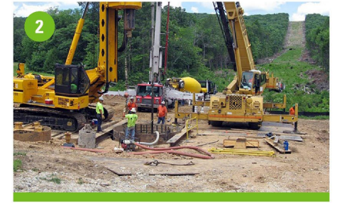
2 Drill hole and pour foundation, as needed
