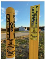
Most pipelines are buried underground. High-visibility markers identify the approximate location of major pipelines in the area and highlight the need for extra care. For
