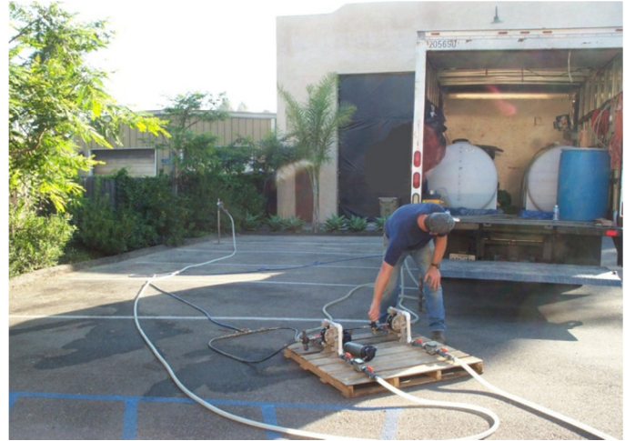
Above: Chemical oxidant pumped from storage tanks to injection point location.
