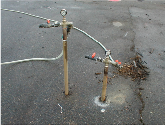
Above: Example of an ISCO injection point location.
