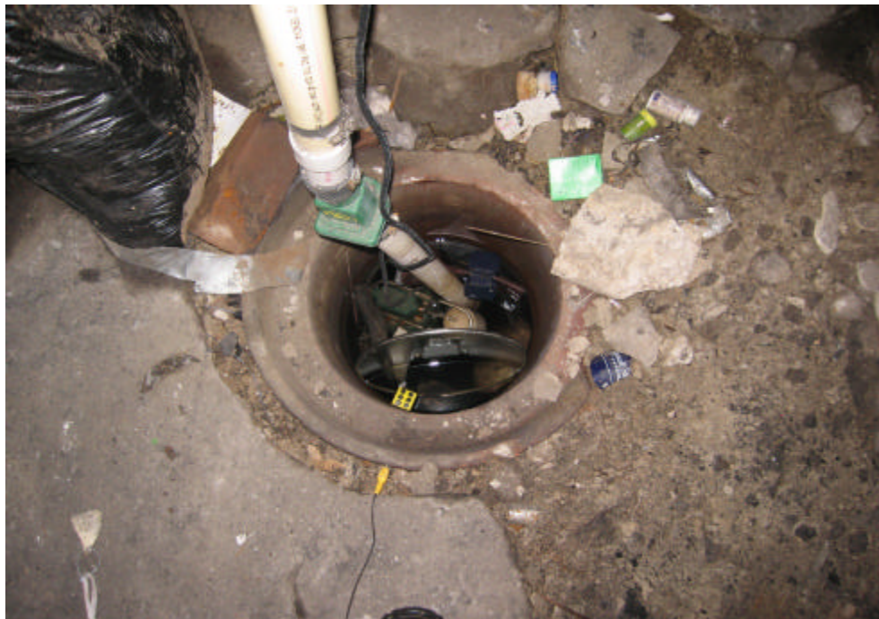
PHOTO 12: Inside basement of 507 E. Washington looking at water in swamp. Note broken concrete floor slab and exposed soil.
