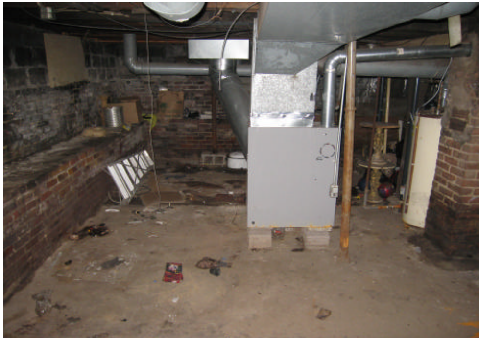
PHOTO 10: Inside basement of 507 E. Washington looking east along north wall. Note new central heating unit and water heater, both fueled by natural gas.
