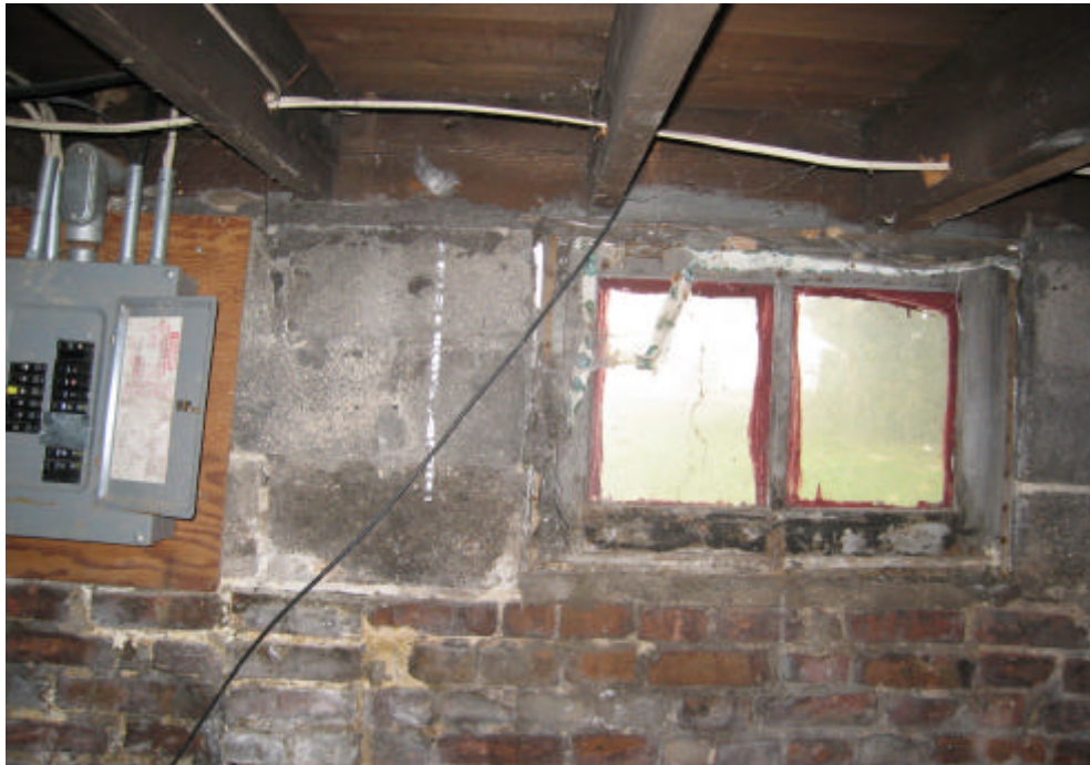
PHOTO 15: View of window along south wall of basement. There are several gaps between window frame and bricks & cinder blocks in this area and throughout basement.
