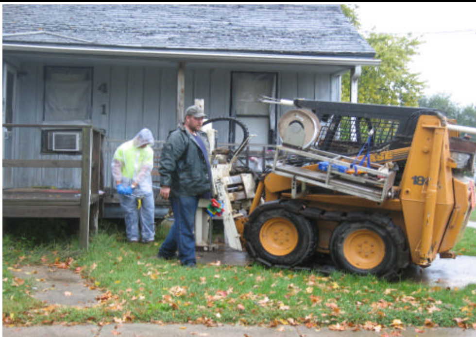
PHOTO 6: View to north at VP412EHill-3 location. Note plywood under Geoprobe rig.
