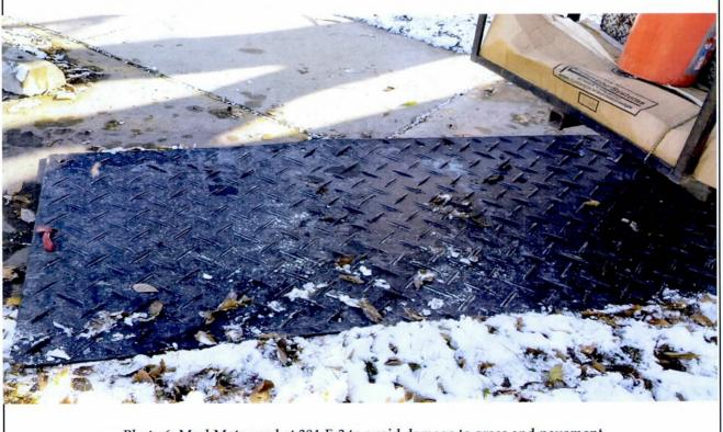
Photo 6: Mud Mats used at 304-E-3 to avoid damage to grass and pavement
