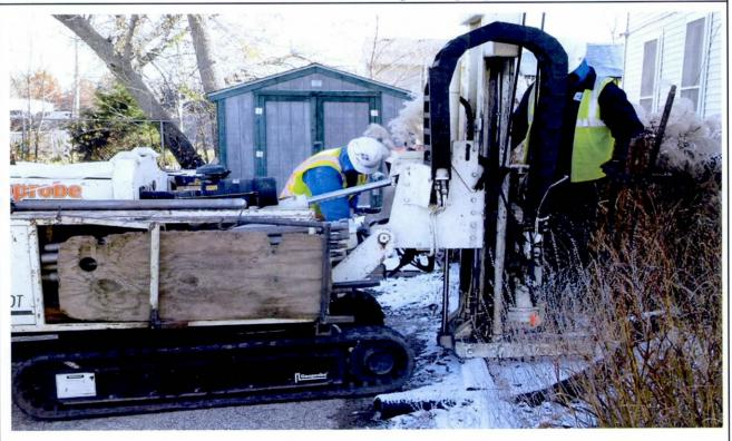
Photo 18: 508-N-8 Boring Installation
