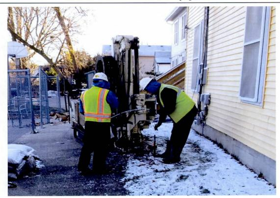
Photo 13: 506-N-6 Boring Installation
