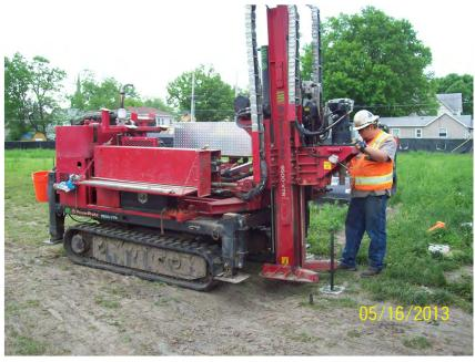
Above: DPT installation of injection locations – two screen depths per location.
