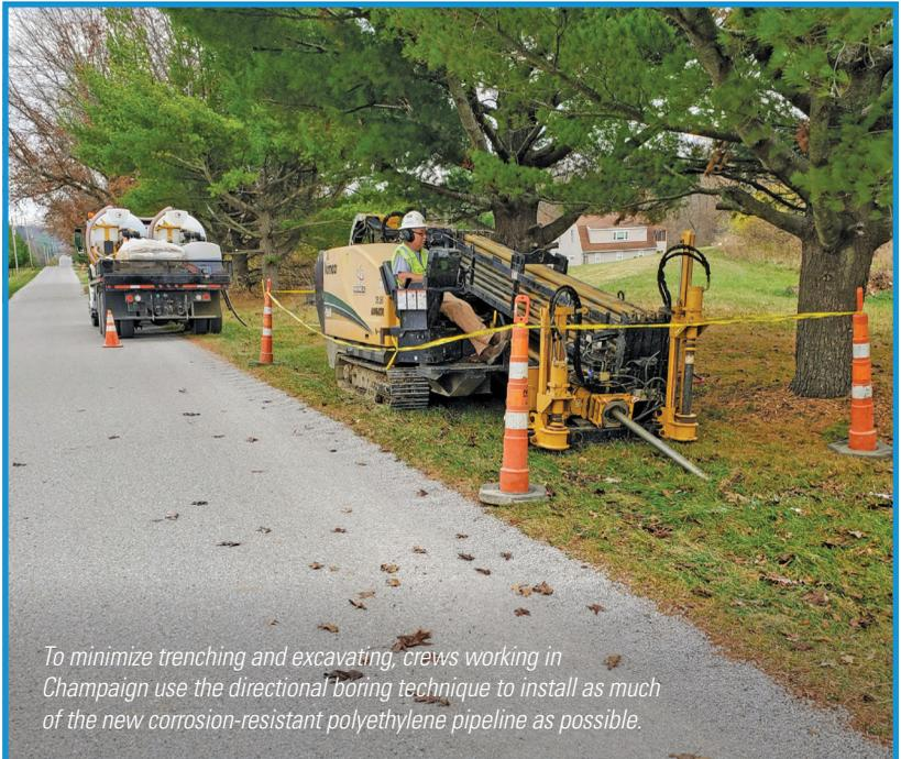
*To minimize trenching and excavating, crews working in Champaign use the directional boring technique to install as much of the new corrosion-resistant polyethylene pipeline as possible.*
