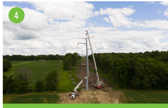
Lift and place structure on foundation
