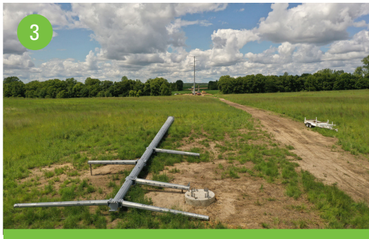
Assemble structure on the ground
