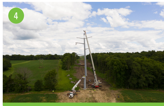
Lift and place structure on foundation
