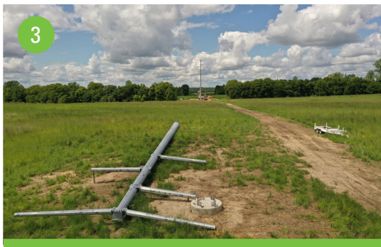
Assemble structure on the ground
