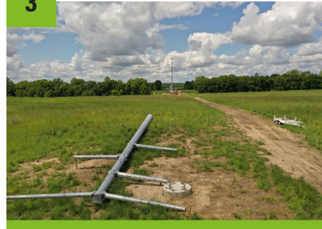
Assemble structure on the ground
