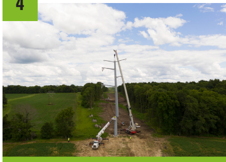
Lift and place structure on foundation
