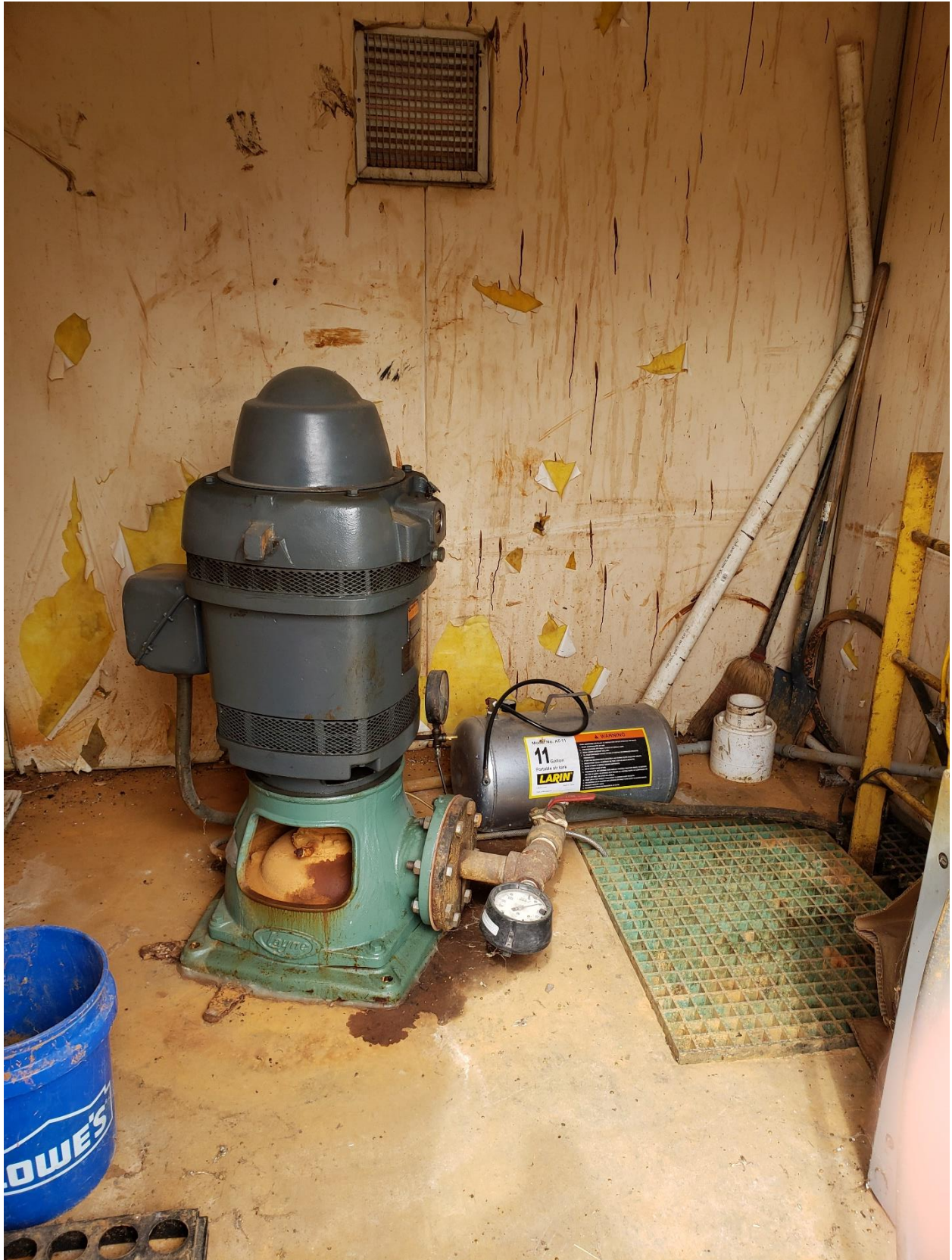
Figure 1 – Overflow Pump
