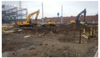
The project work involves excavation of an expected 27,280 tons of material from the Tower Area and an expected 147,060 tons of material from the Phase 3 Area. Considering these depths typically are 20 feet or greater from the existing ground surface, excavation will require the installation of perimeter excavation support systems that will be installed by Goettle.
