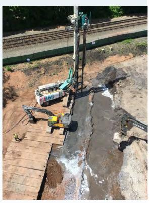
multi-auger soil mixing rigs that are most commonly used to install linear elements, such as cutoff walls or shear panels. DSM auger configurations are specific to each contractor, but typically include 3 or 4 relatively small (3' to 4') diameter augers spaced evenly apart.
