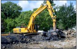
support in-situ solidification (ISS) operations. ISS of approximately 43,500 CY of contaminated soils. Placement of imported backfill material. Collection, testing, and disposal of MGP-impacted storm water. Scope of work also included installation of an eight-inch-thick aggregate layer earthen/asphalt cap. Site restoration activities include installing signage, fencing, and new asphalt/concrete surfaces, as well as placing topsoil and seeds for vegetative regrowth.
