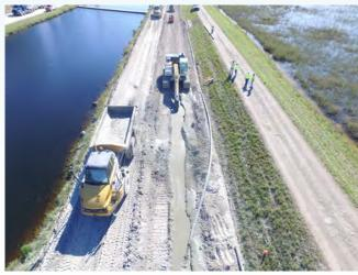
ground. Mixing is usually accomplished using an excavator, much the same as for an SB wall. Backfill can also be placed with the excavator.
