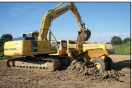
and offsite T+D of ~216,000 tons of MGP impacted soil. Also includes ISS of ~83,000 CY of MGP-impacted soils via bucket mixing, 65% within TFS. Restoration activities will include storm sewer replacement, waterline installation, paving, and the replacement of concrete gutters, sidewalks, and aprons.
