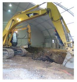
Several structures resided on the former MGP Site footprint including one office building and five duplex residential units. The slide rail excavation support system was utilized to protect the integrity and stability of the structures during excavation activities.
