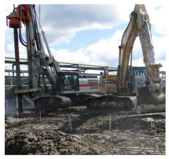
Logistical challenges included site access constraints including height restrictions and site access bridge weight restrictions for equipment, ISS around pile cap locations to maximize the amount of impacted soil remediated via ISS, ISS nearby overhead utilities including pipe racks, and sequencing of ISS to support drill rig stability during mixing.
