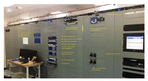
Access to SCADA and Relay control functionality to enable evaluation, monitoring, and controls of energized SG devices with the ability to collect, monitor, and record all nonproduction network control traffic between two devices via a network tap. (B)
