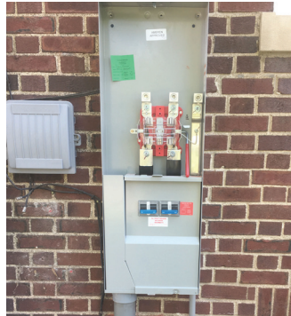
400 Amp With Breaker Safety Lever Bypass
