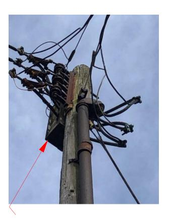
Elevated (bird cage) CT Metering On a Meter Pole
