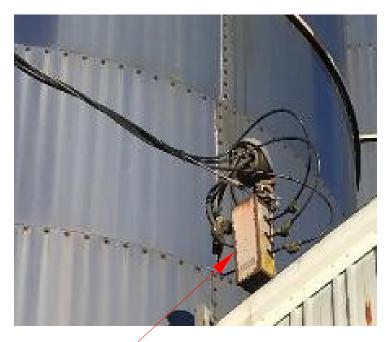
Elevated (bird cage) CT Metering On Service Riser Mast
