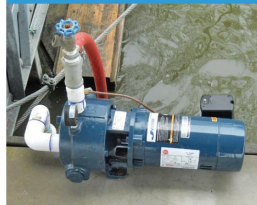
*All non-submersible pumps must be GFCI protected and must be properly bonded and grounded. Submersible pumps are no longer allowed at the Lake of the Ozarks.*
